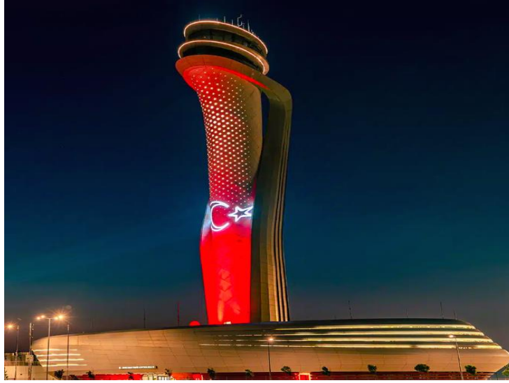
Figure 13 Istanbul Airport's Tulip-Shaped Control Tower 12
