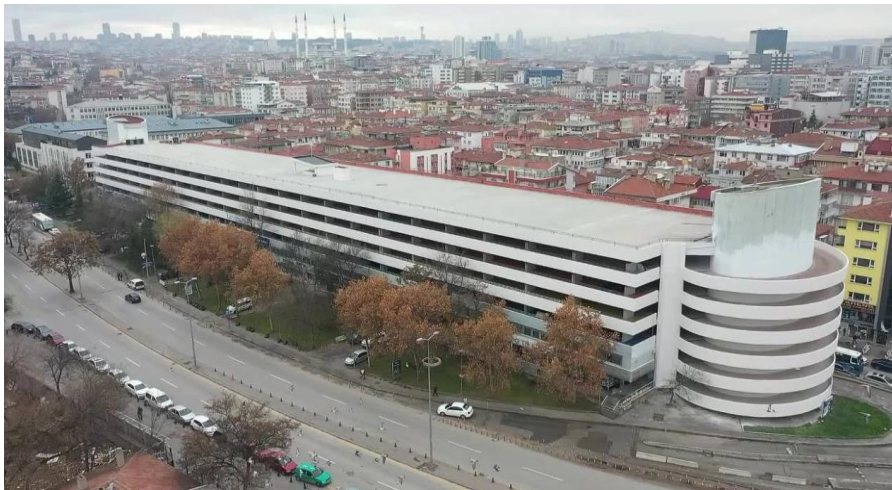
Figure 3.4 Sıhhiye Multistorey Car Parking Building. ( umke.org )
