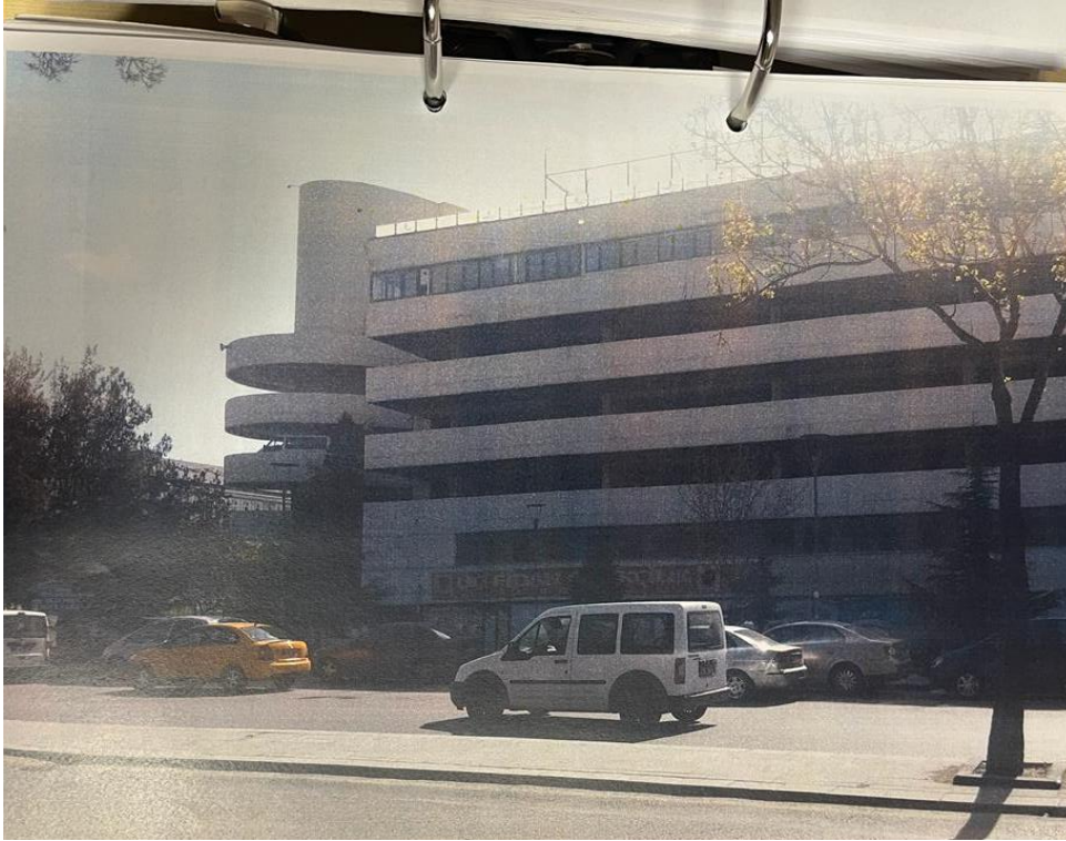
Figure B.1 Sıhhiye Multistorey Car Parking Building from Ankara Metropolitan Municipality archives.
