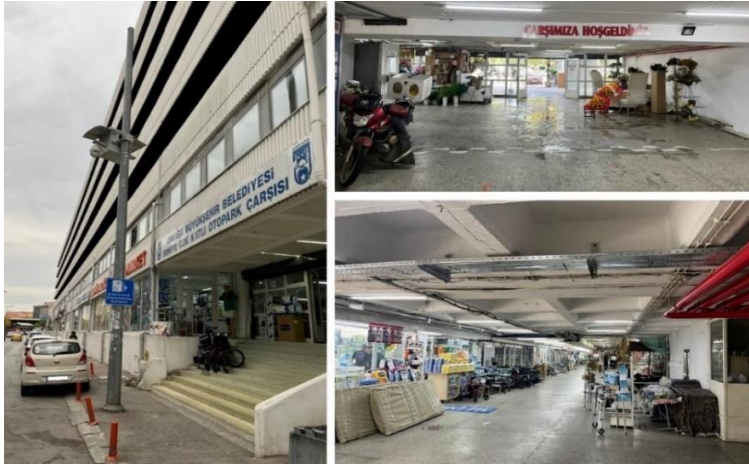
Figure 3.13 Ground floor bazaar of Sıhhiye Multistorey Car Parking Building.
