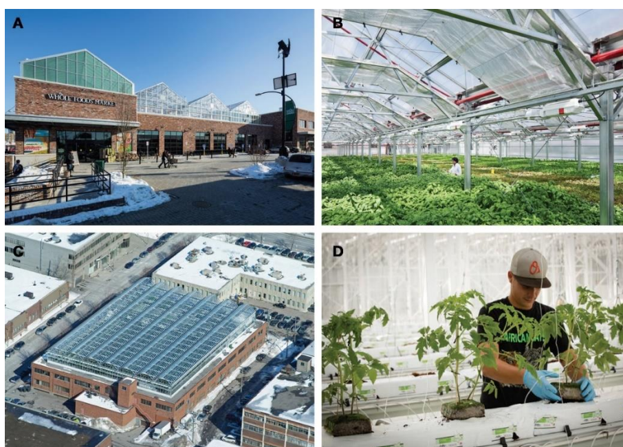
Figure 2.7 A. B. Rooftop greenhouse of Gotham Greens on Whole Foods supermarket in Brooklyn, C. D. Rooftop greenhouse of Lufa Farms in Montreal. (Proksch, 2017)
