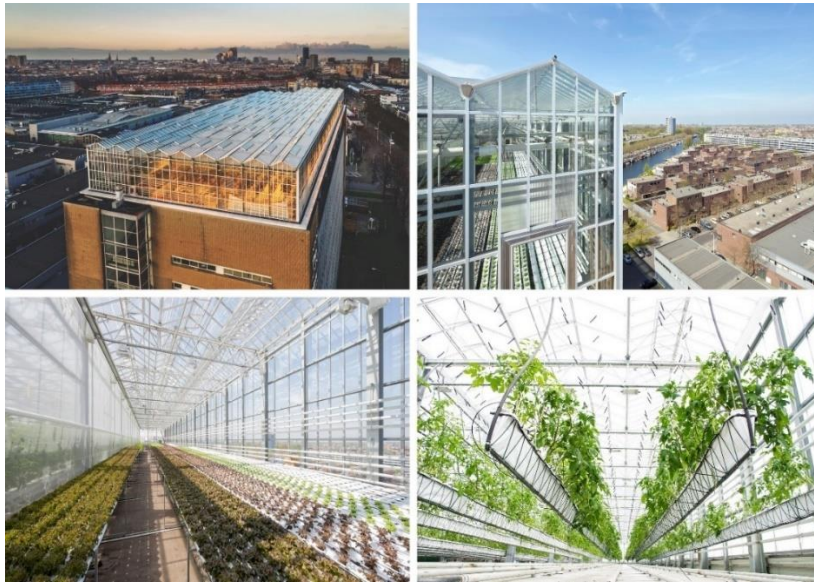
Figure 2.18 Vacant factory roof transformation by Urban Farmers rooftop greenhouse in the Netherlands. (spaceandmatter.nl)
