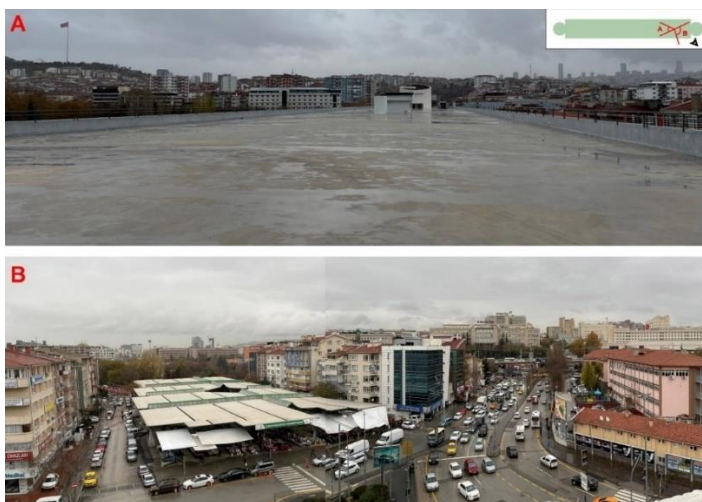
Figure 3.12 Rooftop and rooftop view of the building.
