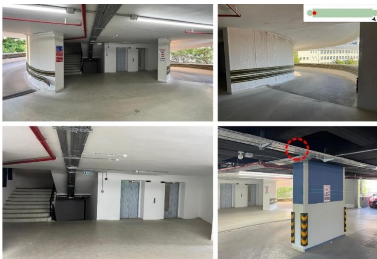
Figure 3.27 Helical vehicle ramps, entrance circulation core with staircases and elevator shafts, and data logging location for 3rd, 4th, and 5th data logging sessions. (10.01.2024-22.01.2024; 03.03.2024-18.03.2024; 24.04.2024-06.05.2024)
