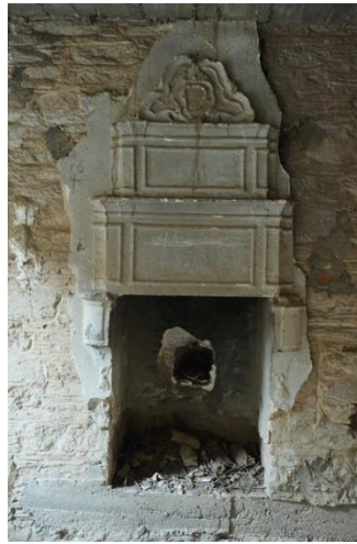
Figure 41. Koçarlı Cihanzade Tower's Fireplace (Photographed by the author)
