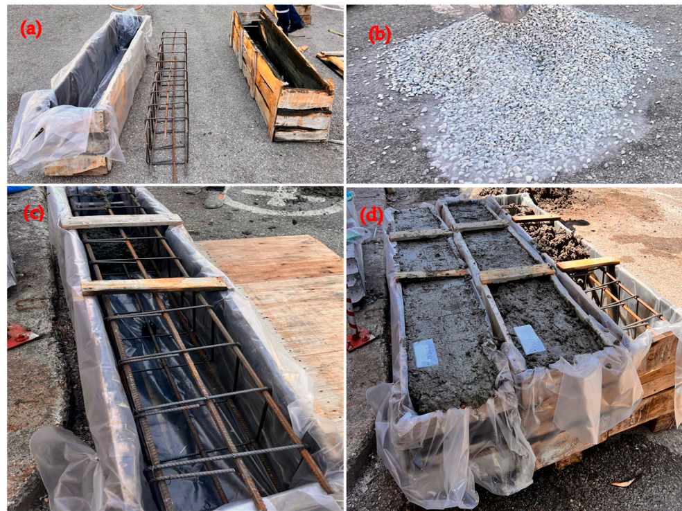
Figure 3. Preparation of RCBs, (a) preparation of molds, (b) materials, (c) reinforcement in the RCB, (d) setting up concrete.
