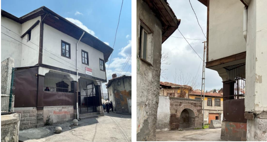
Figure 3.46. Northern facade of the Eskiciođlu Mosque (left), Eskiciođlu Fountain (right) (Author, 2024)
