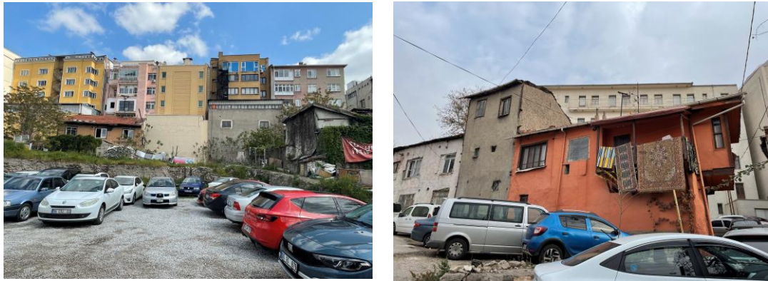
Figure 3.39. Unplanned areas and streets using as parking areas (Author, 2023)
