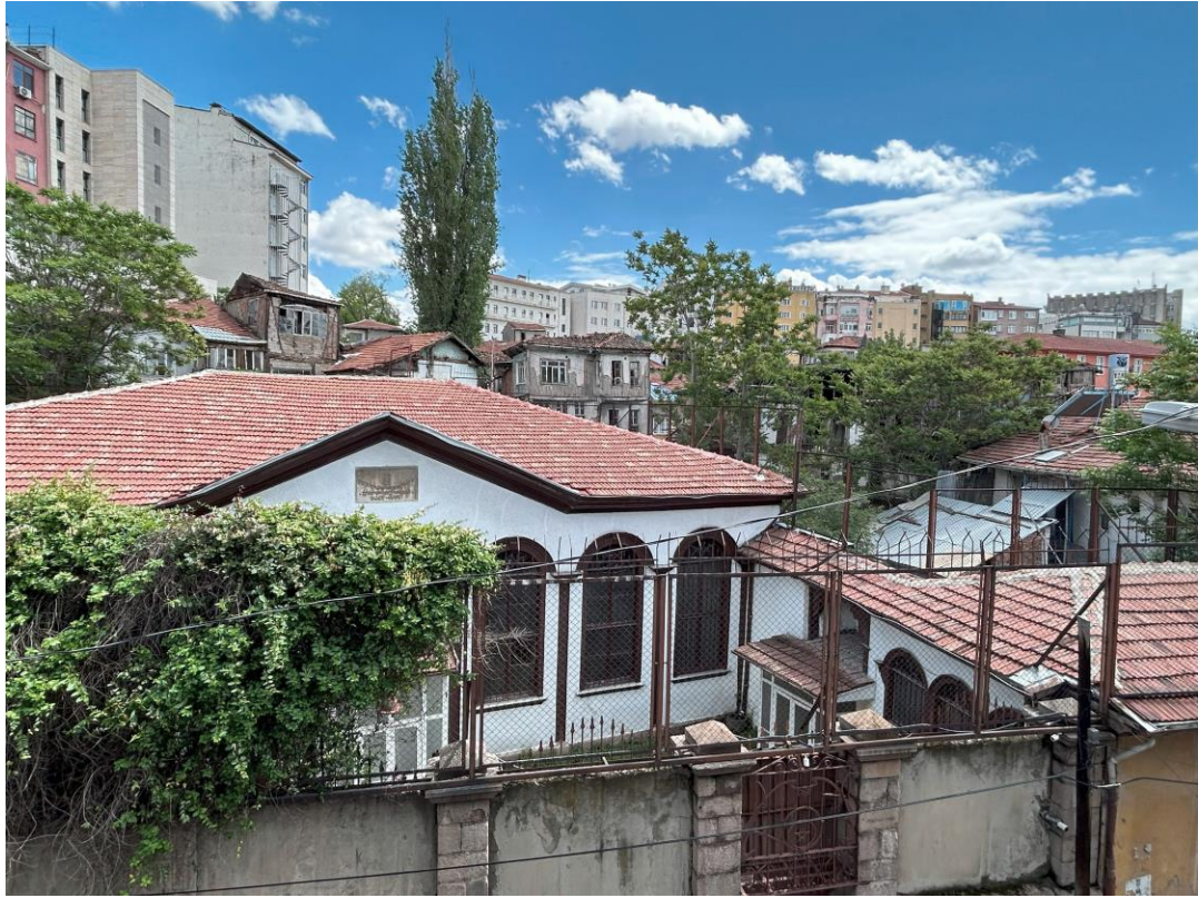
Figure 3.62. Ankara Synagogue, Courtyard and Walls (Author, 2024)
