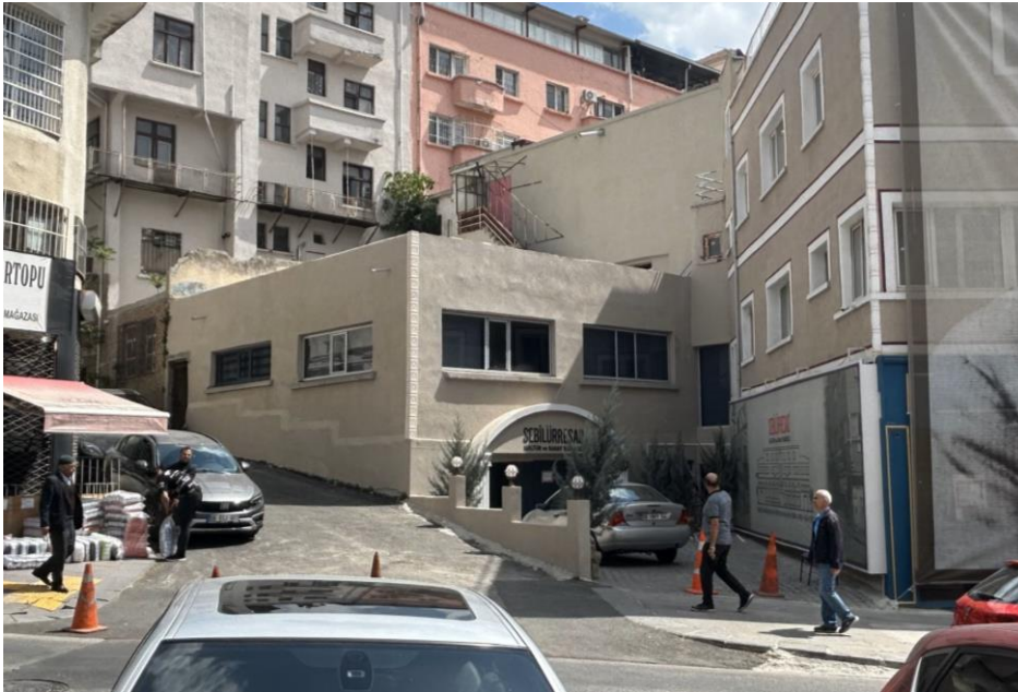
Figure 3.80. Sümer Cinema Building after Restoration (Author, 2024)
