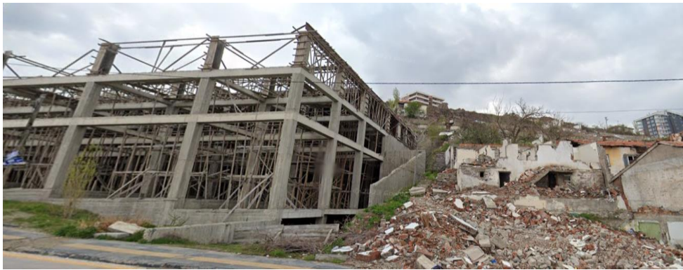
Figure 4.14. Doğantepe neighborhood abandoned areas (obtained from Google Earth Street view, date: 23.07.2024)
