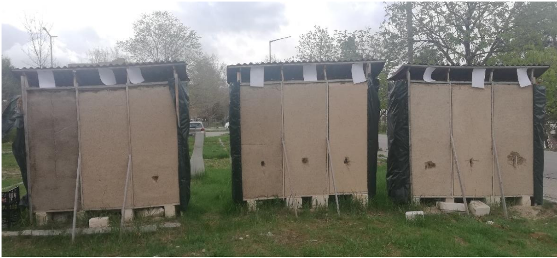
Figure 3-1. Strawbale walls marked A, B and C Panels (ordered left to right).
