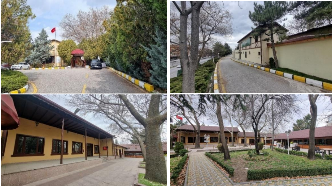
Figure 3. 11: Club building, currently used as Altın Koru Wedding Hall. Spot 1 in Kural’s sketch (left up), Spot 2 (right up), Spot 3 (left down), Spot 4 (right down).
