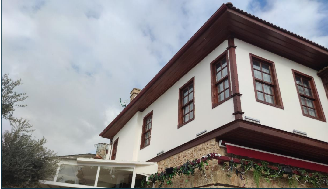
Figure 3.71. Extensively repaired timber exterior wall. Taken by the Author.
