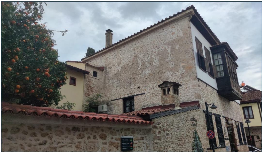
Figure 3.37. Photograph of service wall of Building C. Taken by the Author.
