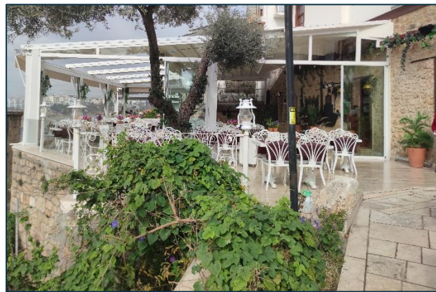
Figure 3.58. Building A leveled and tiled flooring in direct relation with the street. Taken by the Author.
