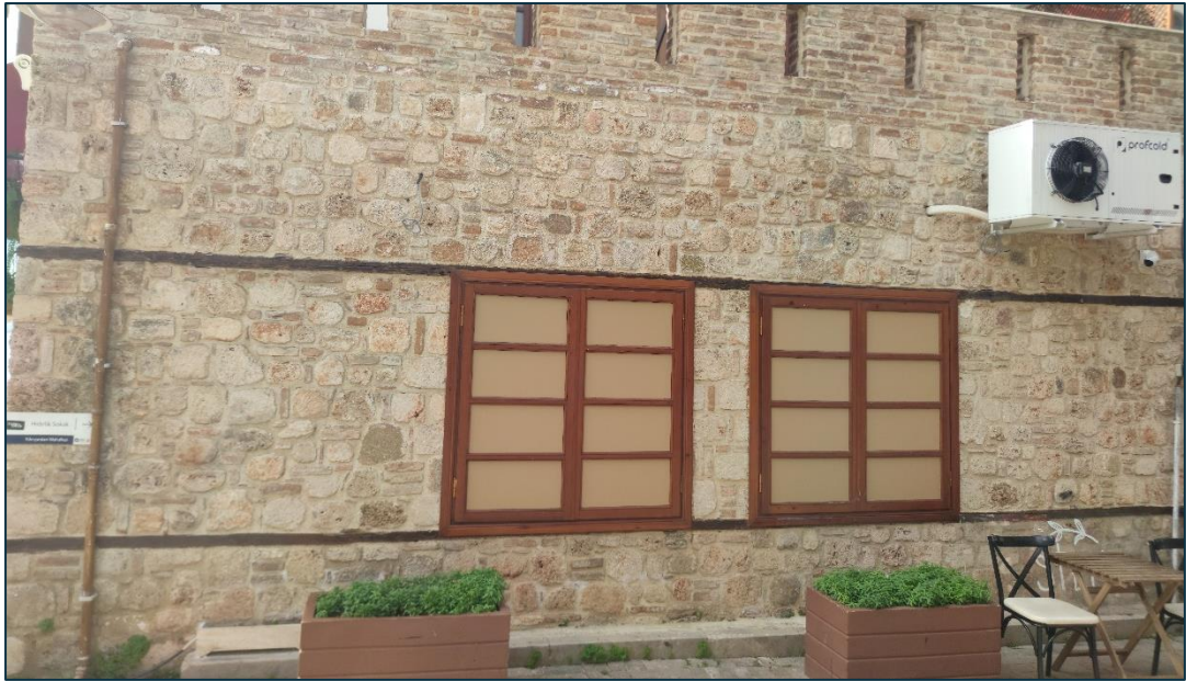
Figure 3.70. Partially reconstructed masonry wall. Taken by the Author.
