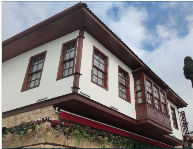
Figure 3.84. Timber windows replacement using the original techniques. Taken by the Author.
