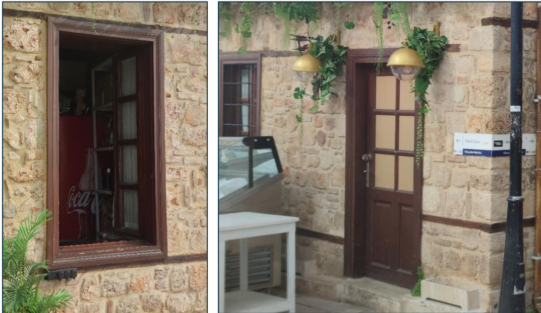
Figure 3.75. Timber window replacing an original one using unoriginal materials and techniques. Taken by the Author. Figure 3.76. Secondary door replacement using unoriginal materials and techniques. Taken by the Author.
