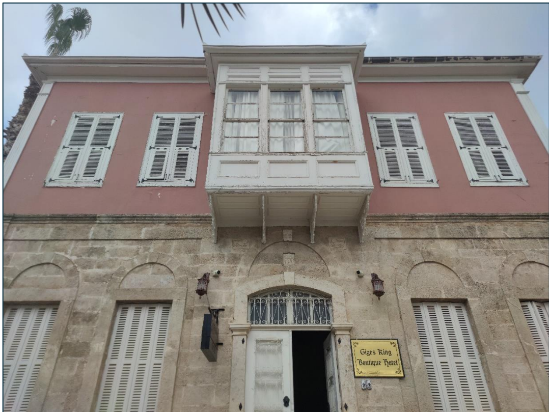
Figure 3.89. Building B entrance elevation. Taken by the Author.
