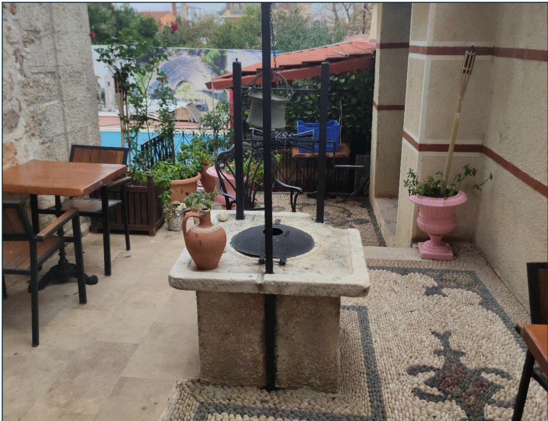
Figure 3.34. Photograph of the cistern within the courtyard of Building B. Taken by the Author.
