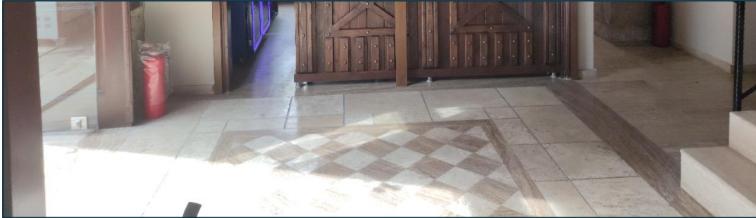
Figure 3.65. Added interior floor tiles. Taken by the Author.
