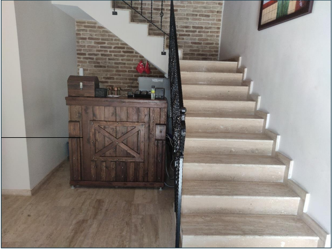
Figure 3.72. Added concrete stairs. Taken by the Author.
