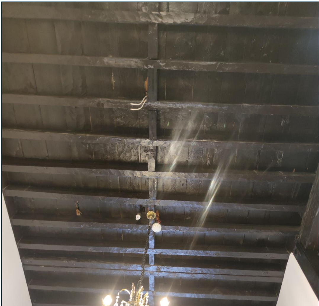
Figure 3.96. Ceiling structure and planks in Building C. Taken by the Author.
