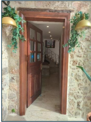
Figure 3.82. Added architectural elements (door). Taken by the Author.
