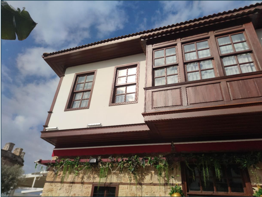
Figure 3.87. Façade additions. Taken by the Author.
