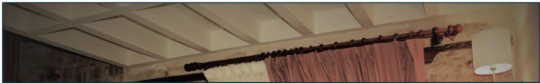
Figure 3.101. Floor planks of the timber addition in Building D. Retrieved on 2/02/2024 from http://palmhouse17.com/
