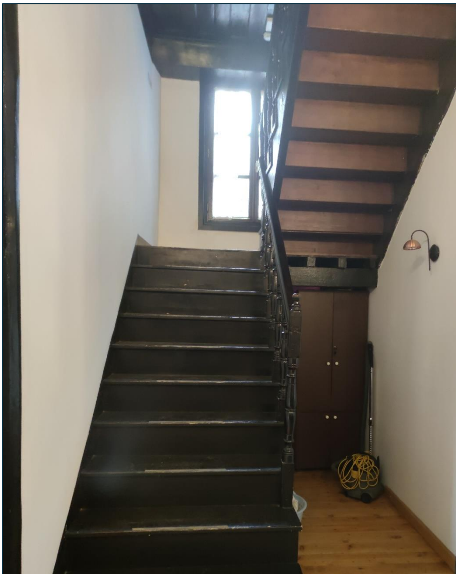
Figure 3.97. Timber stair in Building C. Taken by the Author.
