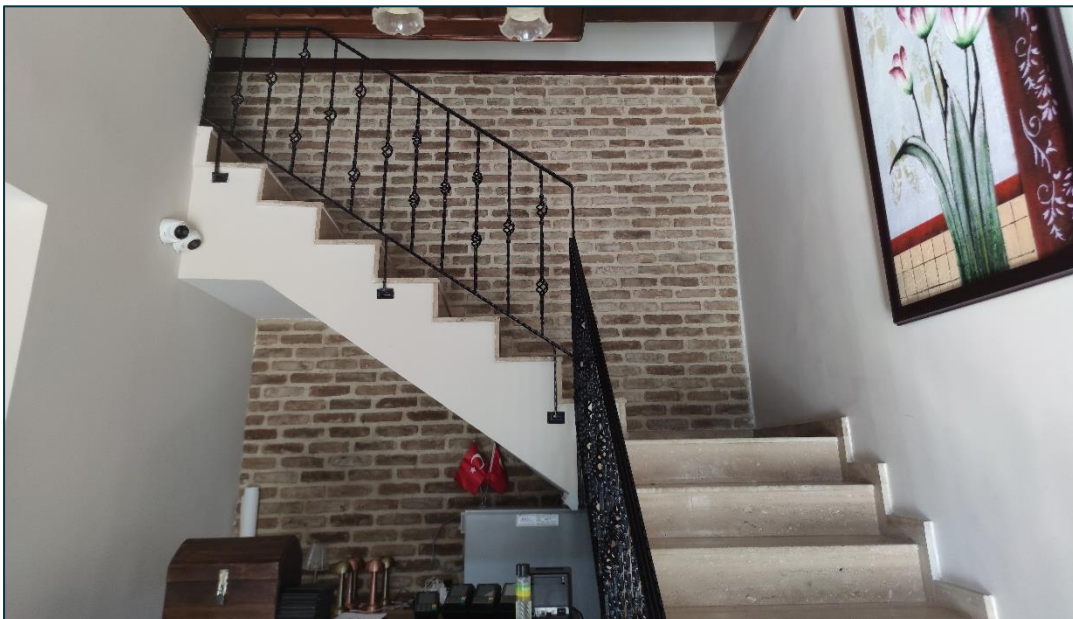
Figure 3.66. New brick wall replacing the original stone masonry one. Taken by the Author.
