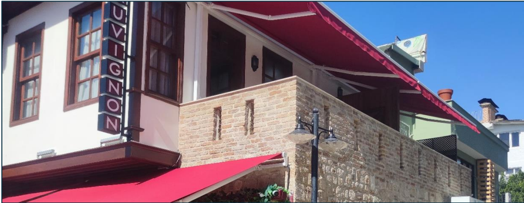
Figure 3.64. Added porch on top of the shop area. Taken by the Author.
