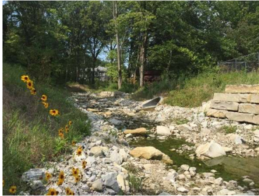
Figure 2.1 Dry Detention Basin (HR Green, n.d.)
