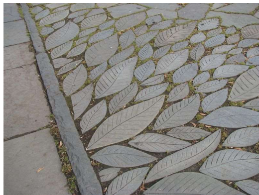
Figure 2.10: Concrete leaf walkway (Whiteley Creek Homestead)
