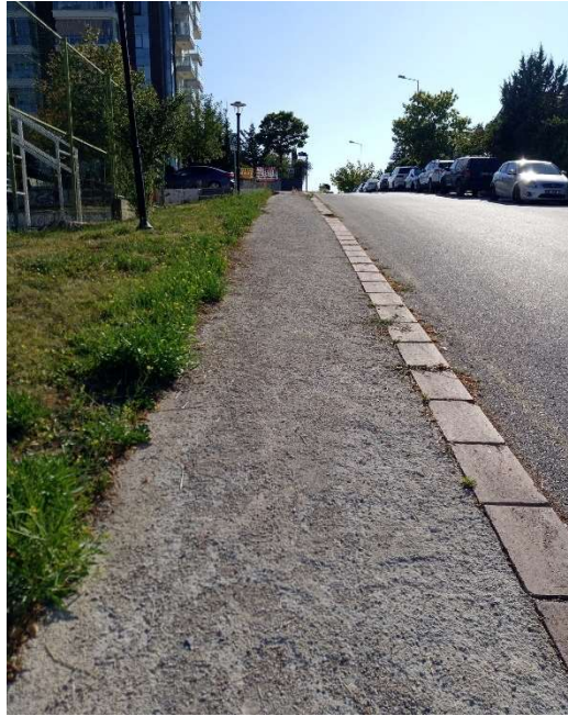
Figure 4.12: Unfinished sidewalk near Area 4
