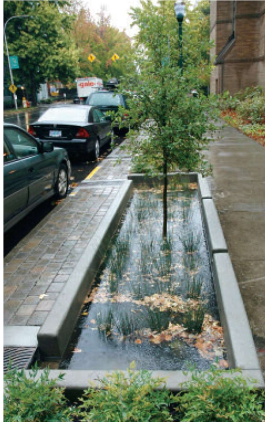
Figure 2.5 Stormwater planter temporarily filled with rainwater after a storm (Dunnett & Clayden, 2007)
