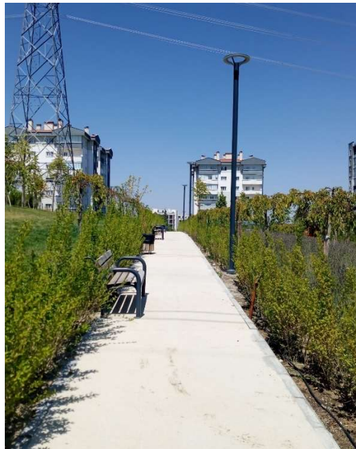
Figure 4.9: Concrete pathway in Area 7
