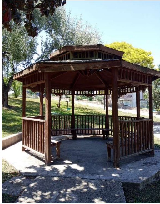
Figure 4.6: Wooden gazebo on top of concrete path in Area 4
