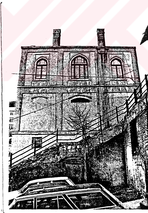
Photo.65 SE facade - the Inspection Committee building (1987)
