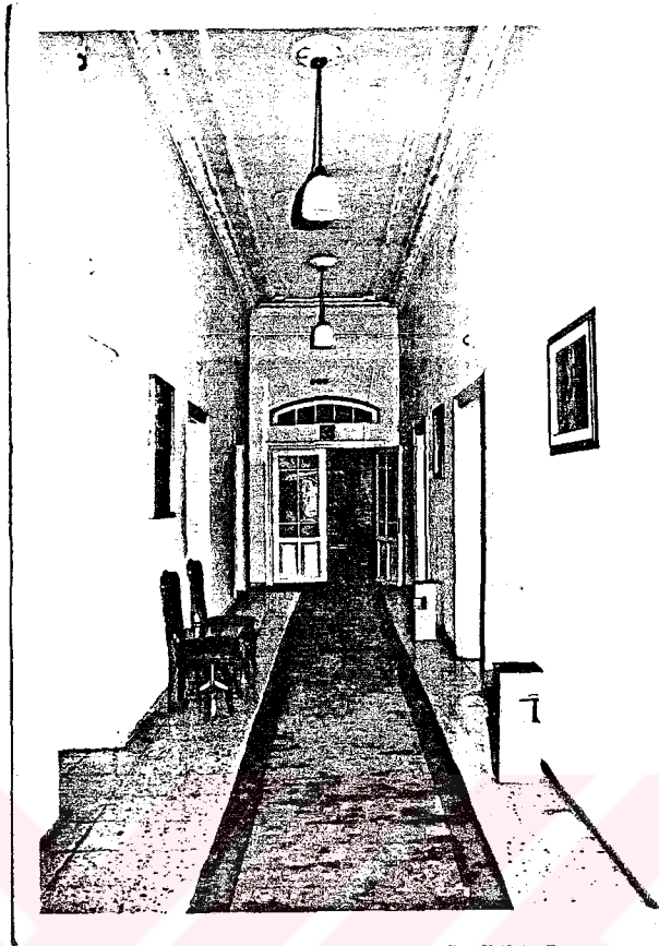
Photo.28 The Central building - upper floor - NW corridor (1987)
