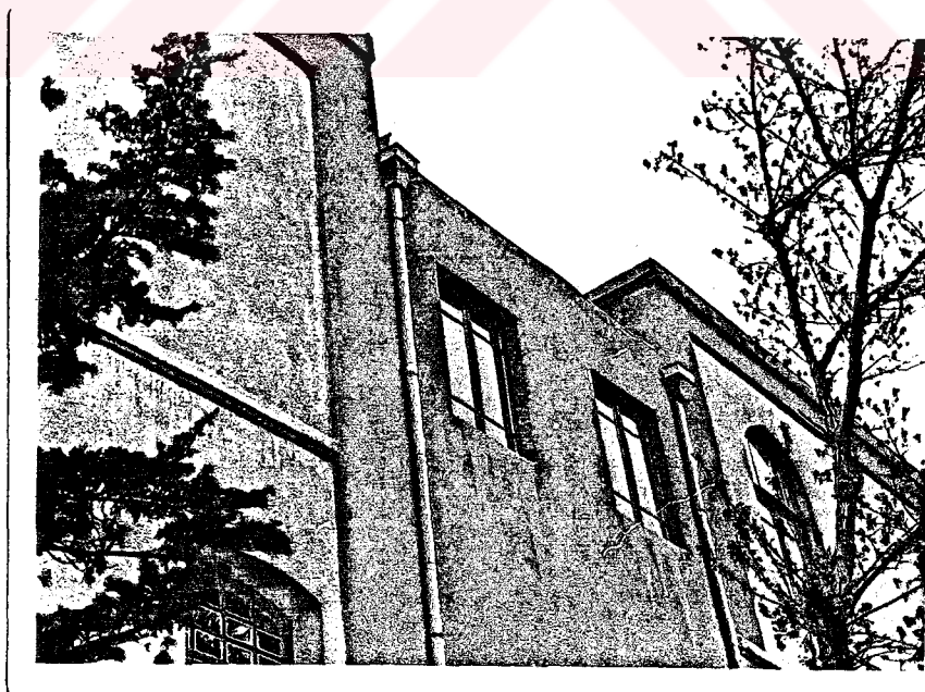
Photo.69 SW facade - SE wing (1987)
