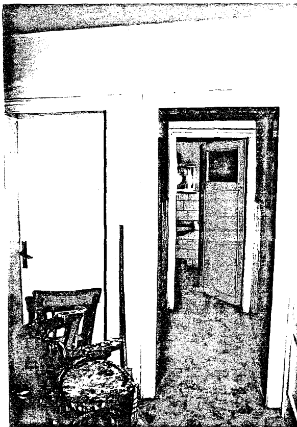
Photo.119 The basement floor - toilets - (1987)
