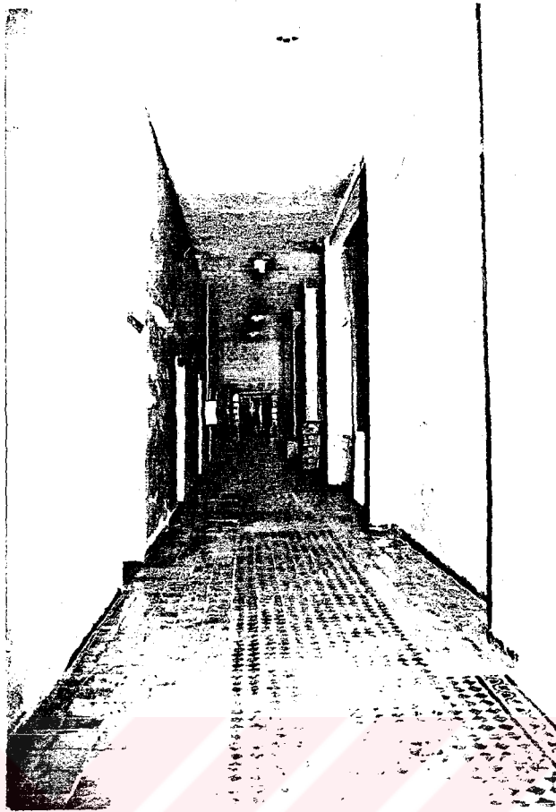
Photo.168 Ground floor - SE corridor (1987)
