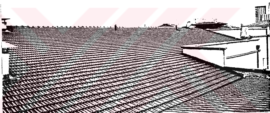
Photo.280 Raised roof (skylight was left under the roof) (1988)
