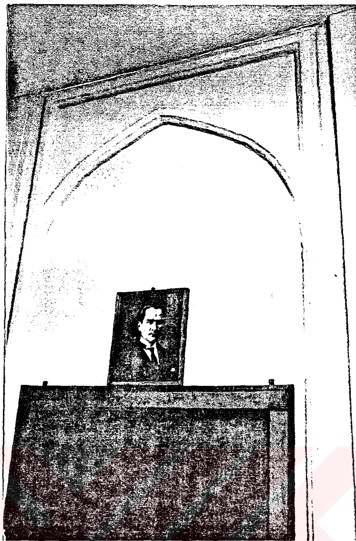
Photo.56 SE wing - upper floor - NW wall of the room on the NE (1987)
