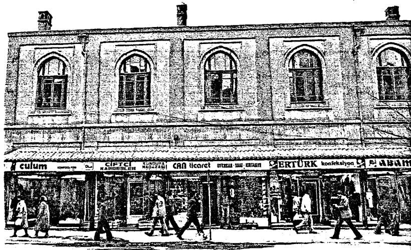
Photo.64 NE facade - the Inspection Committee building (1987)
