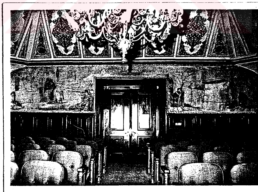
Photo.31 The Central building - upper floor - SE wall of the meeting hall (1987)
