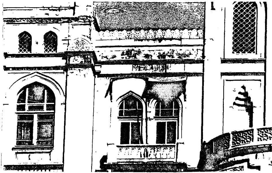
Photo.270 NW facade - broken shelters on the upper balcony (1976)
