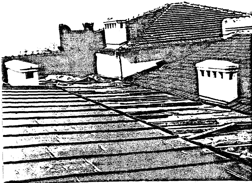
Photo.277 Copper and Marseilles-type tiles of the roof (1986)
