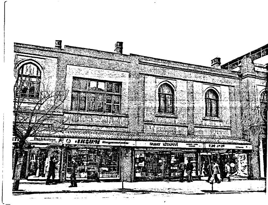
Photo.62 NE facade - the Central building - (SE side portion) - SE wing (1987)
