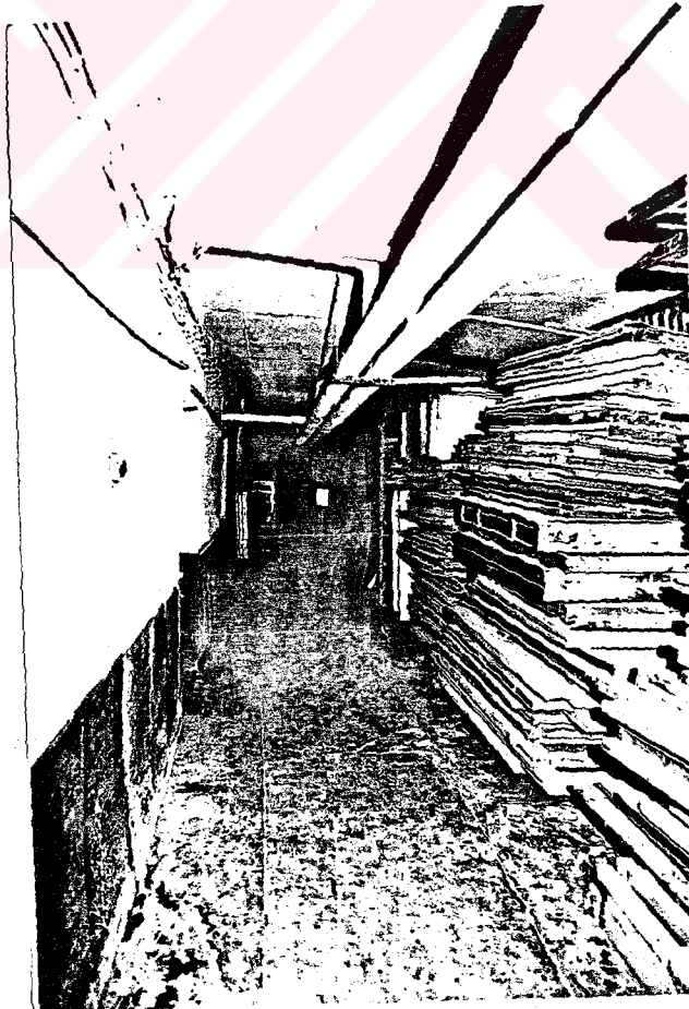
Photo.181 Basement floor - NW corridor - central part (1987)
