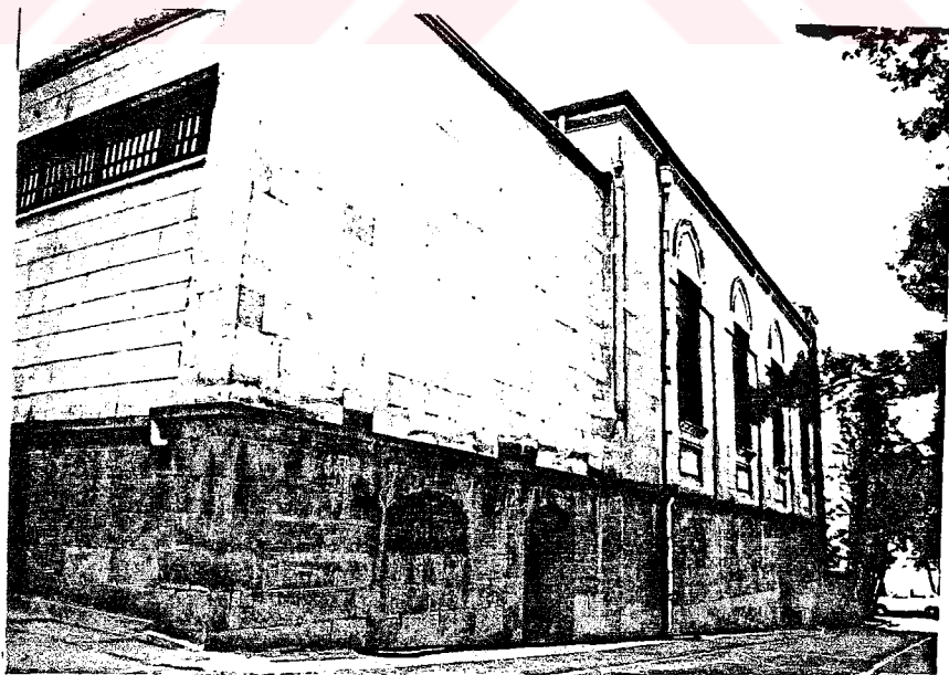
Photo.130 NE facade - SE portion (1987)
