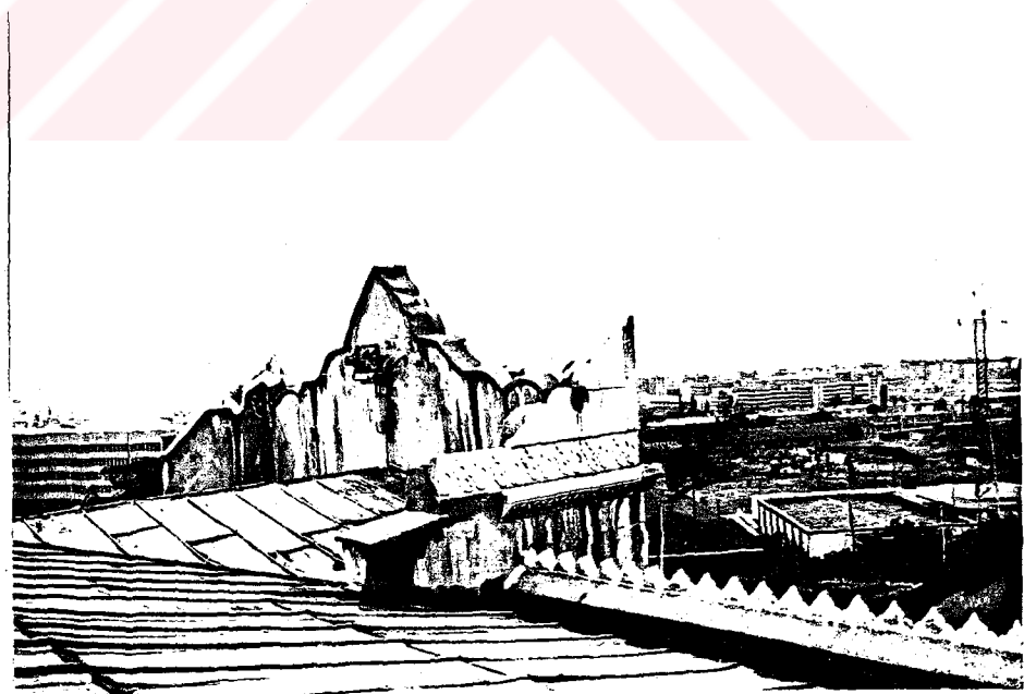
Photo.155 Roof of the SW portion (1987)
