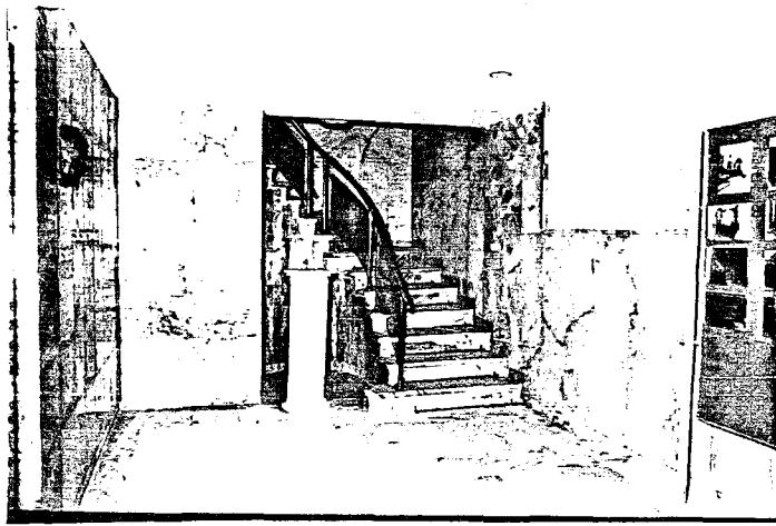
Photo.234 Basement floor - Sedat Simavi gallery (1987)
