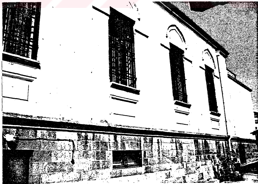
Photo.137 SW facade - SE portion (1987)
