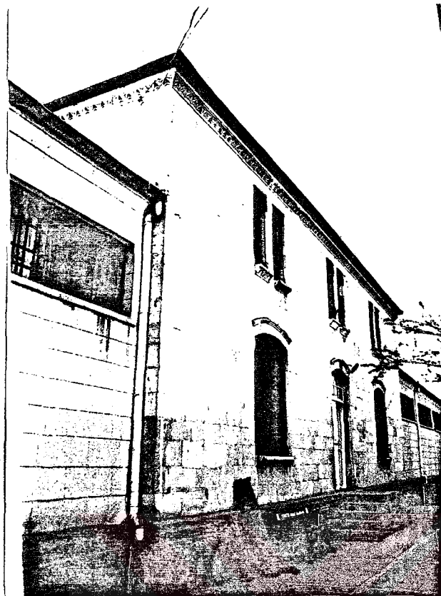
Photo.133 SE facade - central portion (1987)
