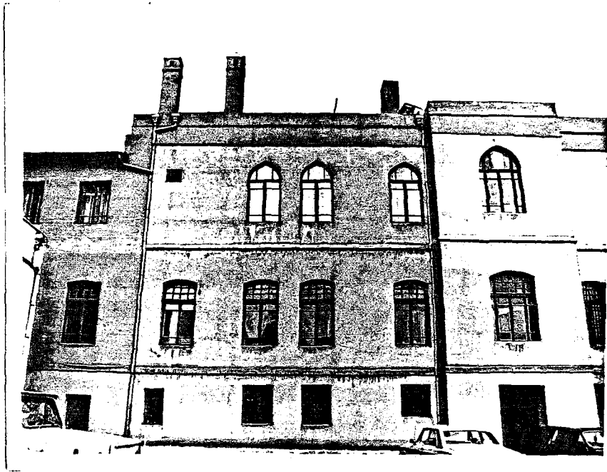
Photo.66 SW facade - the Central building - (central and NW portion) (1987)
