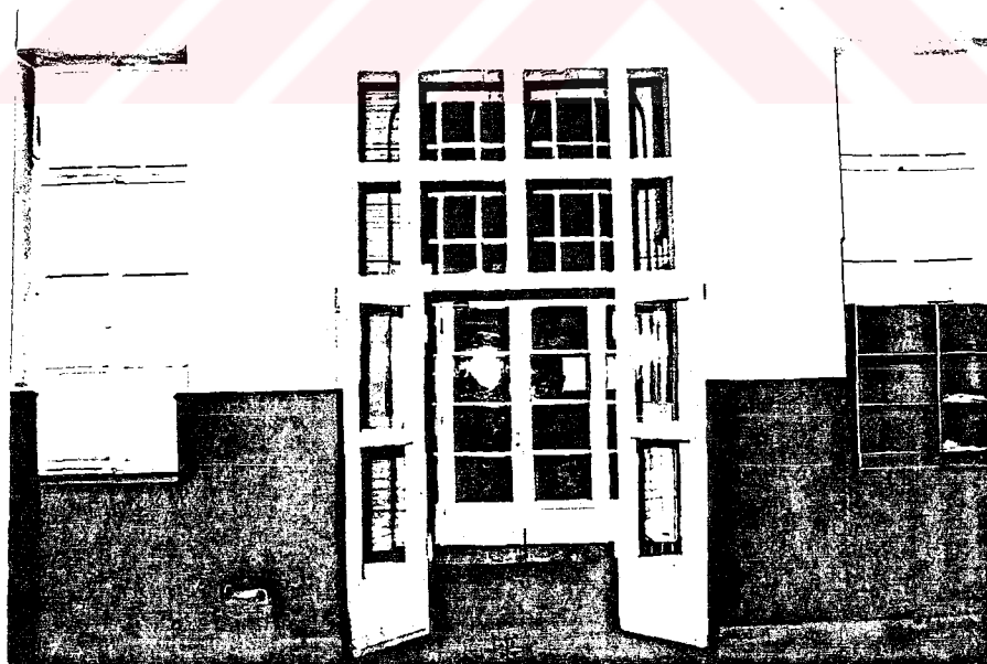
Photo.167 Ground floor - covered entrance in the NE corridor (1987)
