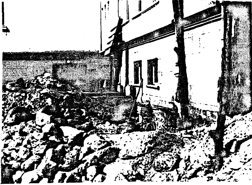
Photo.282 Türk Ocağı Building - isolation of the foundations (1977-1985 restoration)
