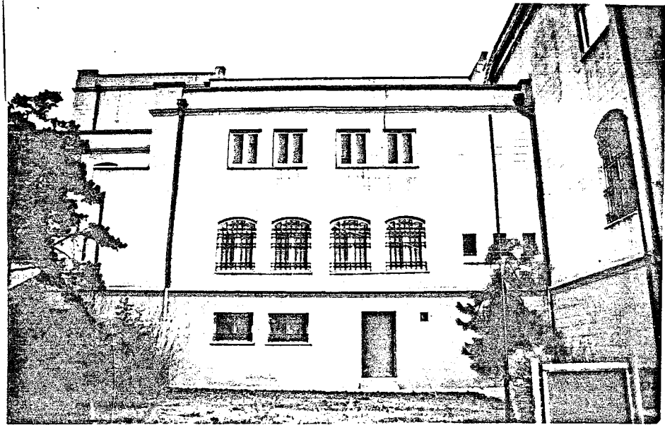
Photo.246 NE facade - third portion (1987)
