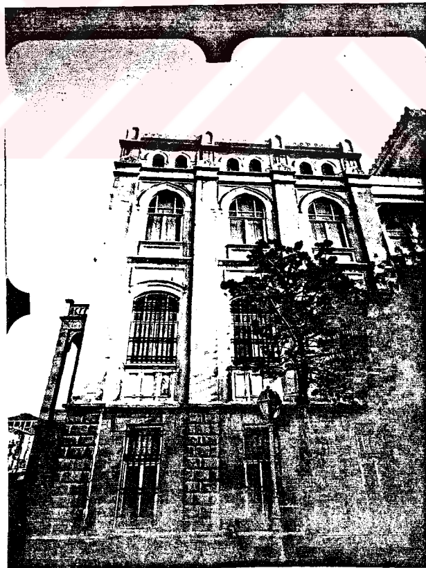
Photo.243 NW facade - NE side portion (1986)
