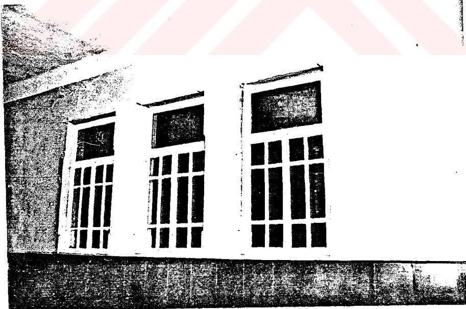
Photo.173 Windows of the stairwell (NE) (1987)
