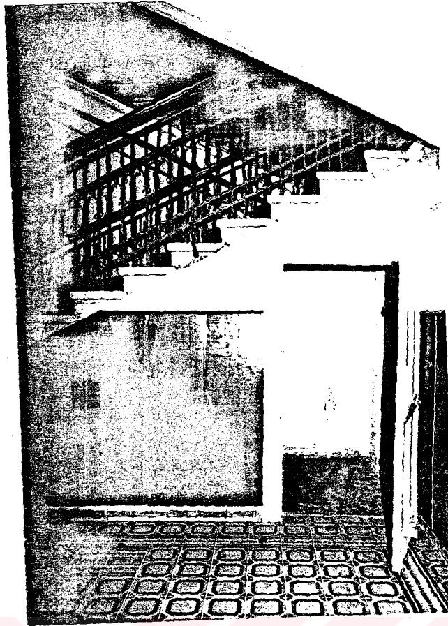
Photo.180 Ground floor - door leading to the basement floor staircase (1987)
