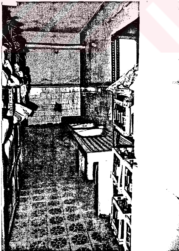
Photo.41 The Central building - basement floor - storage room on the NE of the SE corridor (1987)
