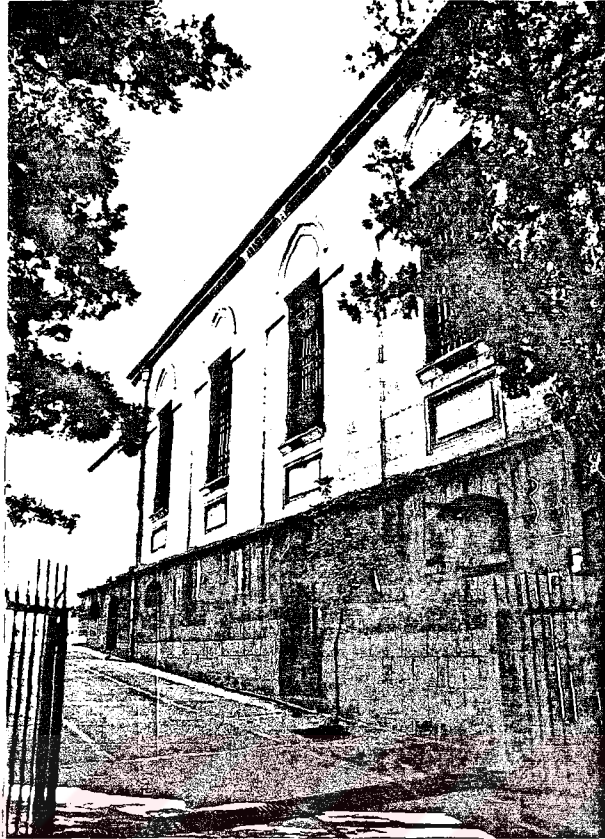
Photo.129 NE facade - NW portion (1987)
