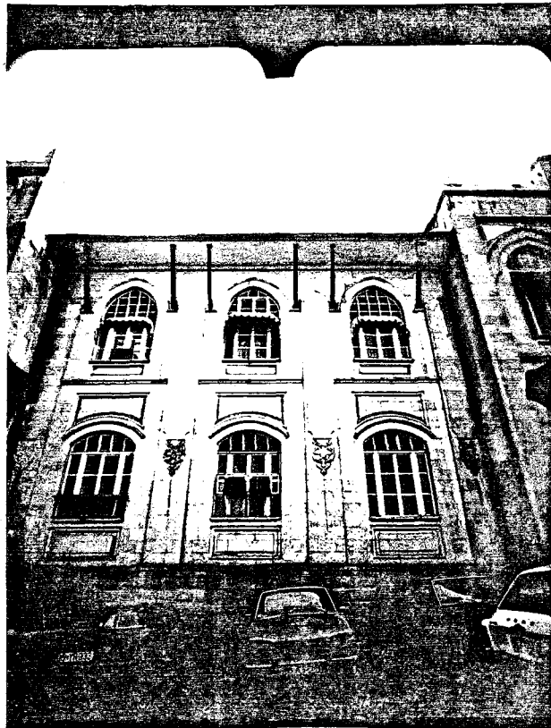
Photo.188 NW facade - SW of the central portion (1986)
