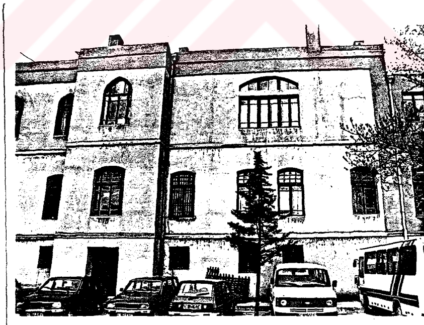
Photo.67 SW facade - the Central building - (central and SE portion) (1987)
