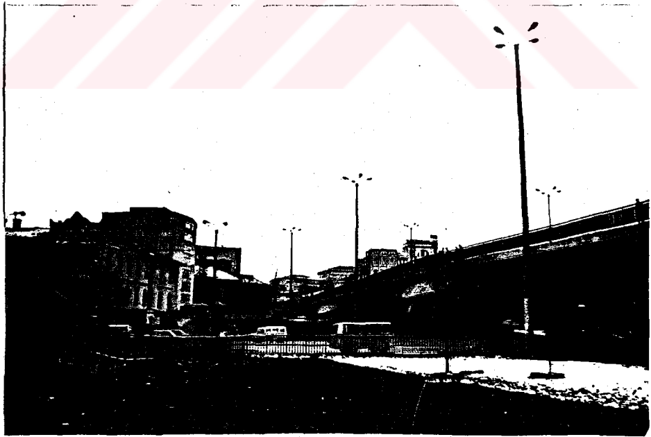
Photo.161 Talat Pađa Boulevard (SW) (1987)
