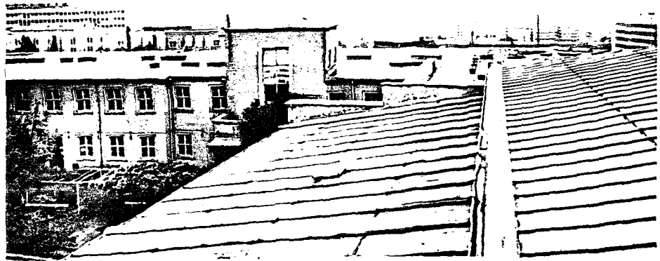
Photo.154 Roof of the second gallery (SW) (1987)
