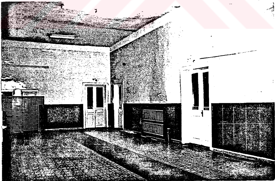
Photo.179 Upper floor - SE of the SW corridor (1987)
