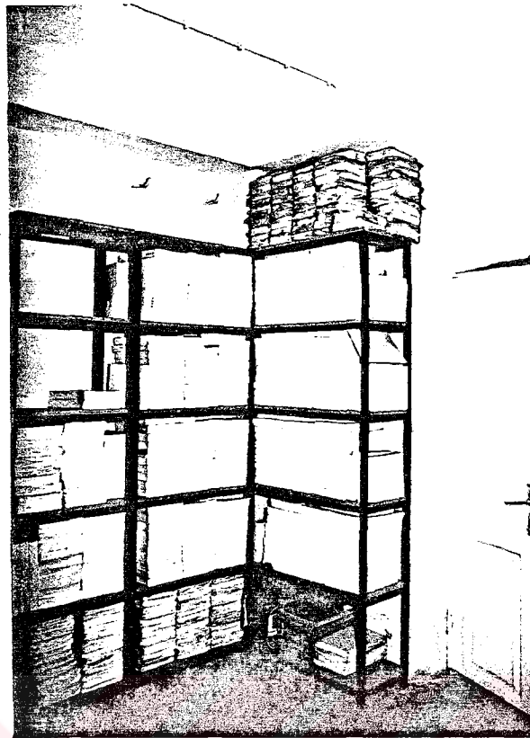
Photo.48 The Central building - SE wing (1987)
