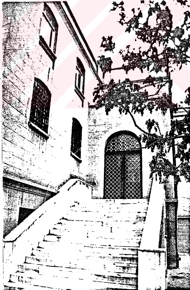
Photo.247 NE facade - fourth and fifth portions (1987)
