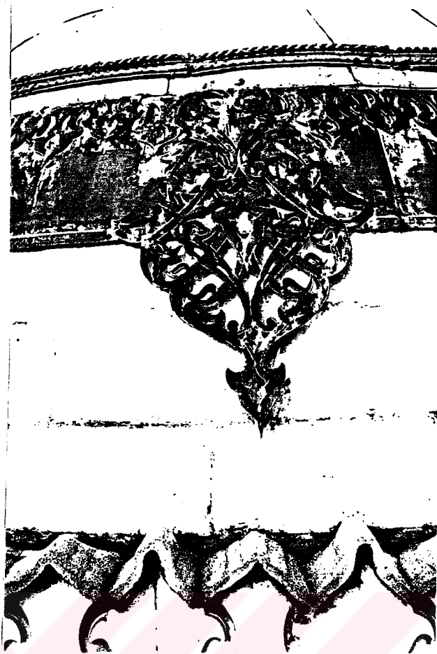
Photo.152 A detail from the dome (1987)
