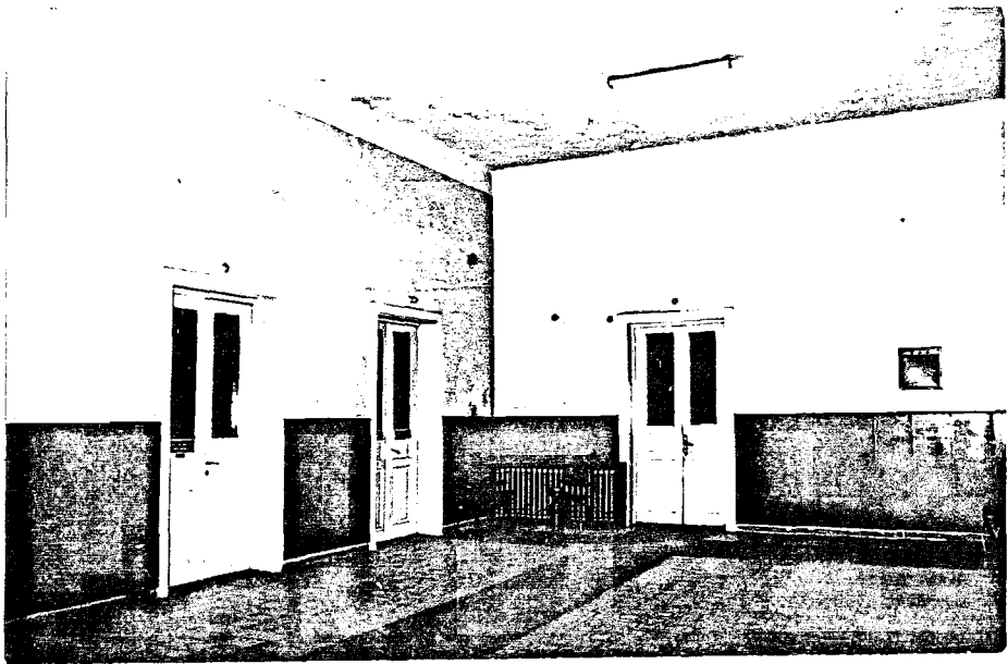
Photo.178 Upper floor - NW of the SW corridor (1987)
