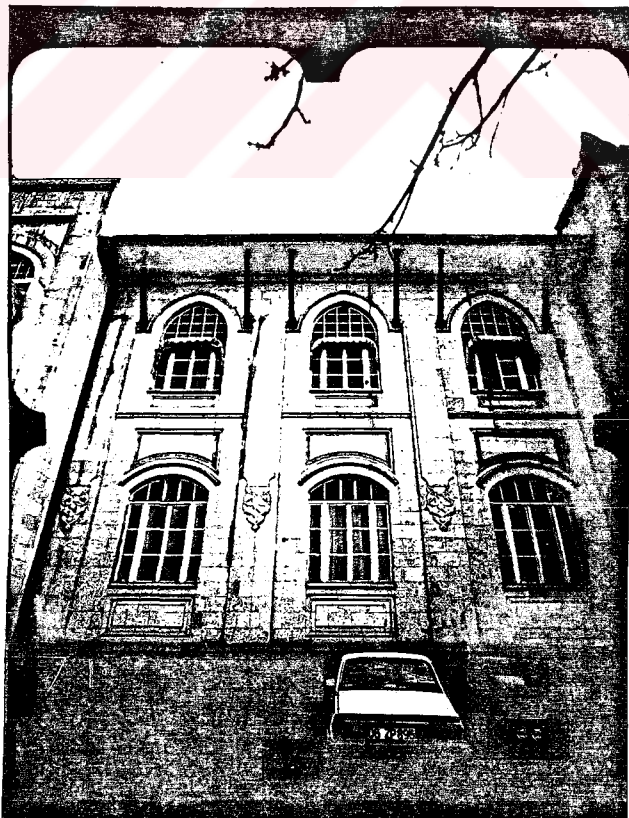
Photo.187 NW facade - NE of the central portion (1986)
