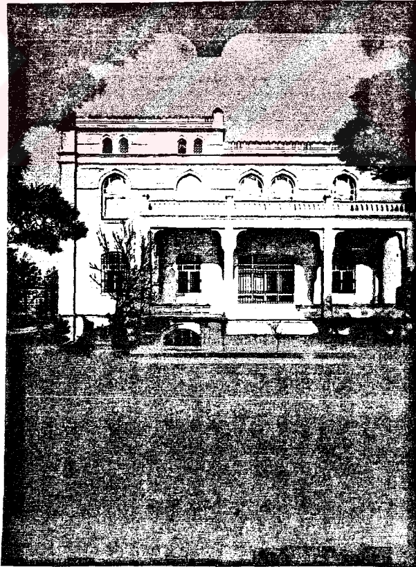
Photo.252 SW facade - first portion (1986)
