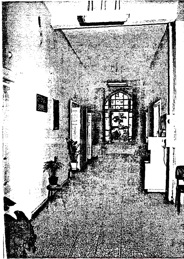
Photo.52 The Inspection Committee building - upper floor - corridor extending in the SE-NW direction (1987)
