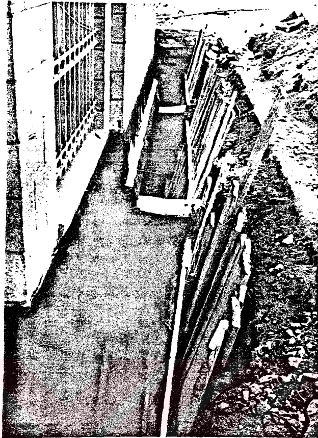
Photo.284 Türk Ocağı Building - isolation of the foundations (1977-1985 restoration)
