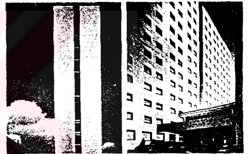
Figure 81a-b. a. Palm Olive office building, Milan (L.Moretti); b. Casa Albergo, Milan (L.Moretti and E.Rossi) (RIBA, October 1958)
