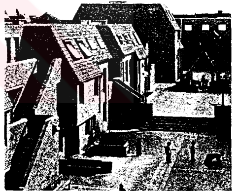
Figure 149a-c. Restructuring of the Alma-Gare quarter, Roubaix (M.Benoit, et.al.); buildings face a court as external extension like the previous tissue; result of twenty years' urban protest against demolishing and rehabilitation (Casabella, January/February 1983)
