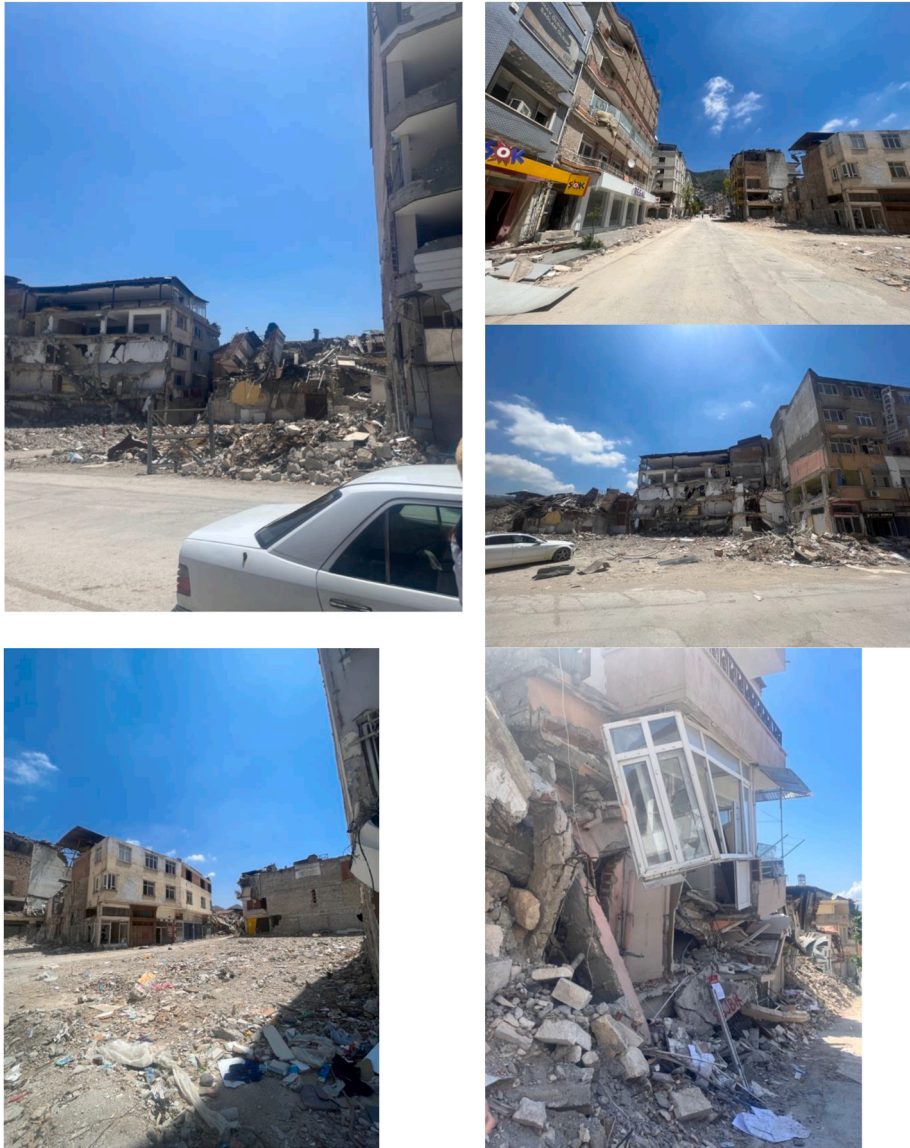
Fig. A.2. Antakya city center on June 5th 2023.
