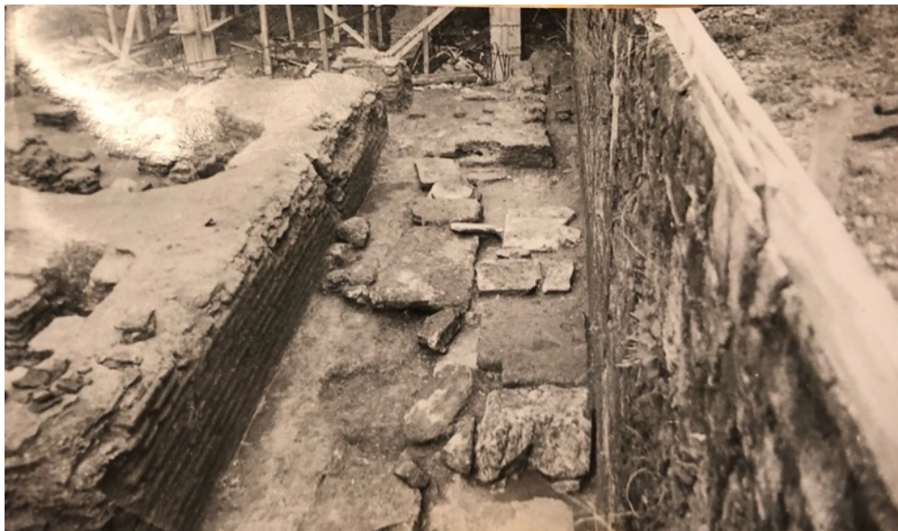
Figure 120. The Photos of Roman street found during the construction of Additional Building (source: The Personal Achieve of Nezhir Firatlı, IAM Archive)
