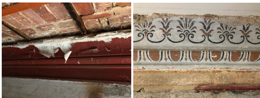
Figure 236. The photographs taken during the removal of painting layer from the cornice decorations (source: taken by the author in 2018)
