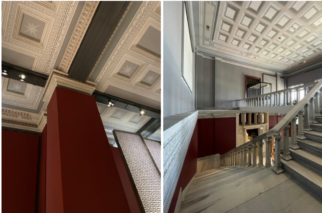
Figure 151. (Left) The decorative ceiling Hall no: 8 after restoration, (Right) The decorative ceiling of Hall No: 30 after restoration (taken by the author in 2024)
