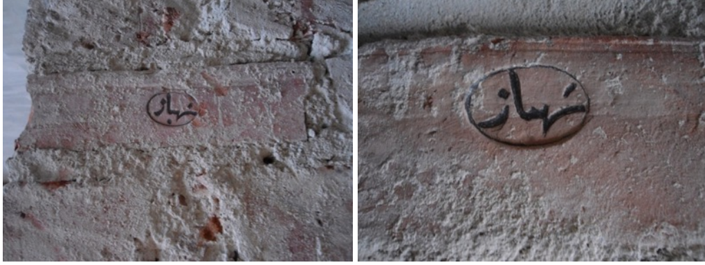
Figure 153. The şahbaz brand machine made bricks found in IAM building (source: Güryapı İnşaat Company, IDSM Archive)
