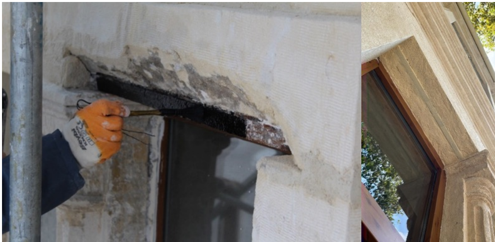
Figure 34. The historical Yeniköy Military Service Building, façade details (source: IDSM Archive)
