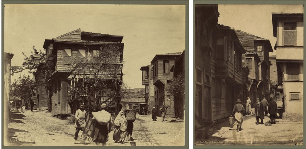
Figure 38. The timber fabric in Istanbul streets source: Library of Congress)
