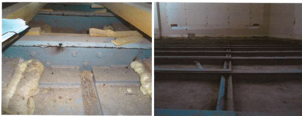
Figure 249. The Photographs of CC sections drawing of Hall 21 jack arched flooring details ( Güryapı İnşaat Construction site report, November 2012, IDSM Archive)
