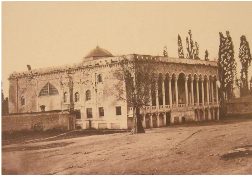
Figure 68. The photograph showing the condition of the Tiled Kiosk in 1863. (source: (Öztuncay, 2003 as cited in Restitution Report of Tiled Kiosk prepared by YD Mimarlık found in IDSM Archive)
