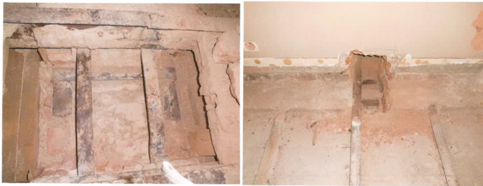
Figure 251. (Left) The Photograph of AA section drawing of Hall 22 jack arched flooring details (Right) The Photograph of BB section drawing of Hall 22 jack arched flooring details (Güryapı İnşaat Construction site report, November 2012, IDSMS Archive).
