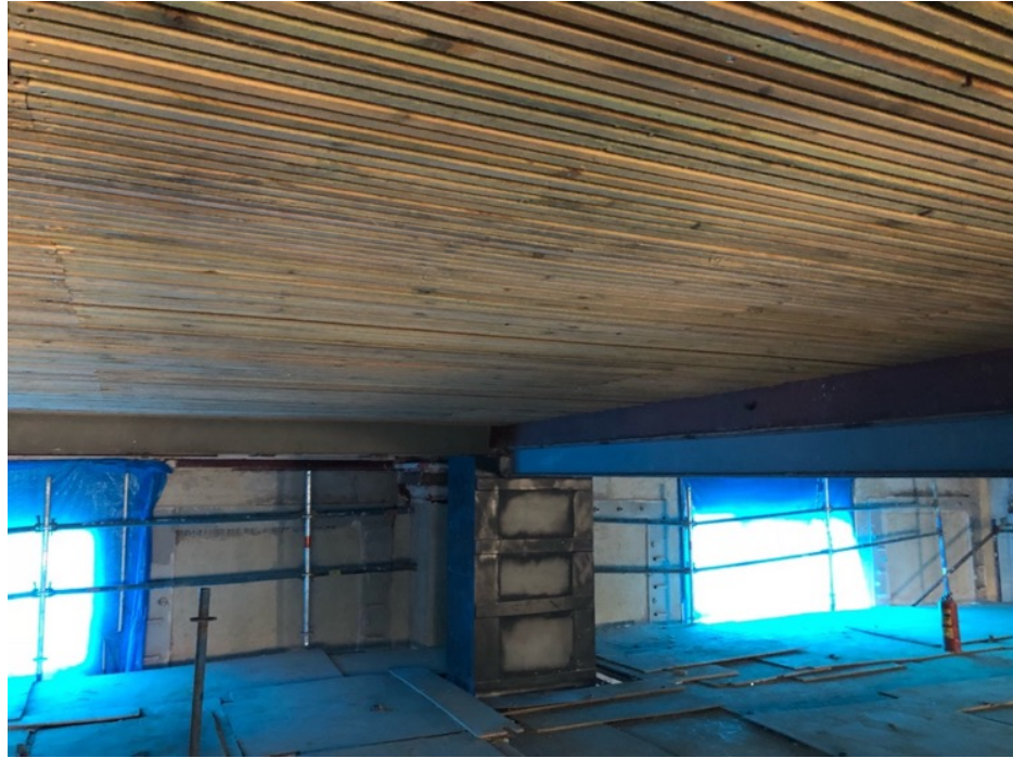
Figure 238. Bağdadi techniques under the Jack arched flooring (taken by the author in 2018)
