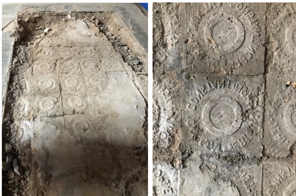
Figure 157. Cement tile “ karo mozaik ” traces written “ Constantinople Kalafat Yeri ” found under one of the sarcophagi in the Sarcophagus hall which was covered by marble later on (taken by the author in 2018)
