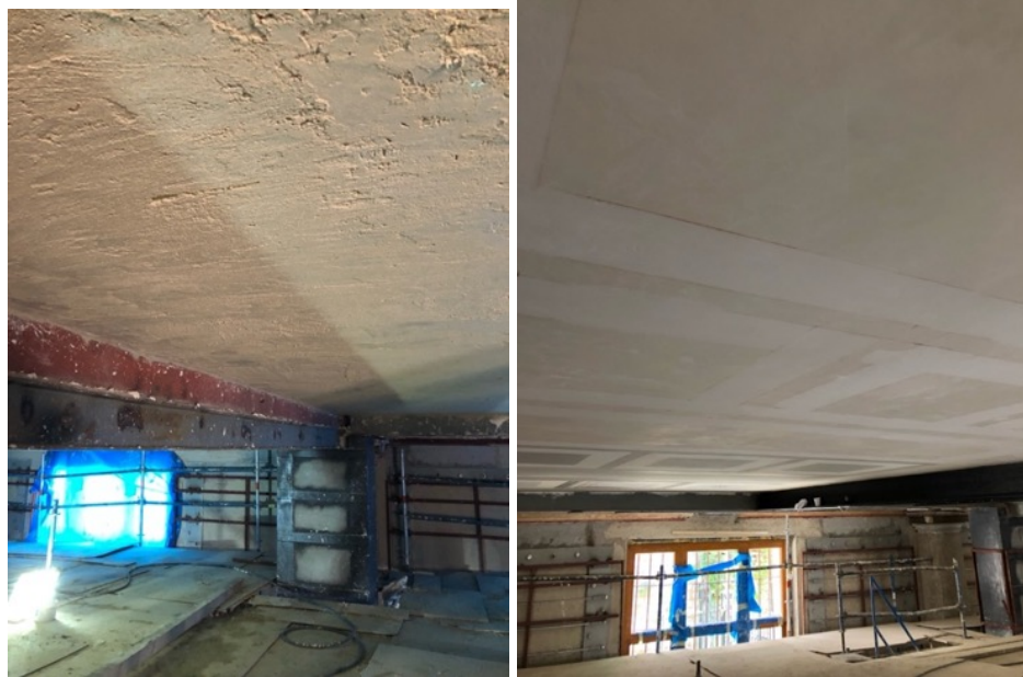
Figure 239. (Left) Plaster over the bağdadi techniques and (Right) nefaset fine plaster over it (taken by the author in 2018)
