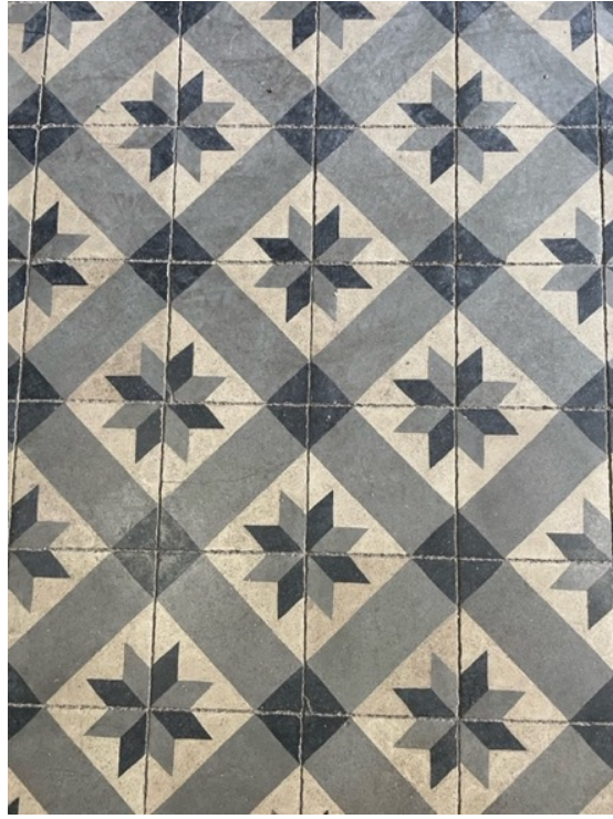
Figure 158. The Cement tiles “ karo mozaik ” in the 2 nd phase of IAM (taken by the author in 2024)
