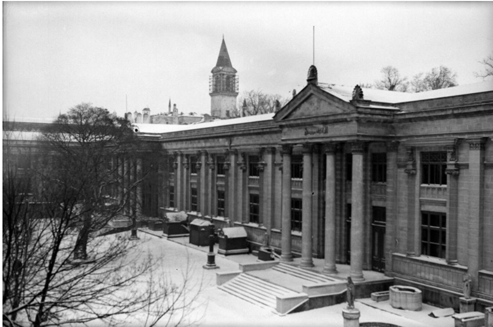
Figure 131. IAM Building (source: IAM-Photography Archive)
