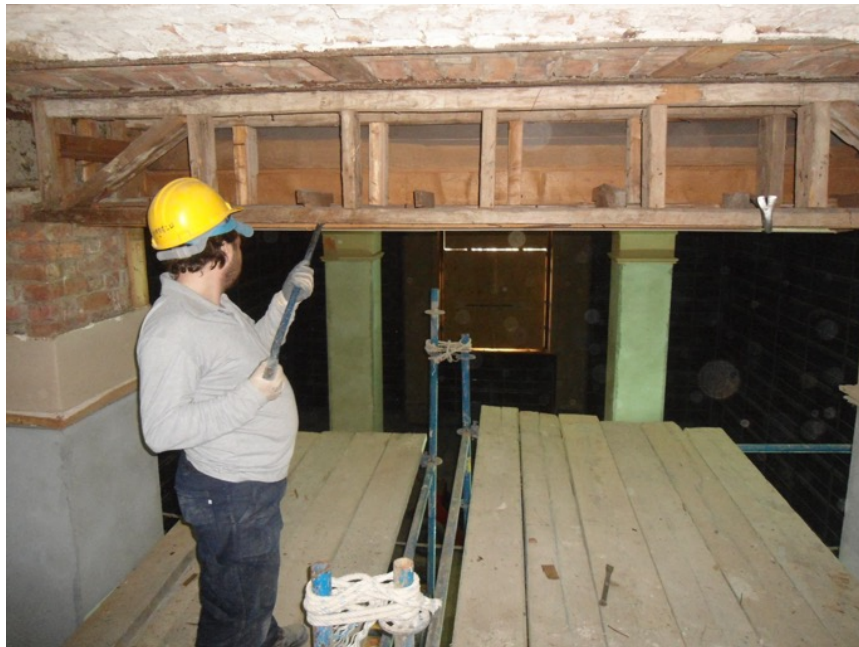
Figure 266. The removal of timber cornices (source: Güryapı İnşaat , IDSM Archive)
