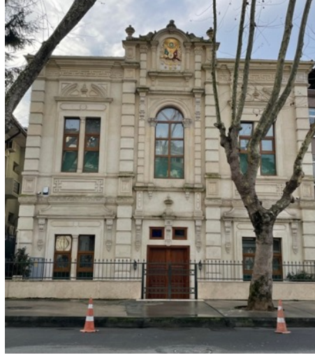
Figure 32. Yeniköy Military Service Building ( Yeniköy Karakolhane-i Hümayun )
