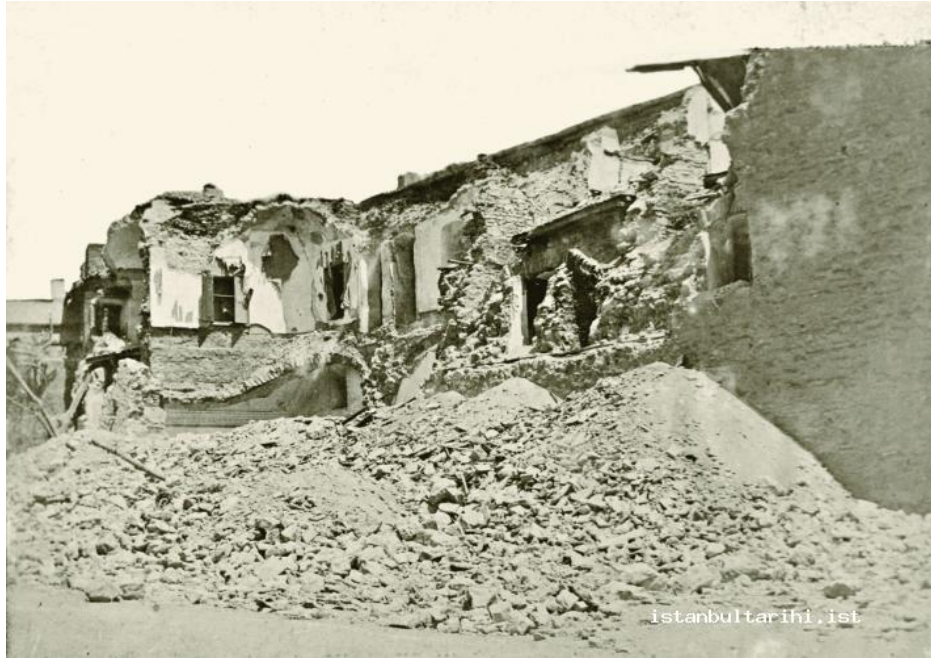
Figure 45. The 1894 earthquake and the damage it caused in Istanbul (source: İstanbul Atatürk Kitaplığı - https://istanbultarihi.ist/27-bir-sehir-manzarasi-istanbulun-tarihinde-depremler )
