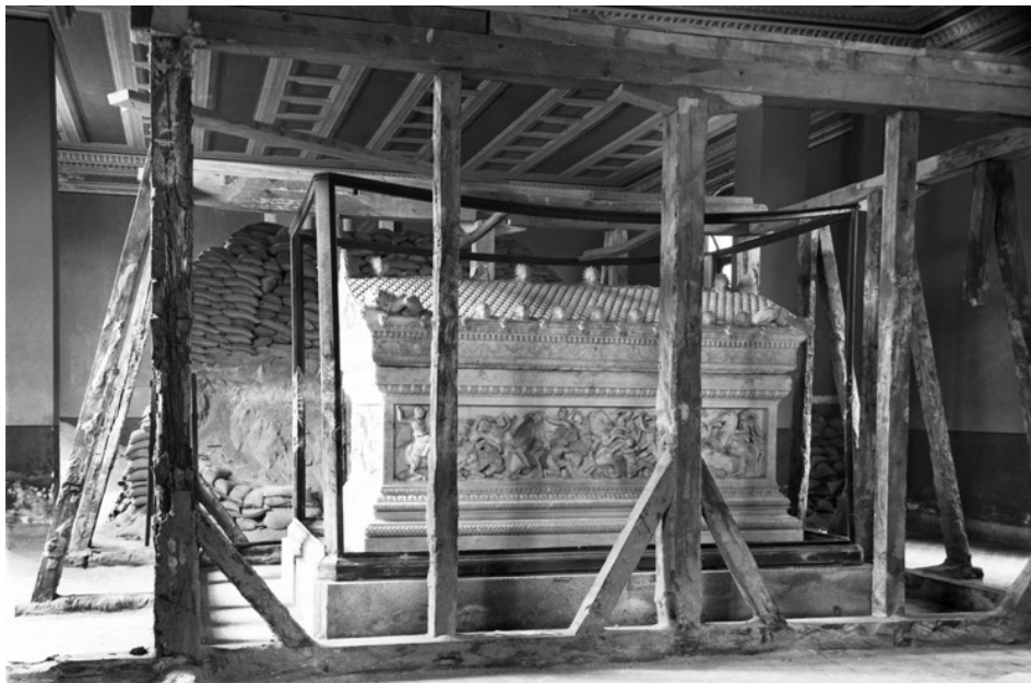
Figure 108. The sarcophagus of Alexandre the Great after taking the Interventions done for the protection of the museum and its artifacts against air attacks during World War I (source: IAM-Photography Archive)
