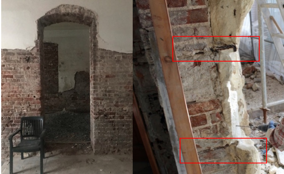
Figure 33. Left: The inner walls of historical Yeniköy Military Service Building, inside (source: IDSM Archive) (right) the section of exterior brick masonry wall with stone cladding
