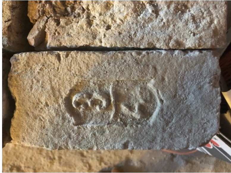
Figure 154. A solid brick example used in IAM building taken from a partition wall added to the building in later periods (taken by the author in 2018)
