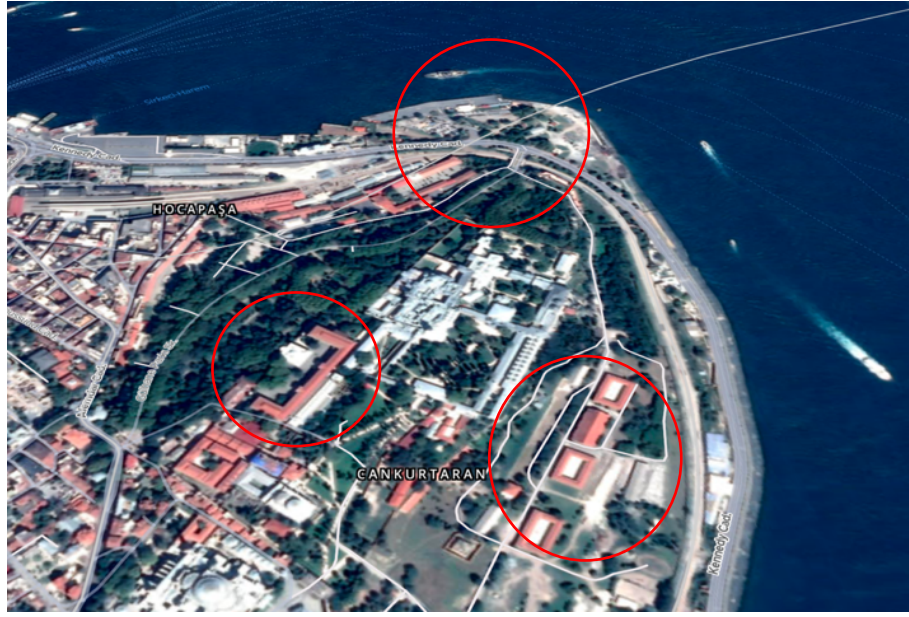
Figure 174. The place of Sarayburnu IAM building and Military Warehouses (source Google Earth Image, 2024)
