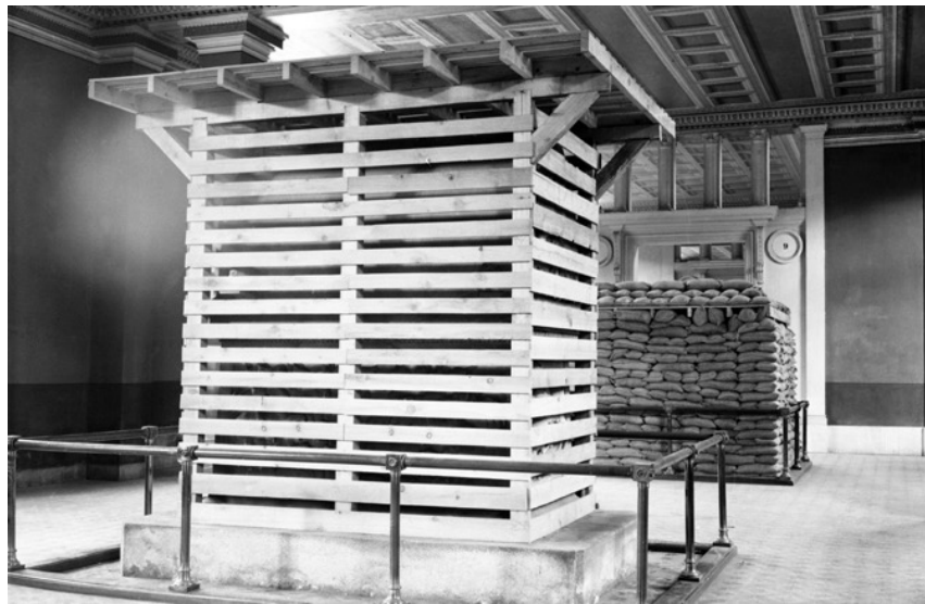
Figure 106. The Interventions done for the protection of the museum and its artifacts against air attacks during World War I (source: IAM-Photography Archive)
