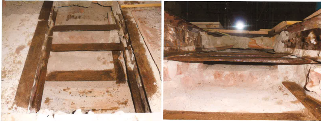
Figure 253. The Photographs of AA section drawing of Hall 23 jack arched flooring details ( Güryapı İnşaat Construction site report, November 2012, IDSM Archive)
