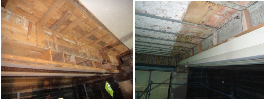
Figure 267. The removal of timber cornices (source: Güryapı İnşaat , IDSM Archive)
