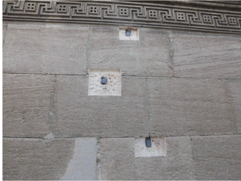
Figure 25. The iron clamps used between brick wall and stone claddings in IAM Building, photograph from 02.10.2012 dated presentation (source: IDSM Archive)
