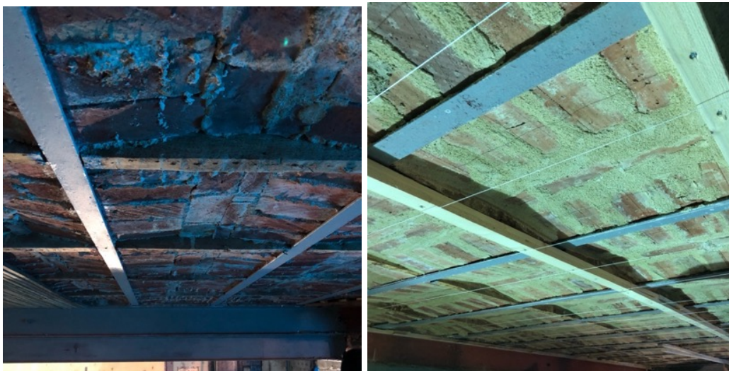
Figure 237. The construction system under the ceiling (taken by the author in 2018)
