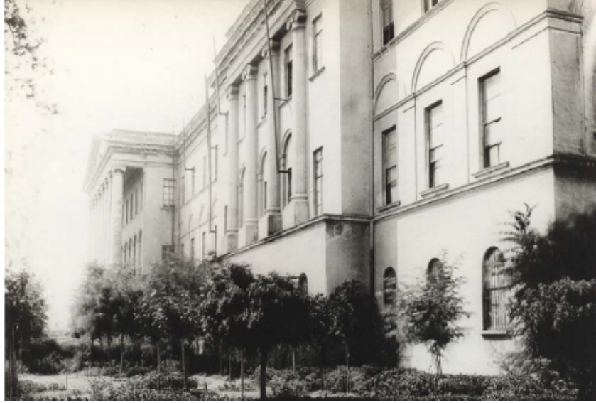
Figure 19. Top: The facade of Darülfünûn Building designed by Fossati near Hagia Sophia (source: Şehbal, 1 Teşrin-i Sani 1325, no 15, 289) (G. Çelik, 2007) Bottom: (source: A.A.E.F.A., Negatif No: R24855) (G. Çelik, 2007, p. 398)
