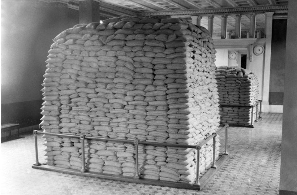
Figure 107. The Interventions done for the protection of the museum and its artifacts against air attacks during World War I (source: IAM-Photography Archive)
