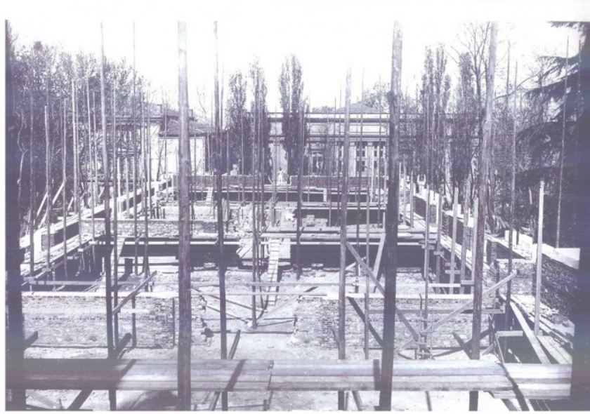
Figure 278. The brick and stone masonry with brick lintel wall construction Techniques of 3 rd Construction Phase of IAM (1904-1907) (source: Restitution Report prepared by Seçkin Mimari Hizmetleri , IDSM Archive)
