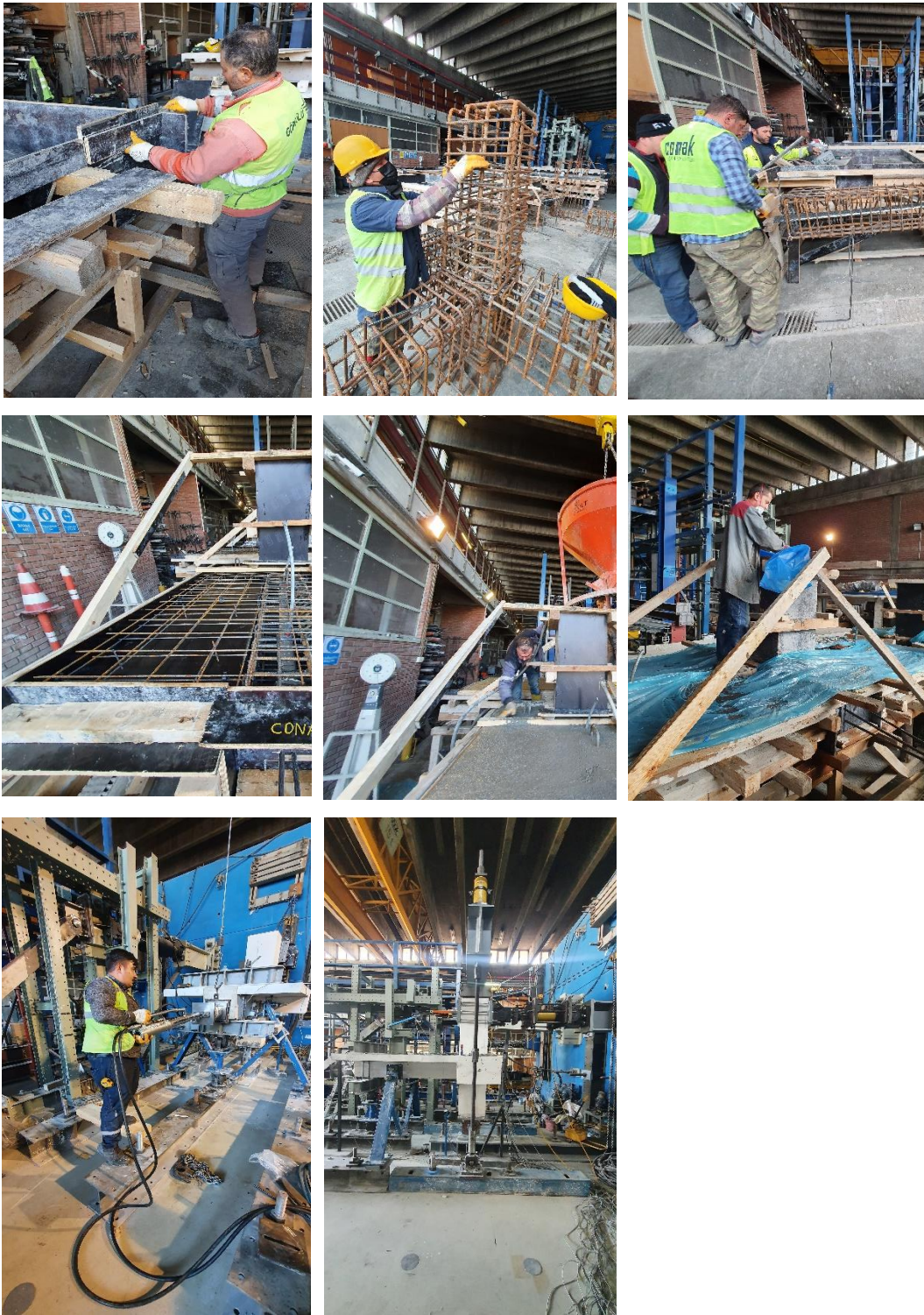
Figure 2.18. Construction stages for PTE-3-75
