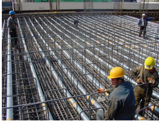
(d) Ankara Sheraton Hotel Culture and Conventional Center, beam-slab
