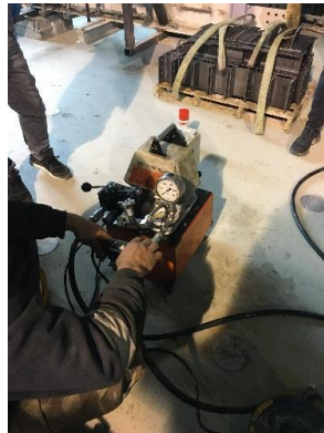
(c) Load pump for prestressing force
