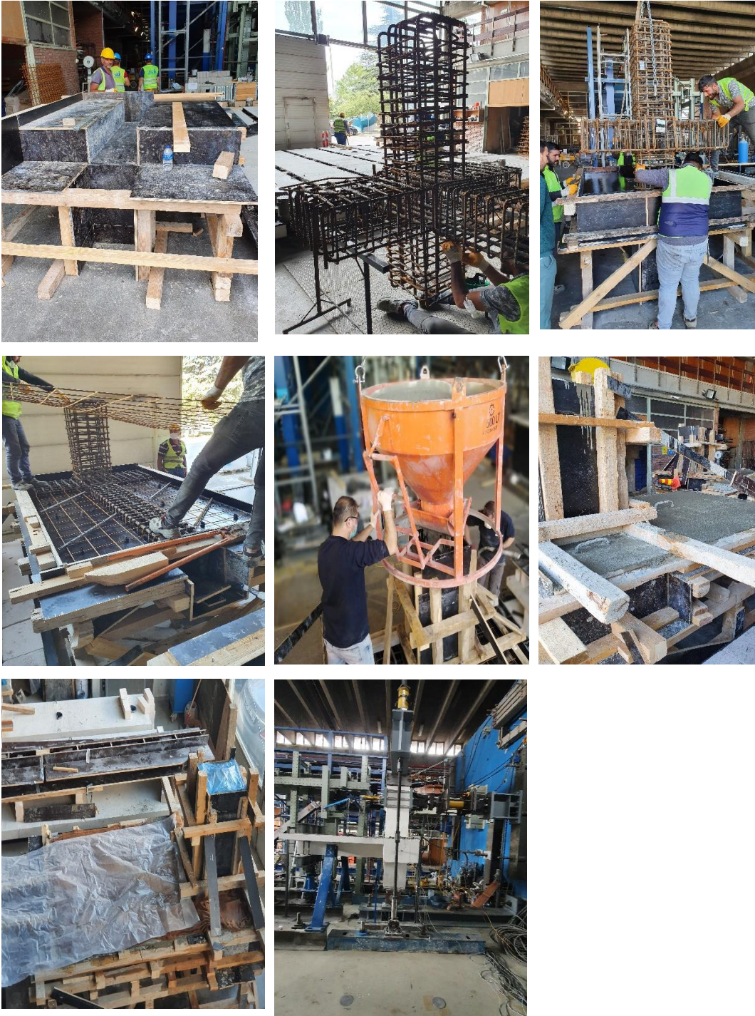
Figure 2.22. Construction stages for RC-10-NA
