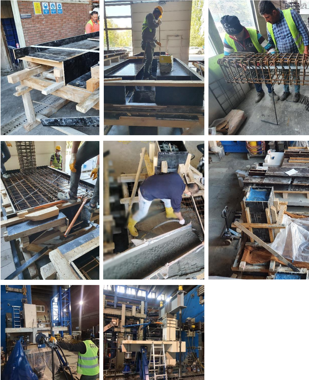
Figure 2.16. Construction stages for PTE-4-50
