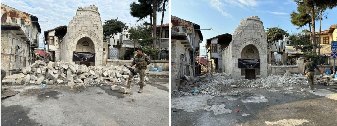
Figure 54. Collection of Scattered Construction Materials at Sarımiye Mosque, Hatay Following the Earthquakes
