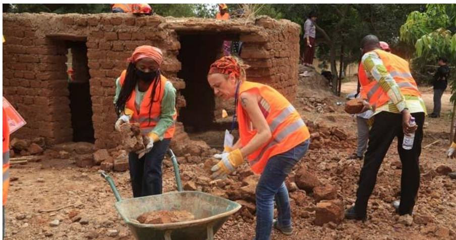
Figure 34. Removal of Debris 102
