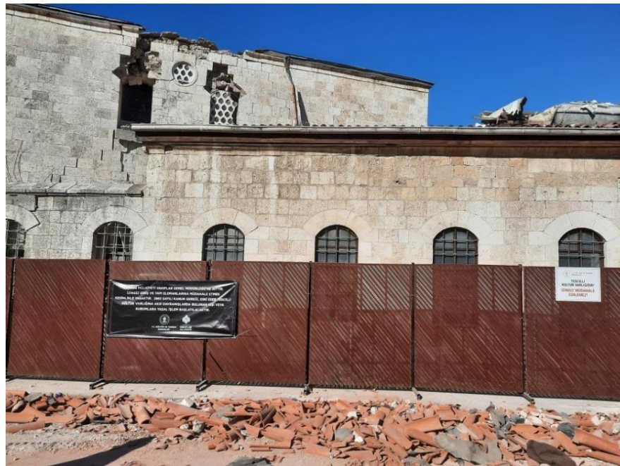
Figure 53. Protection Measures Applied for Habibi Neccar Mosque, Hatay
