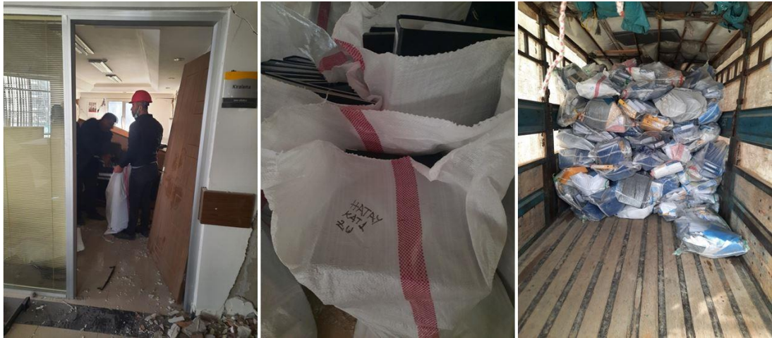
Figure 57. Evacuation of Electronic Devices and Folders from the Directorate's Office Building, Hatay
