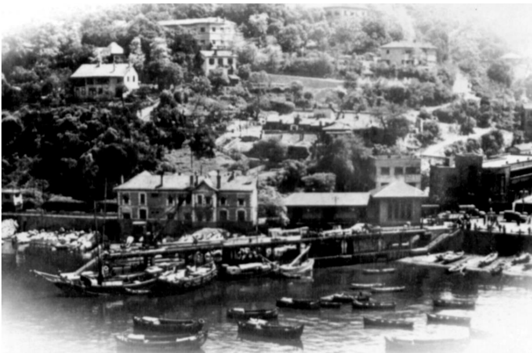
Figure 88: Concrete pier of Zonguldak Port, Workers Management Building on the western side of the pier, 1930, (top), retrieved from https://www.facebook.com/photo/?fbid=667693230048106&set=a.384019231748842 , Concrete pier from front view (bottom), taken from the archives of Zonguldak Directorate for Culture and Tourism
