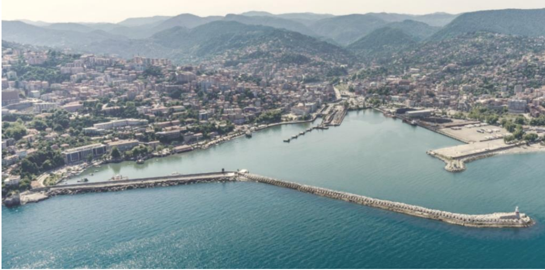
Figure 142: Breakwaters of the Industrial Port of Zonguldak, the city and region in backside, retrieved from https://batikaradeniz.gov.tr/?p=3321
