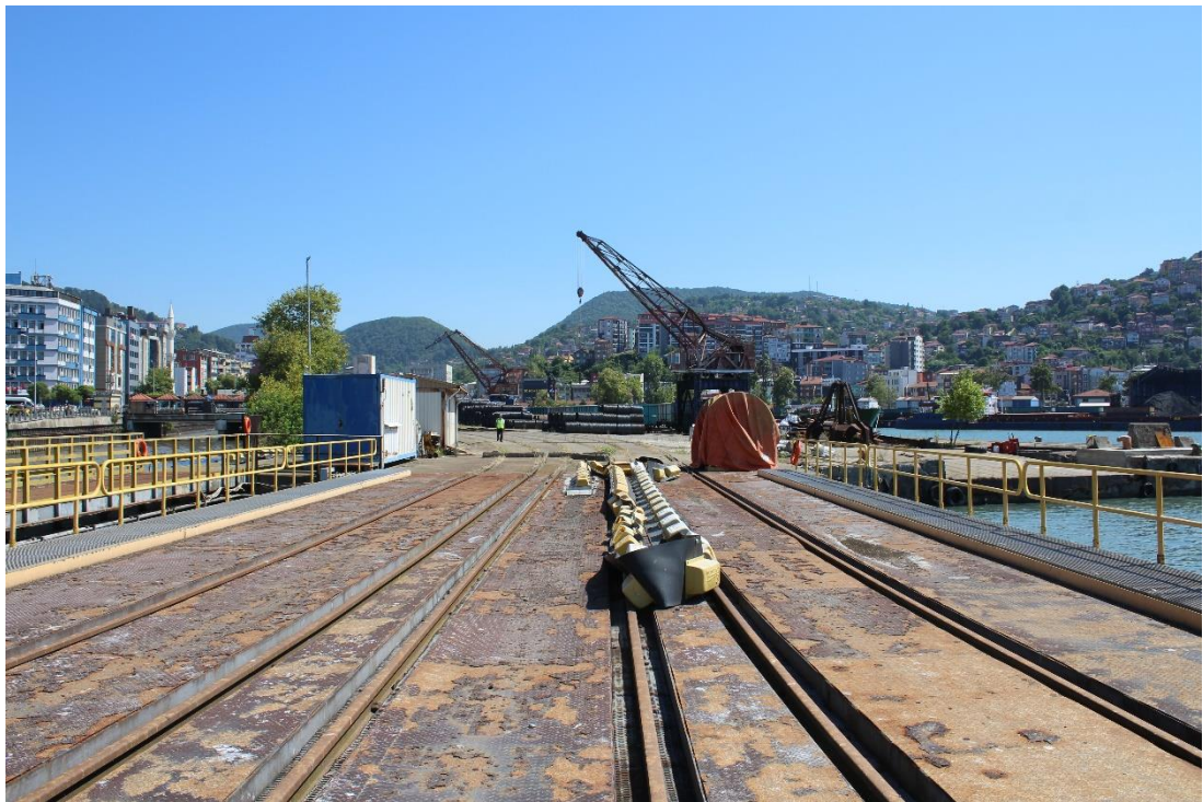
Figure 41: Hydraulic ramp (top), railway tracks and connection with Cargo Dock (bottom), photographs taken by the author
