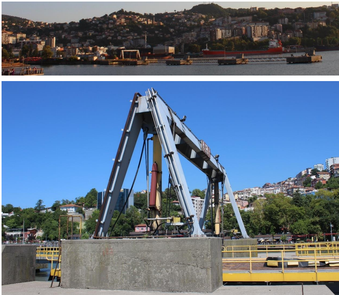
Figure 140: Train ferry dock (top), hydraulic ramp (bottom), photographs taken by the author
