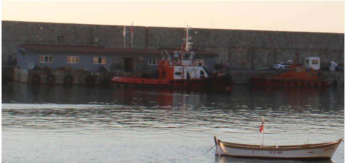
Figure 63: Ship Services Building, photograph taken by the author
