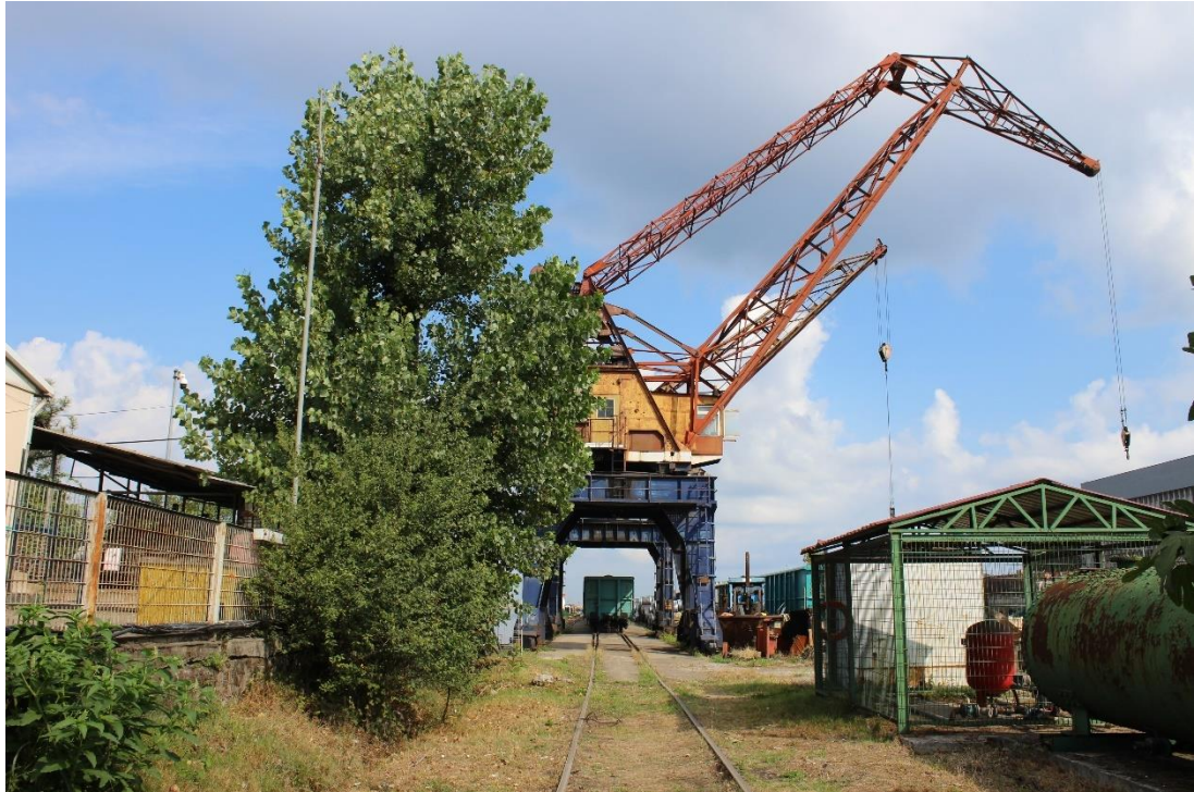
Figure 135: Electric-powered cranes and its railroad tracks, photograph taken by the author
