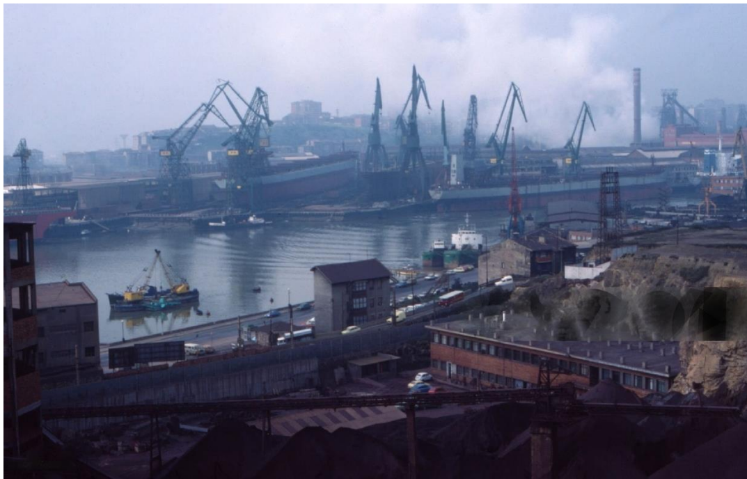
Figure 21: Industrial Port of Bilbao, mid-20th century, in original location along River Nervion, retrieved from https://www.gettyimages.com/detail/news-photo/port-sur-le-nervion-%C3%A0-barakaldo-dans-la-banlieue-de-bilbao-news-photo/1147968375
