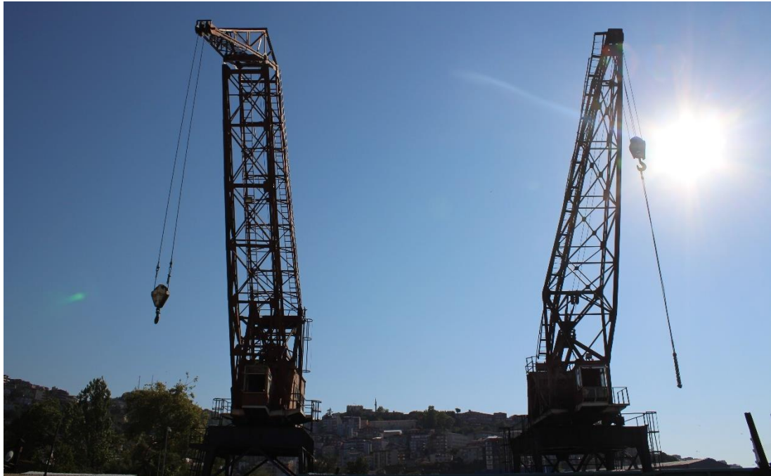
Figure 141: Electric-powered cranes, photograph taken by the author
