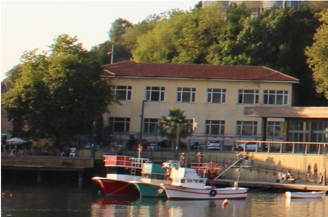
Figure 62: Vacant Building, photograph taken by the author
