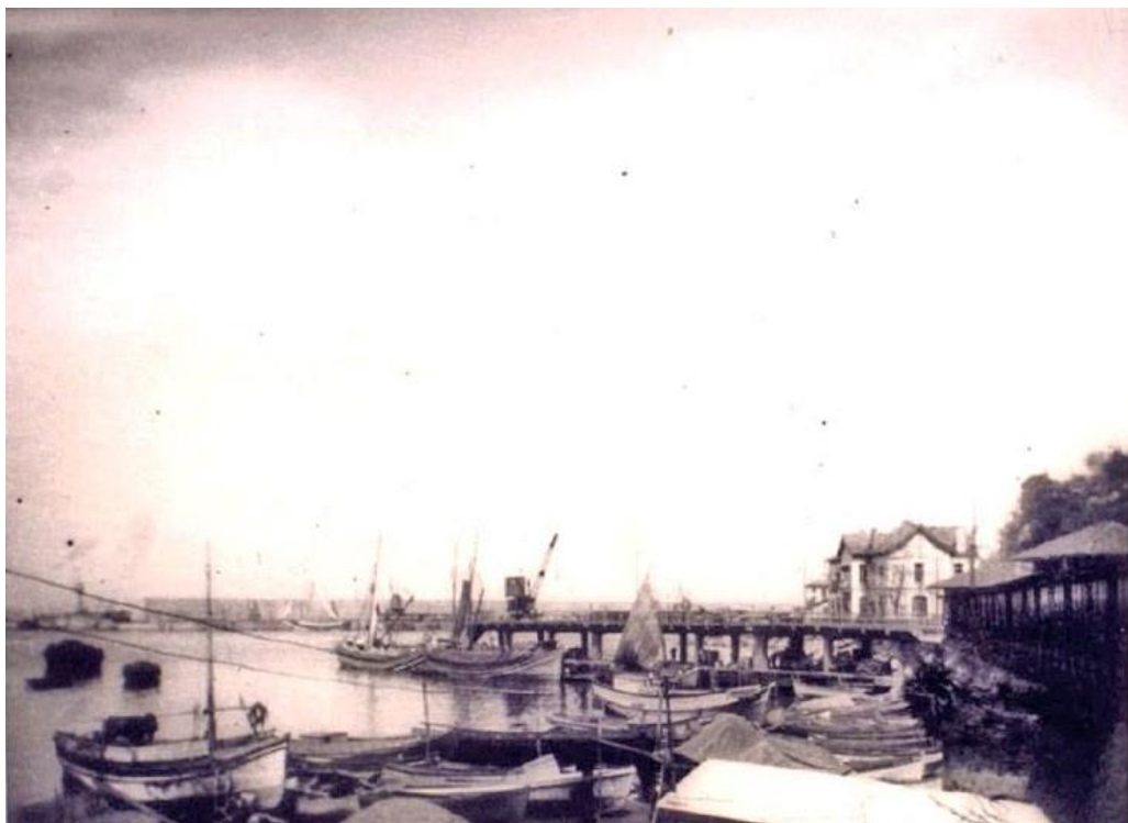
Figure 81: Port of Zonguldak, Breakwater, Loading Cranes and Dock, 1896-1906, (top) retrieved from
