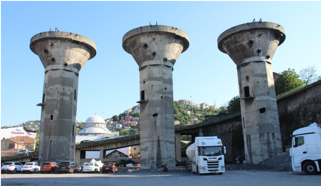
Figure 52: Previous filtering and storage units of the Zonguldak Central Scrubber, currently referred to as “Lavuar Kuleleri”, photograph taken by the author
