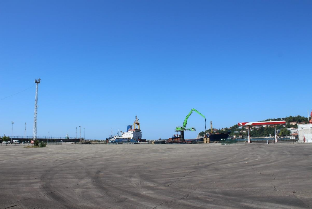
Figure 47: Ro-Ro Dock and ramps (top), Truck Parking Area (bottom), photos taken by the author
