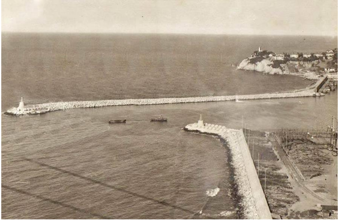
Figure 137: Breakwaters of the port during construction in 1953, kırmızı mendirek (left), yeşil mendirek (right), retrieved from https://www.facebook.com/photo/?fbid=503380209812743&set=a.421319804685451
