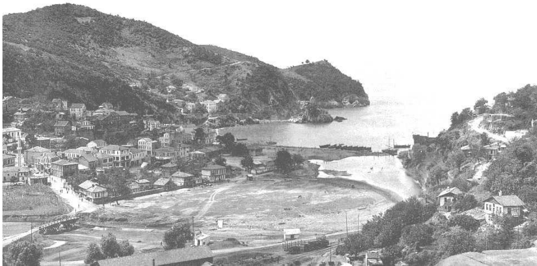
Figure 78: Zonguldak, before construction of the port in 1896, taken from the archives Zonguldak Directorate for Culture and Tourism
