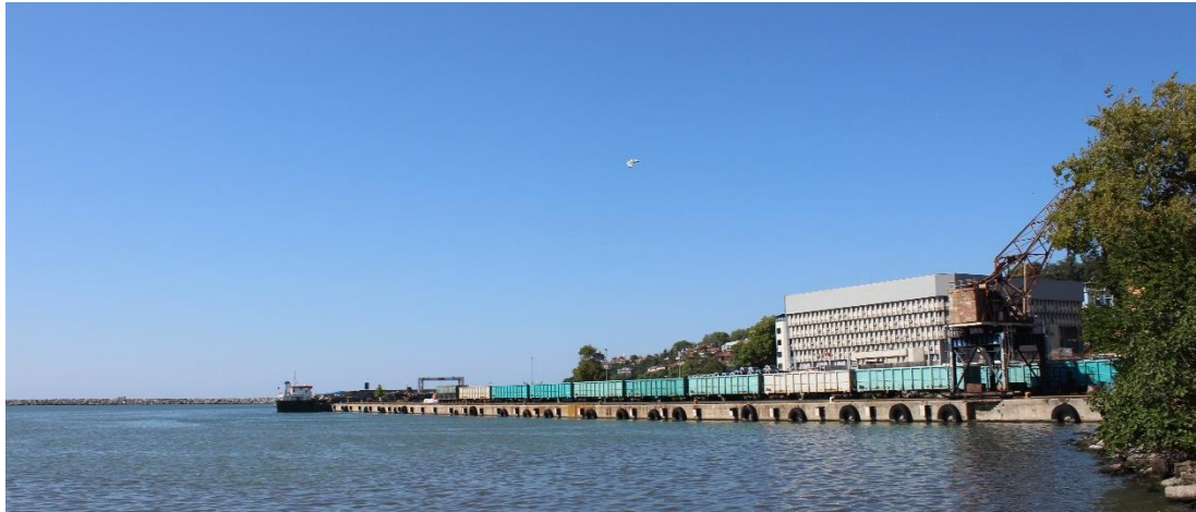
Figure 145: Cargo Dock, photograph taken by the author
