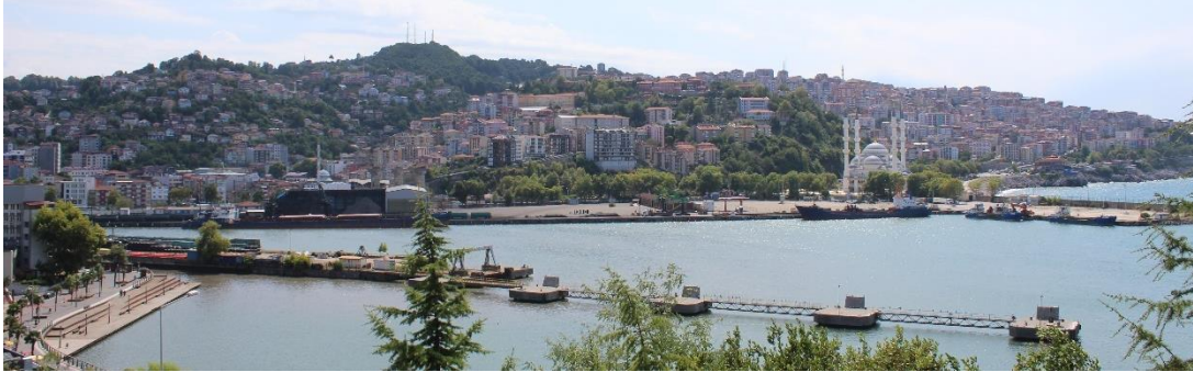
Figure 132: Landfill of cargo, bulk cargo and ro-ro docks, taken by the author
