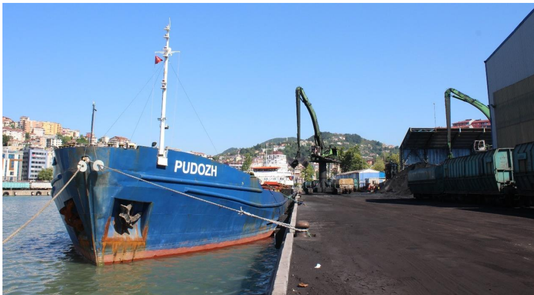
Figure 45: Bulk Cargo Dock, photograph taken by the author
