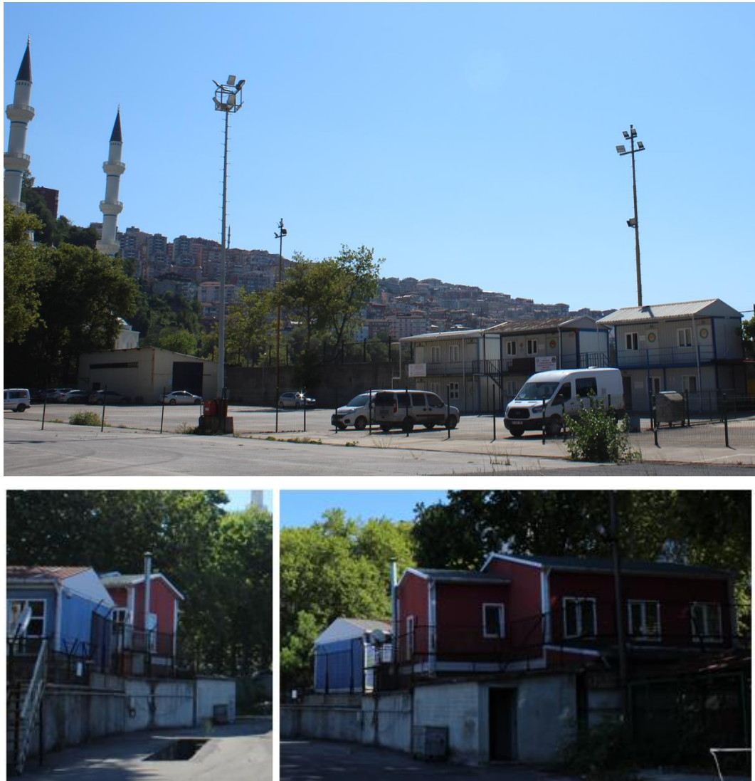
Figure 53: Customs Buildings (top), buildings of 3rd party companies (bottom), photographs taken by the author
