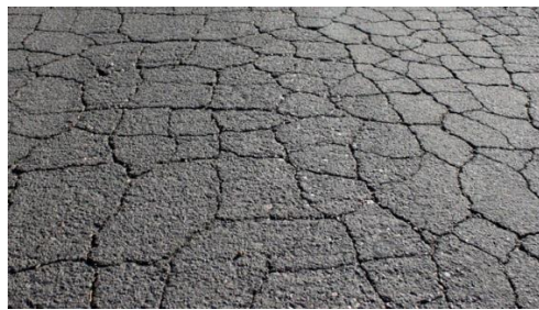
Alligator Cracking
