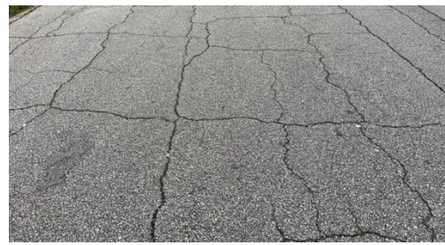
Block Cracking
