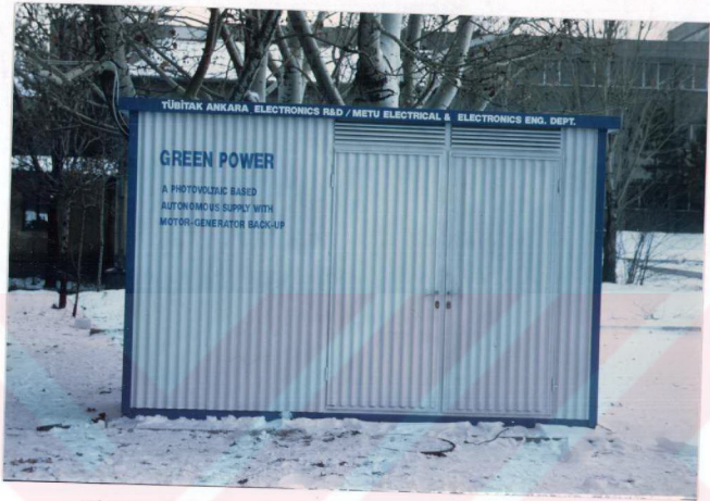
Figure 1.2 The Photograph of the Shelter Building
