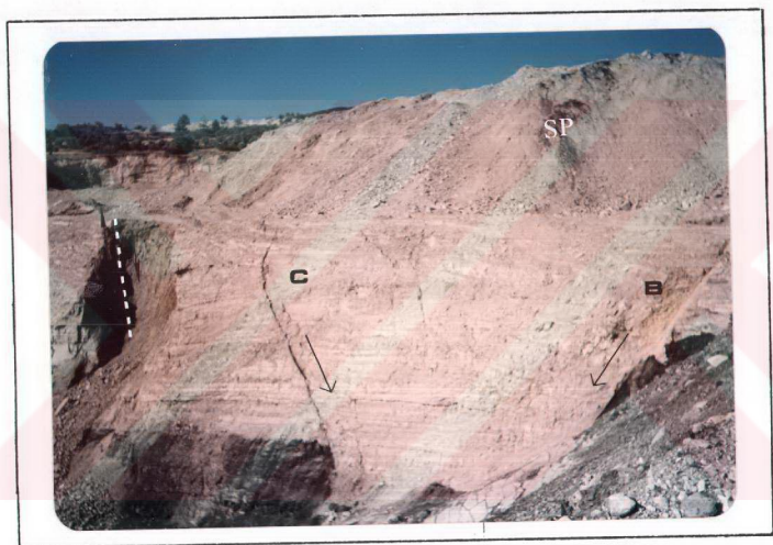
Figure 40: Slide initiation and separations along faults B and C in the new highwall at the south of ninth slice (SP: spoil pile; Plate 3-Photo. No.21).
