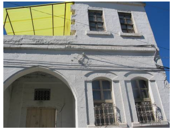
Figure 3.74 Unfinished stone masonry construction expressing open-ended construction
