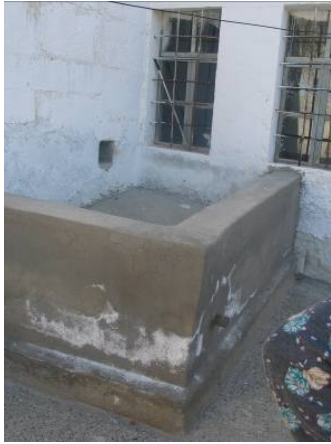
Figure 3.78 Pools in courtyard for pressing grapes
