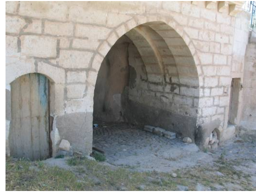
Figure 3.42 Laundry II in Old Square
