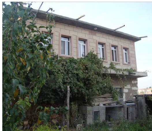
Figure 4.9 New building in Körgümiş Mahallesi
