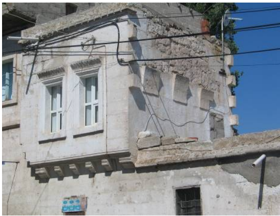
Figure 3.73 Unfinished arches and stone masonry construction
