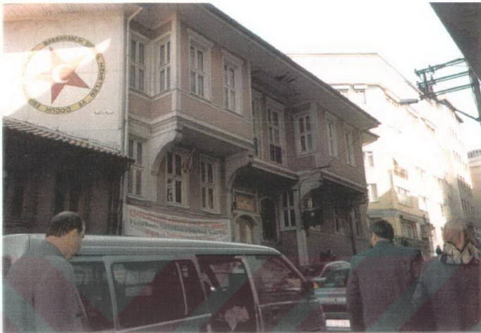
Plate 49. Namazgâh Street, No: 17 (March-2001)
