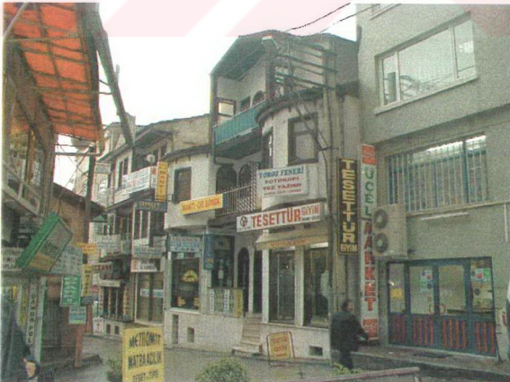
Plate 59. Kanara Street, No: 10 (October-2000)
