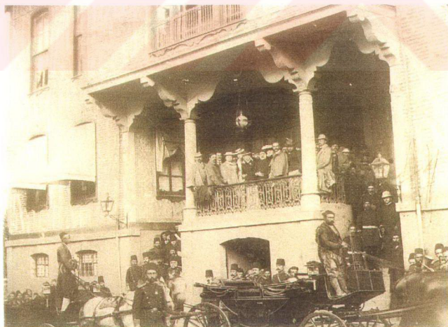
Plate 16. Entrance of the Municipality Building (Papazyan-1901)
