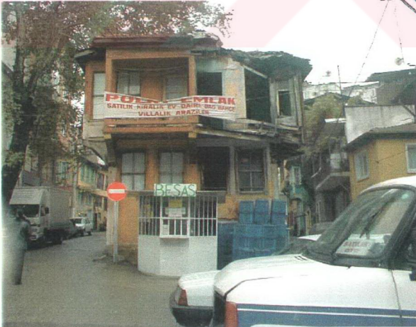
Plate 68. Kanara Street, No: 27 (October-2000)
