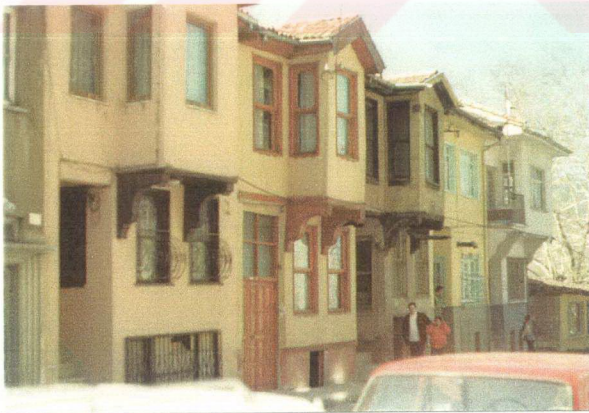
Plate 33. Row Houses on the Eşrefiler Street, No: 16-22 (March-2001)
