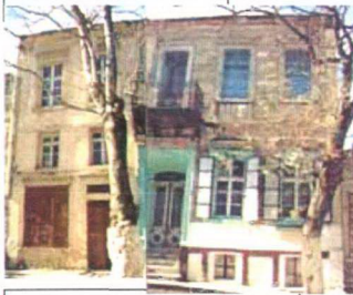
Figure 2.1.9 Restored Building İzmir Cadesi No:56
