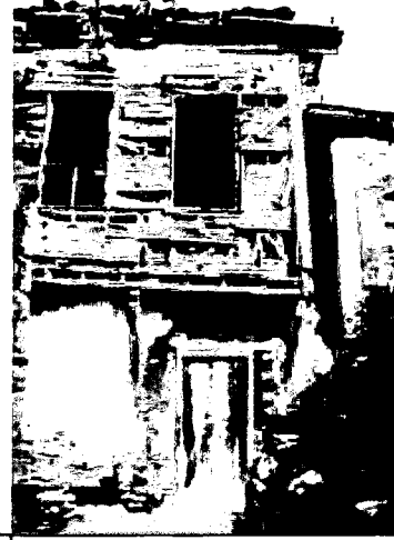
Figure 2.3.2 Orkun Sokağı No:9 Example of Wooden Skeleton Construction System
