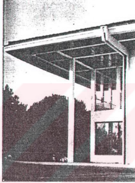
Fig.4.78 Sertel Köşkü, Yeniköy. Details of the roof. Source: Eldem (1982).
