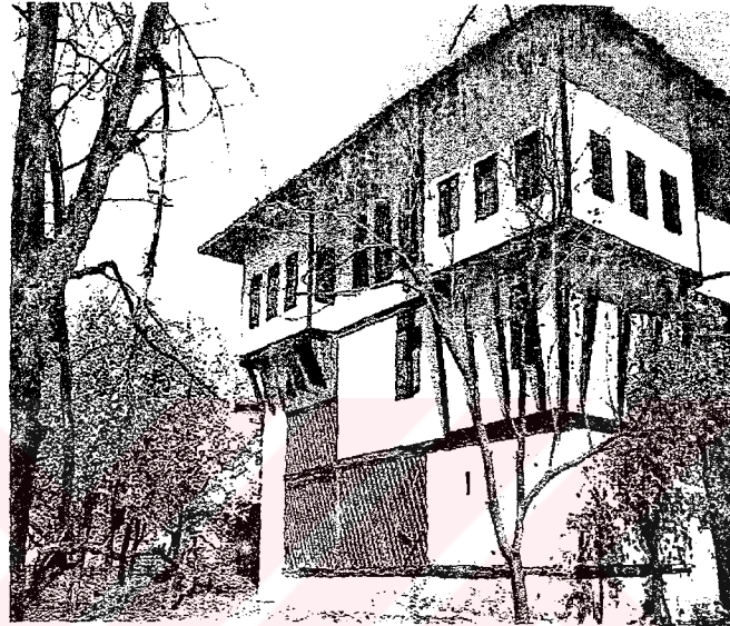
Fig.3.35 Safranbolu House, North-west Turkey. Source: Yenal (1987).
