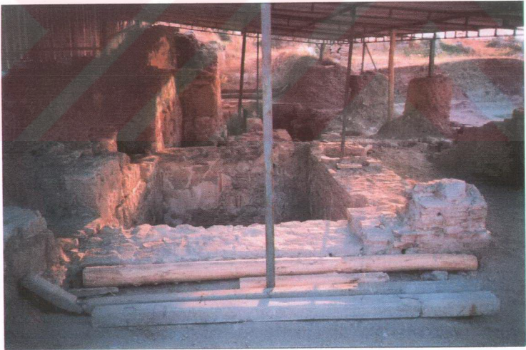
Fig. 5.19 The Shelter Structure of the Hypocaust Building Seen from the Inside (B.N. Öz, 2001)
