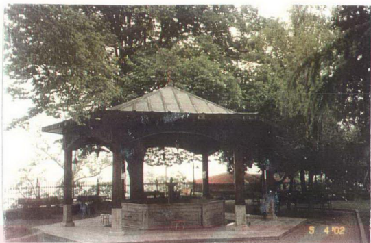
Plate 40. Murat I (Hüdavendigâr), fountain.
