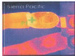
b) Electrical hot connection
