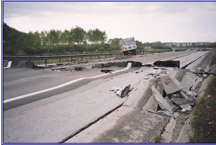
Figure 2.2. Roadway in Izmit after August 1999 EQ
