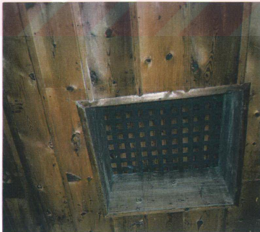
Figure 3.12 Peep hole on the 1 st floor's flooring
