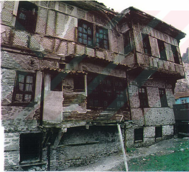
Figure 3.3 South-east façade of the dwelling
