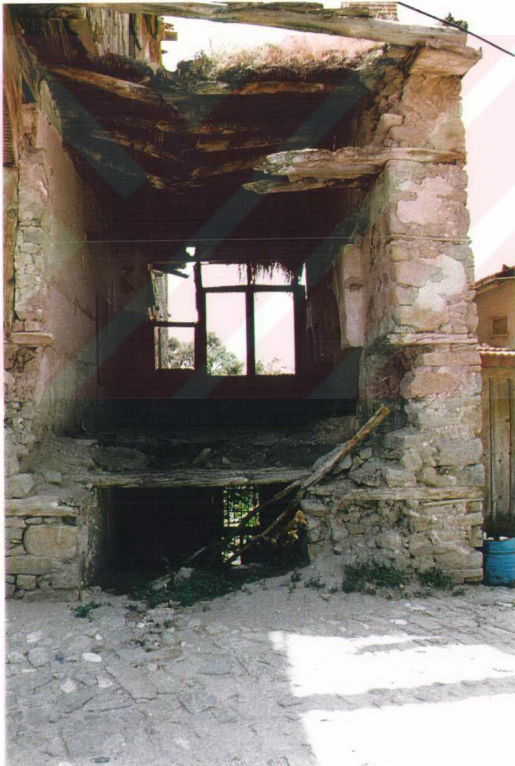
Figure 3.10 View through space SG-01
