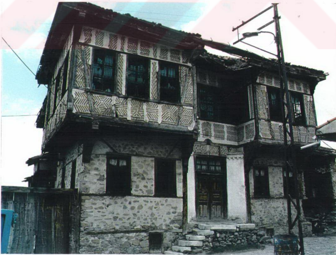
Figure 3.1 North east façade of the dwelling
