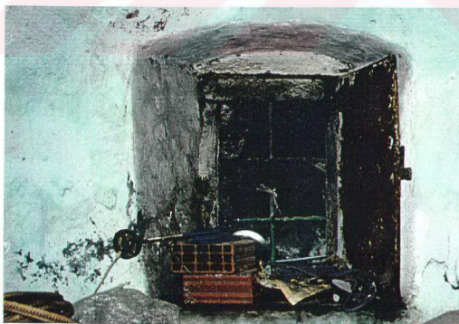
Figure 25- Window on the South wall of Space 11
