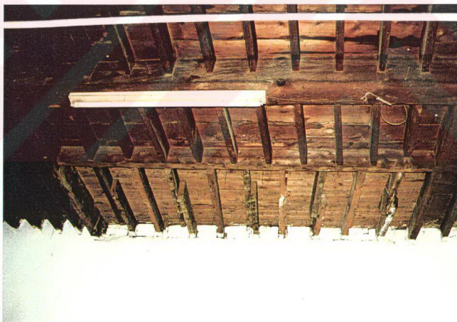
Figure 27- Trace of staircase in Space13
