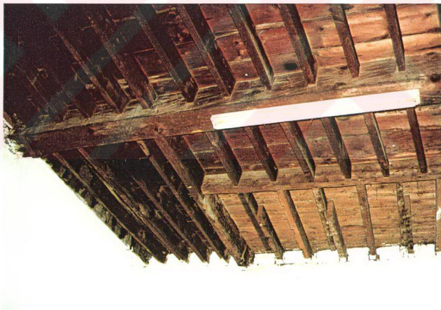
Figure 22- Timber beams and joists separating two floors in Space 13
