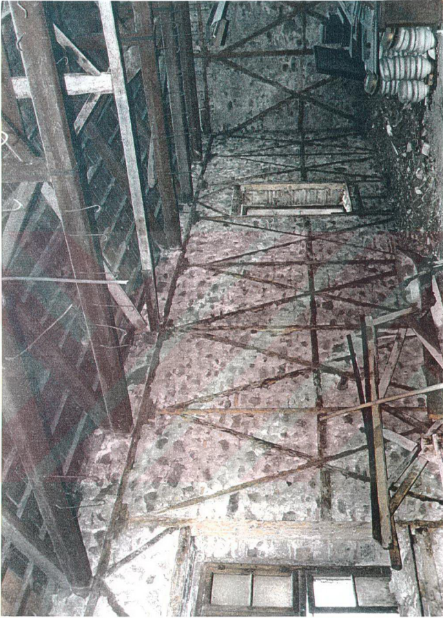
Figure 14- Space 1 and Space 2 First Floor North East Wall
