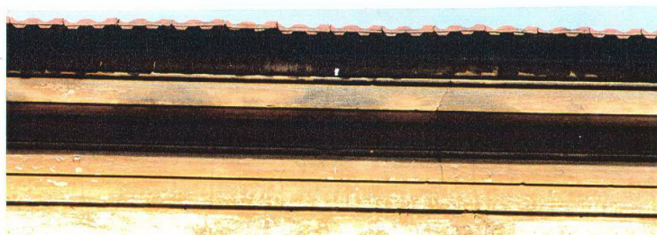
Figure 28- Eave of South West elevation facing courtyard
