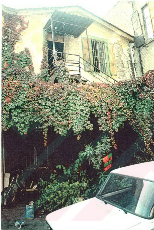
Figure 17- East wall facing courtyard (Space 17)
