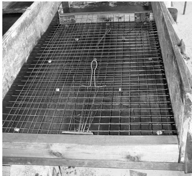
Figure 4.1: The reinforcement of the concrete shearwall
