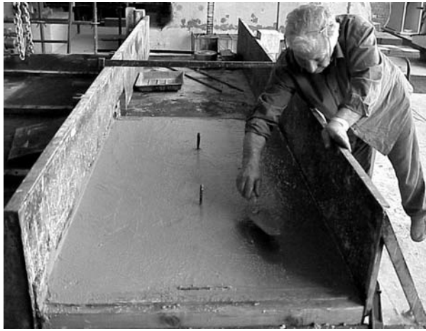
Figure 4.2: The fresh concrete of the shearwall
