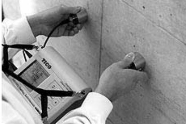
Figure B.4: Another application of TICCO
