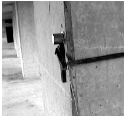
Figure 4.31. Interior column of the 24-storey high building
