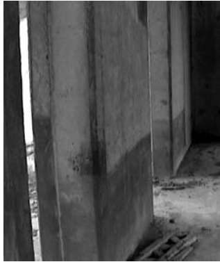
Figure 4.33. Shearwall (interior) of the 24-storey high building
