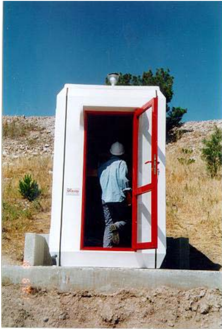
Figure 4.3 General view of BG2 station
