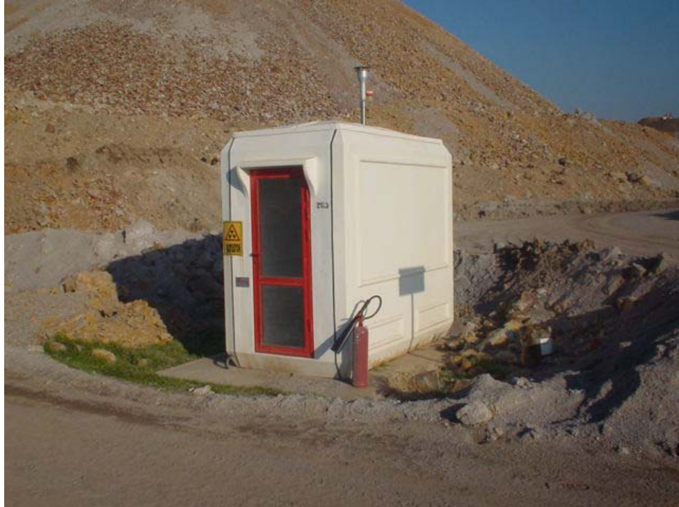
Figure 4.4 General view of BG3 station
