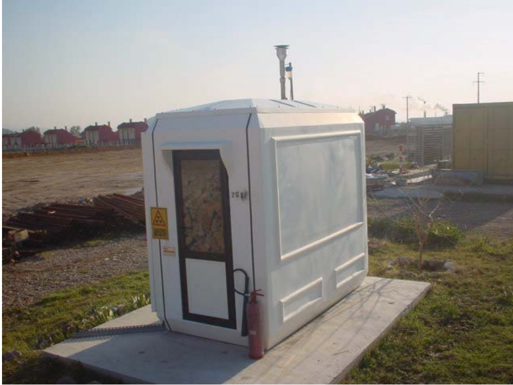
Figure 4.2 General view of BG1 station
