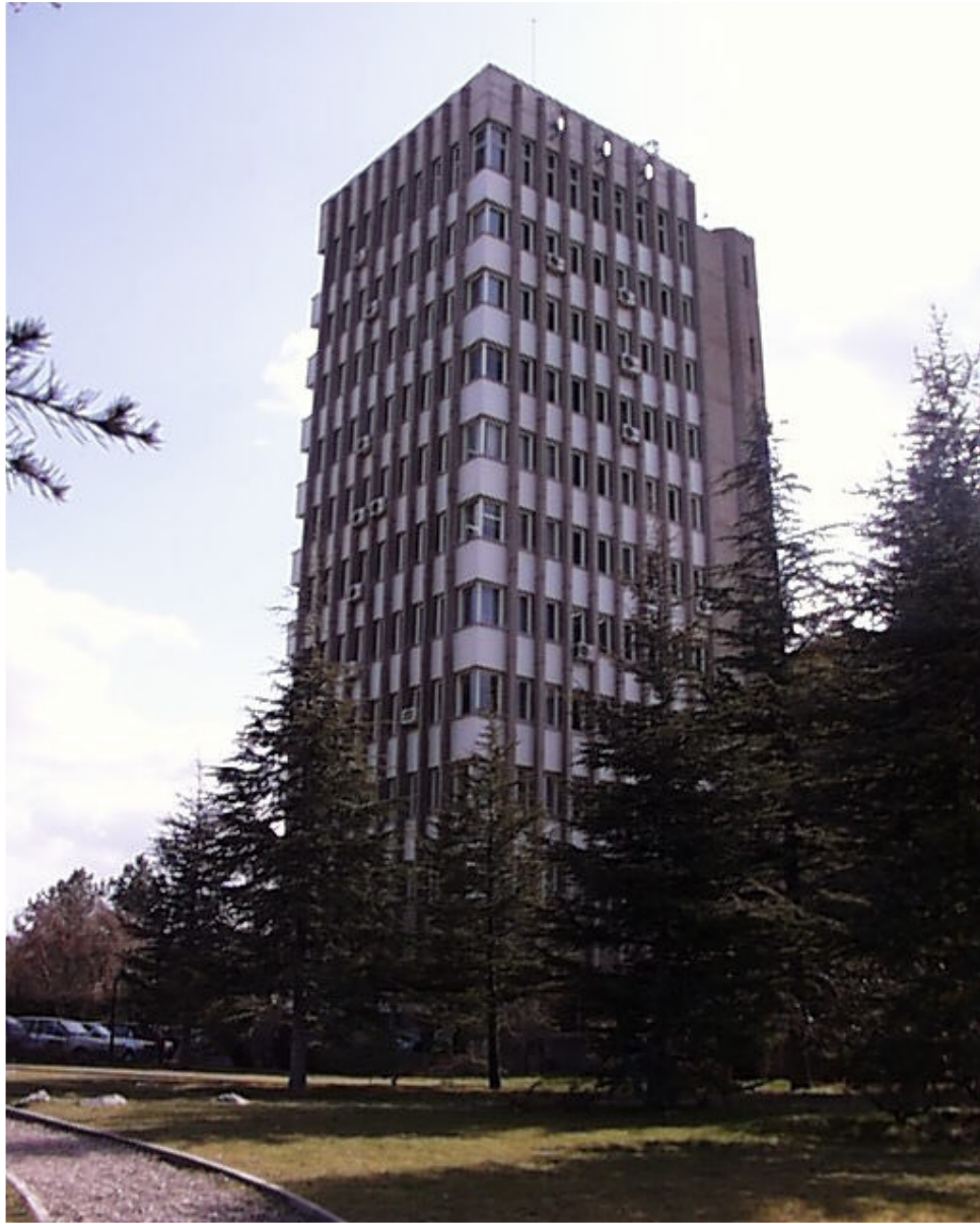
Figure 3.2 General view of case study MM building
