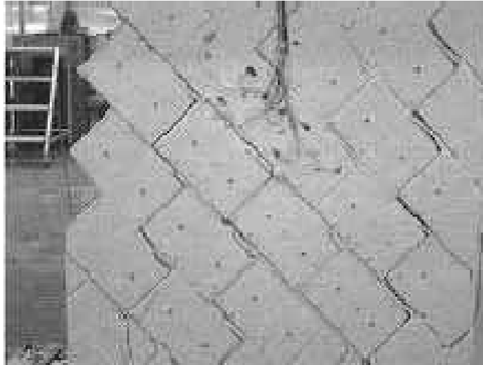
Figure 2.6. Sliding failure along joints
