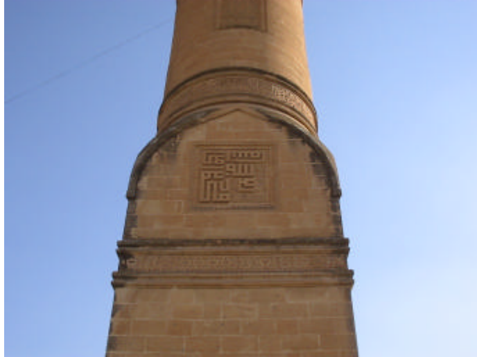
Figure 5.14. Special handworks on the Sultan Süleyman Mosque's minaret
