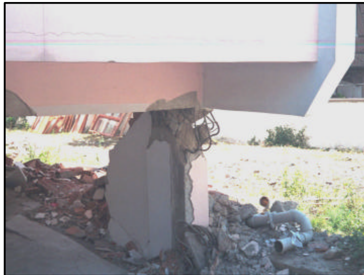
Figure 2.21: Short-column effect [40]
