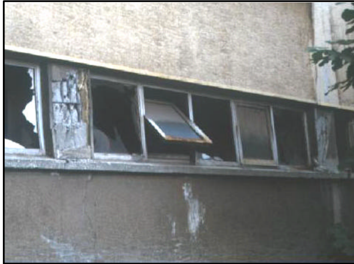
Figure 2.20: Short-column effect [40]
