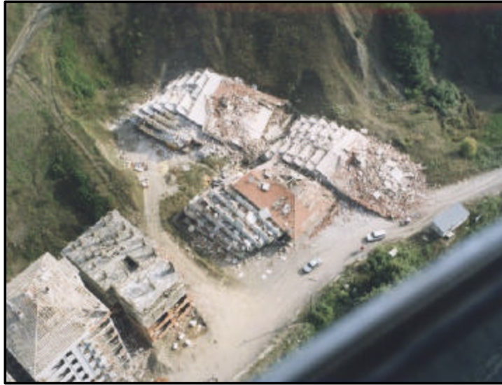
Figure 2.9: Failures of reinforced concrete structures [30]
