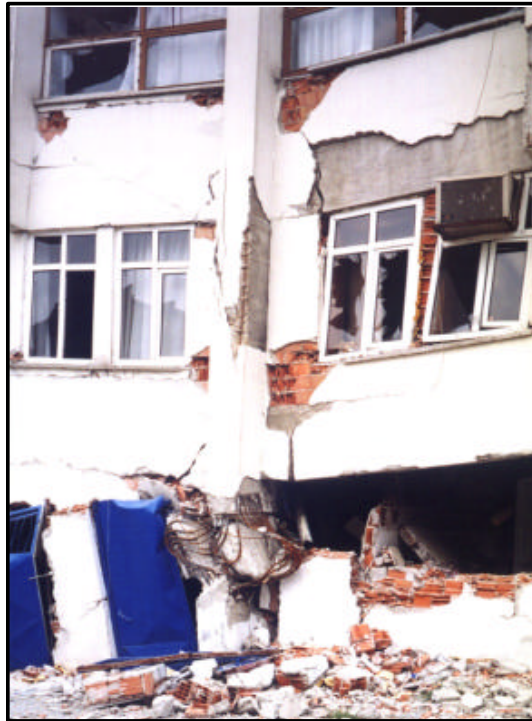
Figure 2.12: Torsion failure
