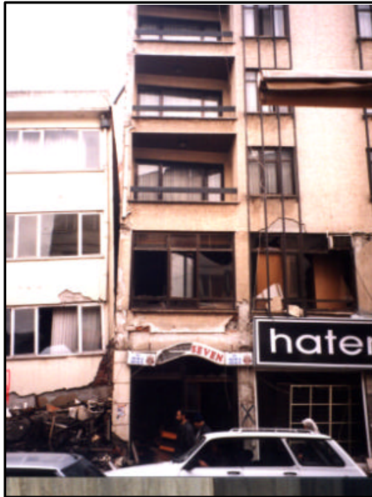
Figure 2.19: The pounding effect
