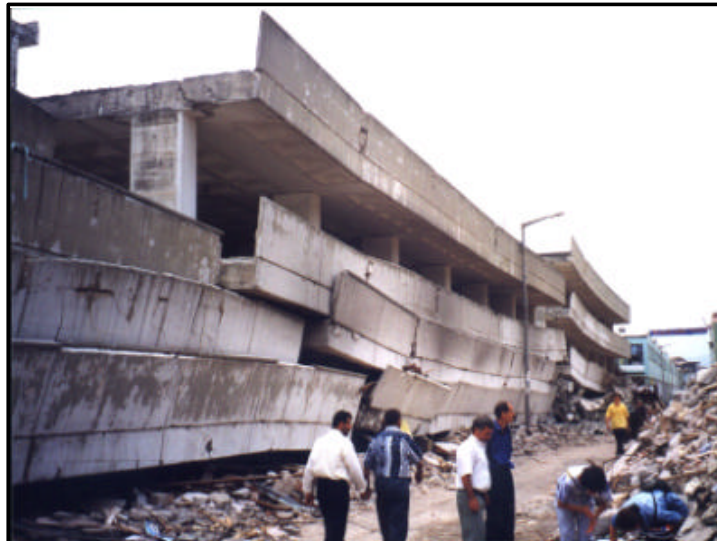
Figure 2.22: Strong beam-weak column effect
