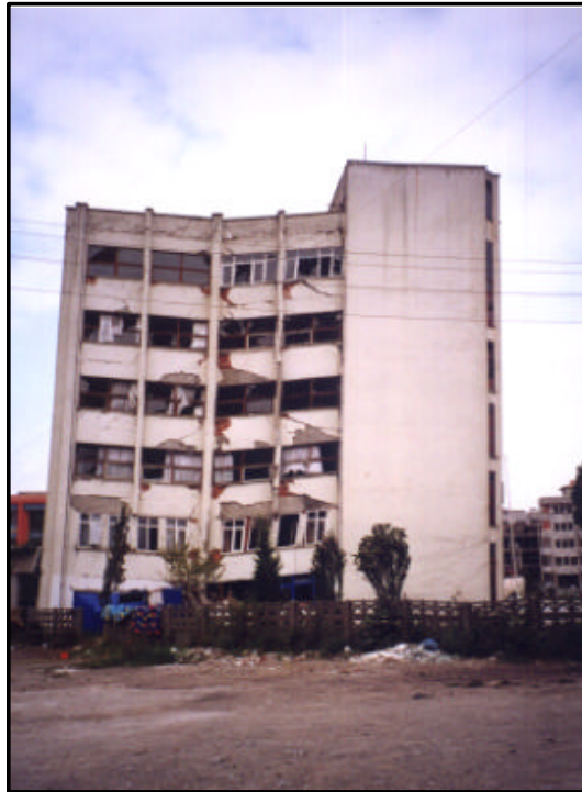
Figure 2.13: Torsion failure
