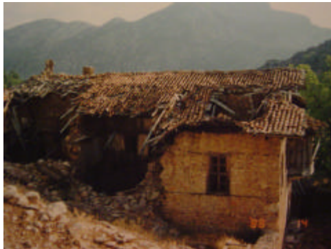
Fig. 132. The North Facade, 1988
