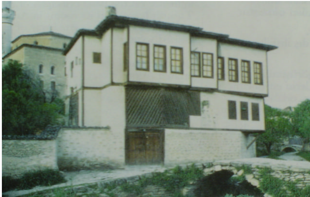
Fig. 5. A House that was Built to Fit to the Available Building Parcel on the Ground Floor, and the Independent Development of the Upper Floor
