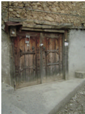
Fig. 81. The Main Entrance Door
