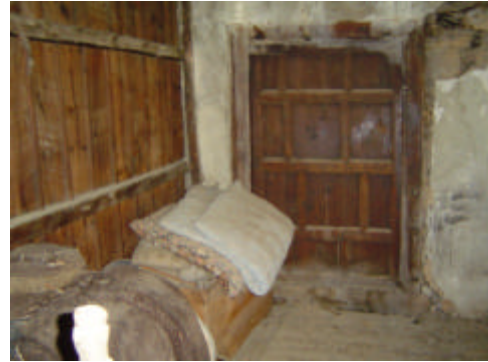
Fig. 73. The Partition between the Old and the New Section
