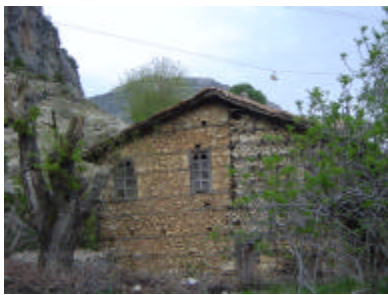
Fig. 78. The West Facade
