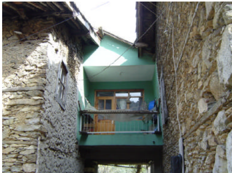
Fig. 104. The Newly Attached Room
