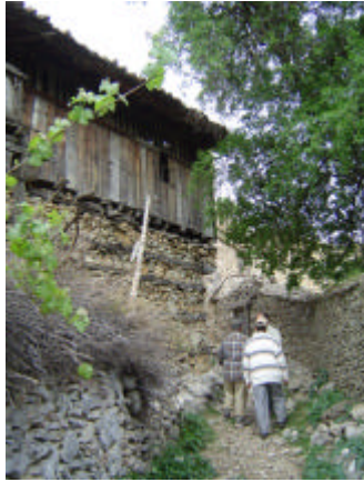
Fig. 77. The South Facade
