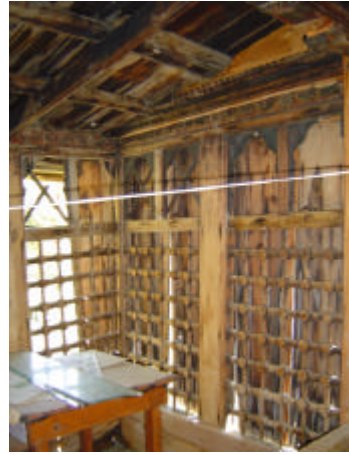
Fig. 152. The Latticework windows of the 'ahni'in
