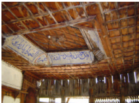
Fig. 164. The Ceiling Ornamentation of Şhni'in
