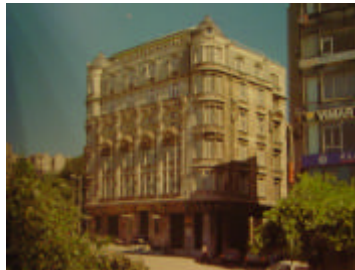
Fig. 14. Frej Apartment in İstanbul
