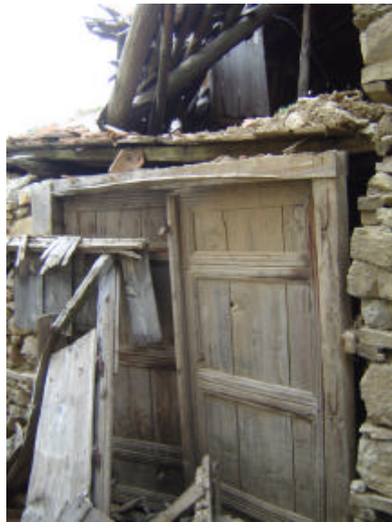
Fig. 98. The Main Entrance Door
