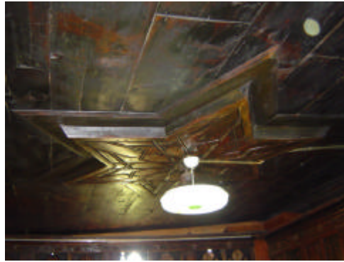
Fig. 151. The Ceiling Detail in ahni'in
