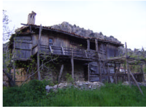
Fig. 89. The Garden Façade
