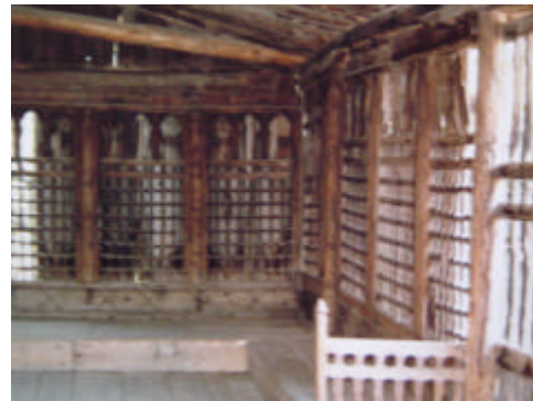
Fig. 123. An Old View of the İhni'in , Before Renovation
