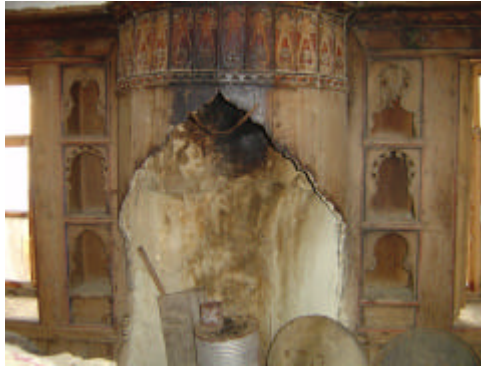
Fig. 166. Davlumbaz and Open Niches
