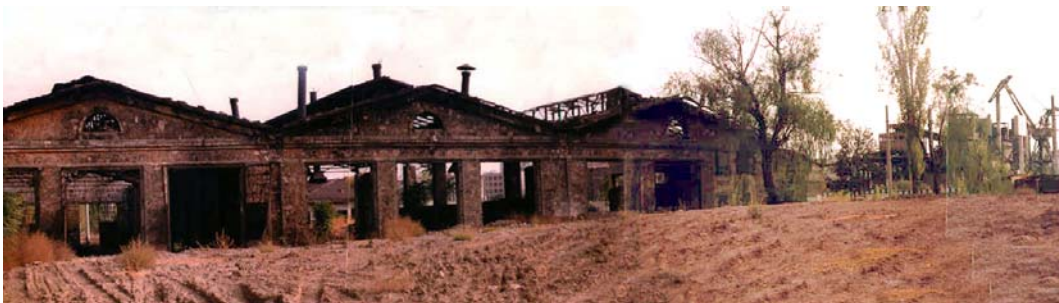
Fig. 3.26. Maintenance ateliers of railways before restoration
