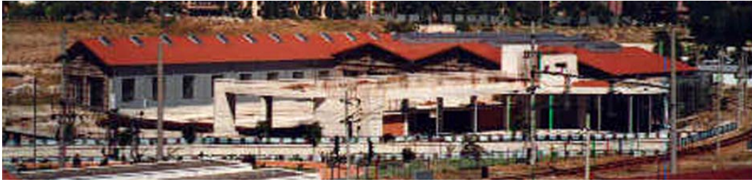
Fig. 3.27. Ateliers after restoration, as a museum of contemporary arts
