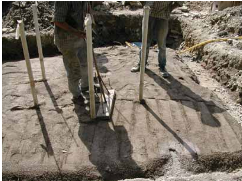
Figure 3.20 Laying and compaction process of sand layer on the loading surface
