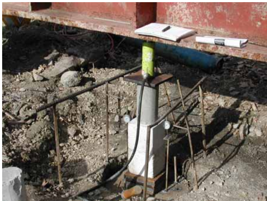
Figure 3.24 Single aggregate pier load test arrangement
