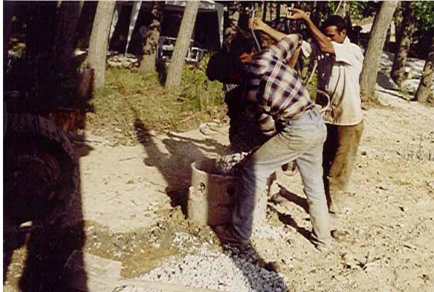
Figure 3.10 Filling the granular material into the borehole
