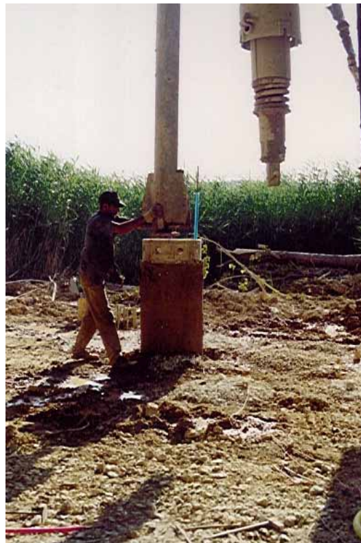
Figure 3.11 A view from ramming operation
