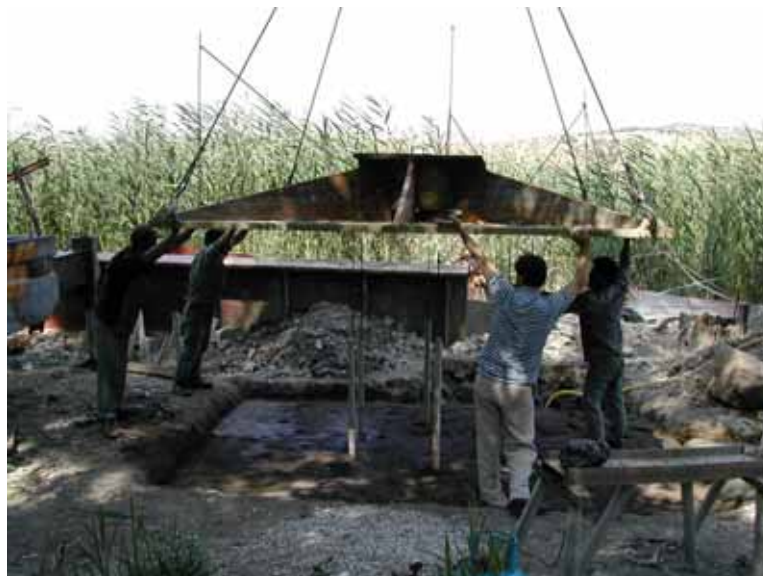
Figure 3.22 Placing of loading plate
