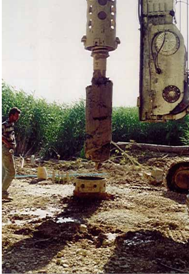
Figure 3.9 Cleaning operation of borehole with auger
