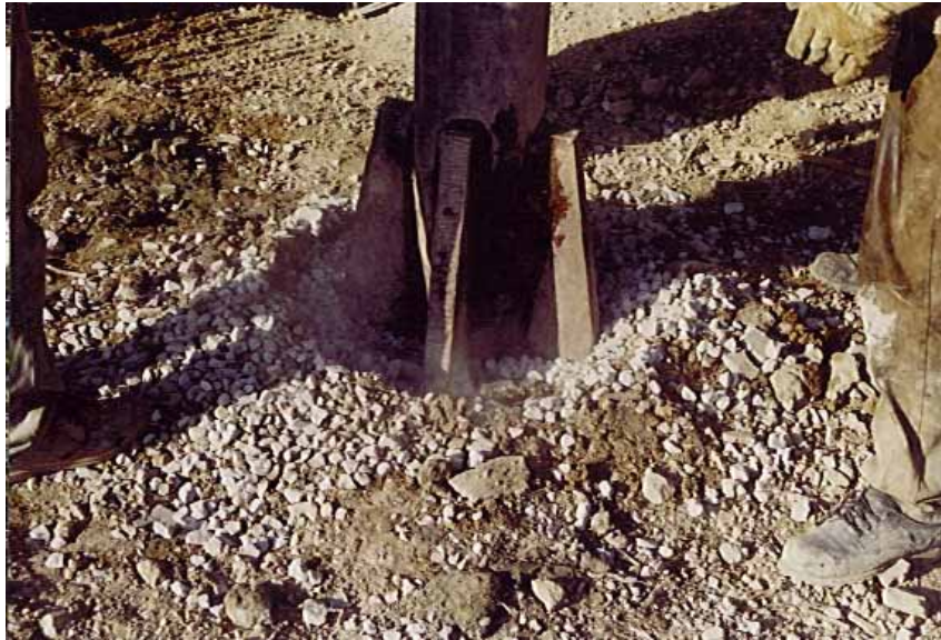
Figure 3.12 A view from completion of aggregate pier
