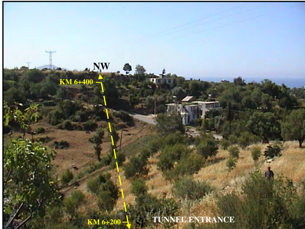
Figure 3.2 General view of proposed Dim Tunnel route from Km 6+200.
