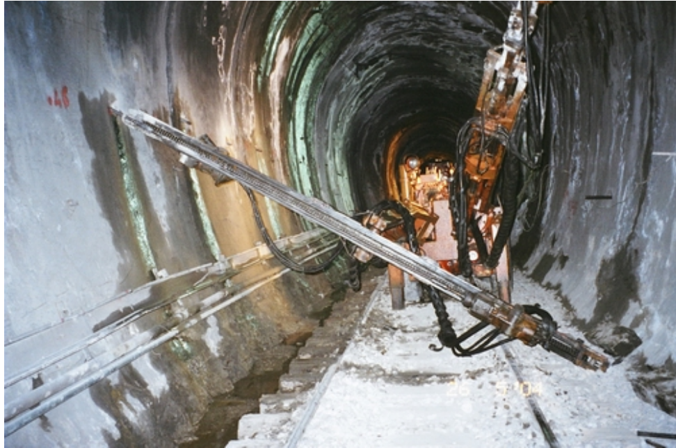
Figure 5.6 Jumbo Used in No: 7 Tunnel for Installation of MAI SDA
