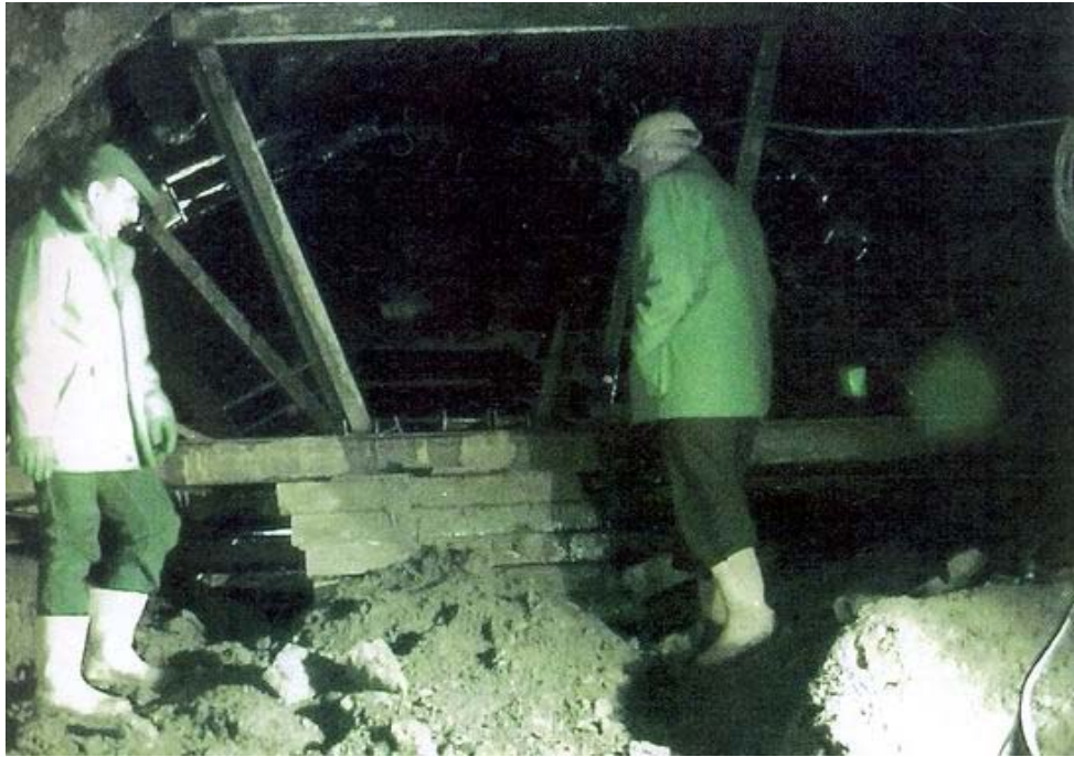
Figure 4.9 Bench Support Used During Clearance of the Collapsed Material
