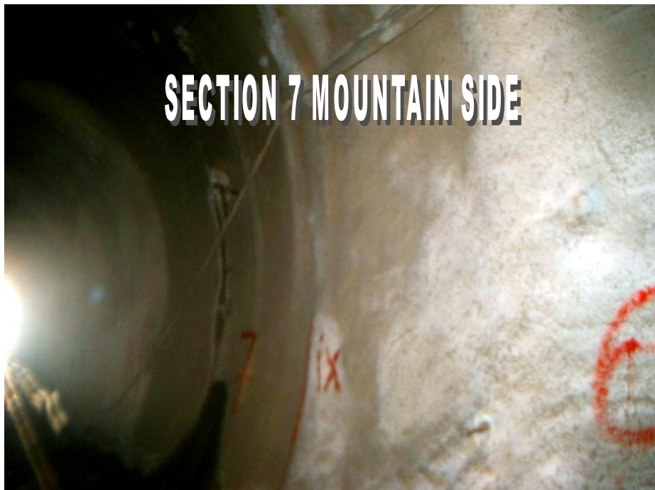
Figure 4.28 The Condition of Section 7 after the Rehabilitation of the Tunnel
