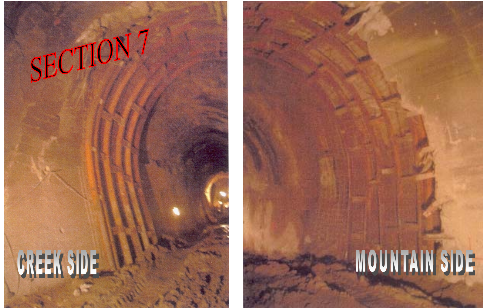
Figure 4.27 The Condition of Section 7 before the Rehabilitation of the Tunnel
