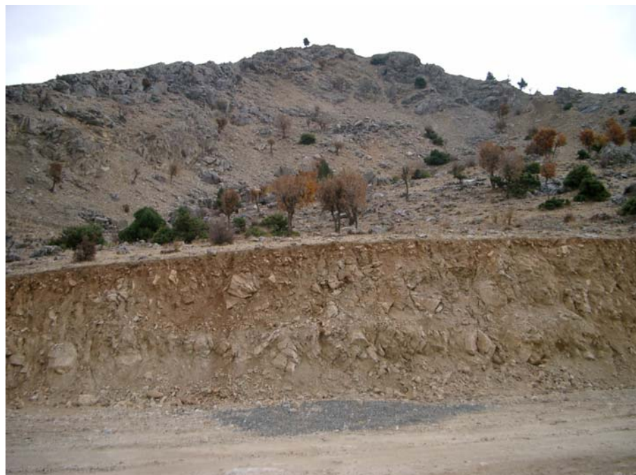
Figure 3.8 Landslide Materials at the Mountain Side (after Ergun et al., 2002)
