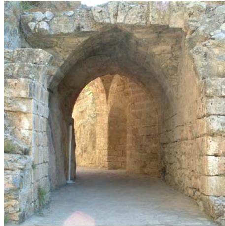
Fig.108: The Vaulted Path Inside The Gate Is Slightly Bending.
