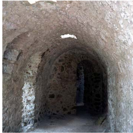
Fig. 190: Inside The Tower, There Are Openings On The Roof For Light And On The Walls For Ventilation And Shooting.
