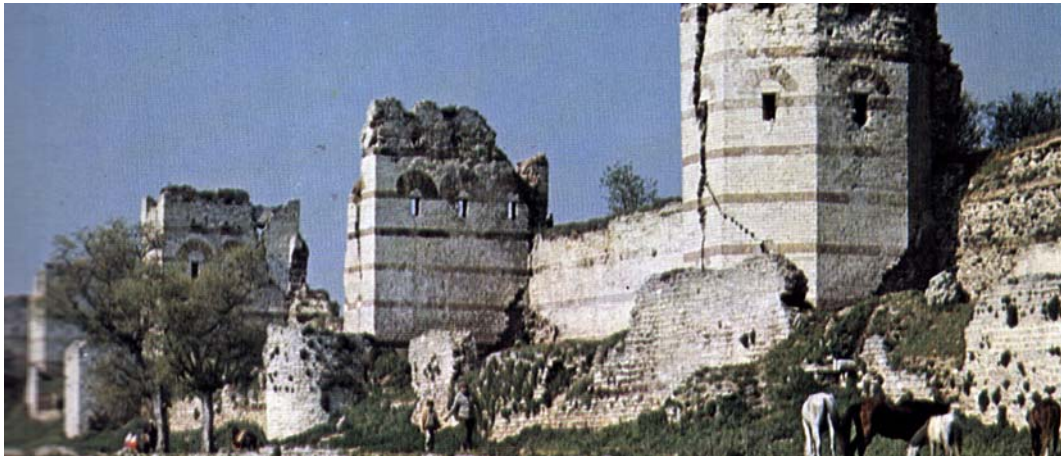
Figure 33: Constantinople, The Walls.
