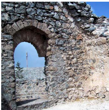
Fig. 165: From The Window Of The Room, The Cellular Rooms May Be Observed.
