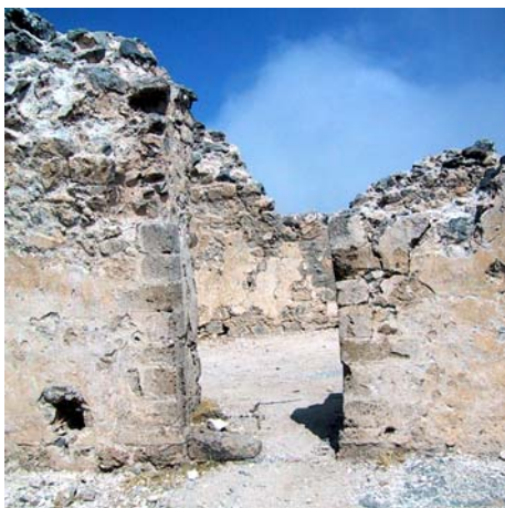
Fig. 164: The Two Rooms Are Separated With A Door, There Are Plaster Remains On The Walls.
