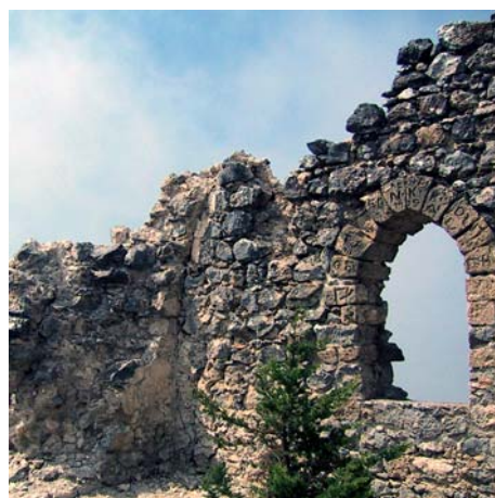
Fig. 163: The Window Of The Adjacent Room.
