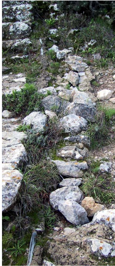
Fig. 201: The Detail From The Drainage Channels.
