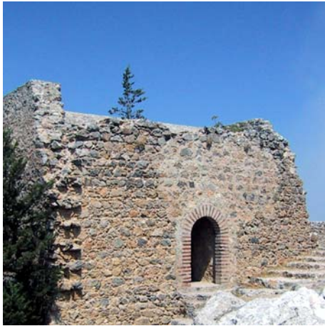
Fig. 152: The Vaulted Cell Structures Of The Upper Level.
