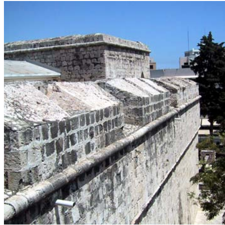
Fig. 70: The Places Of Blasting At The Roof.
