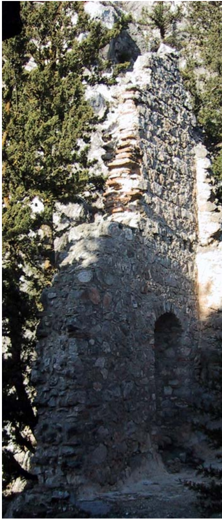
Fig. 147, 148: Interior Views With Traces A Second Storey.
