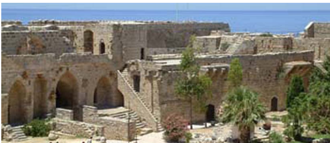
Figure 63: View Of The Buildings Around Courtyard.
