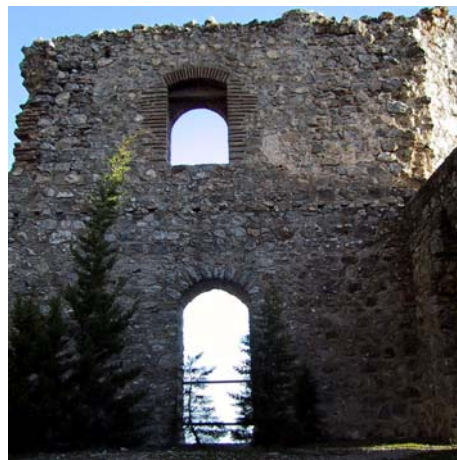
Fig. 151: The Windows Of The Bigger Chamber.
