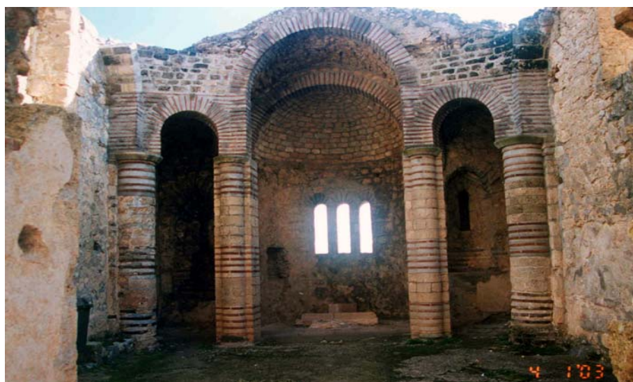
Figure 115: The Church With The Double Layers Of Brick Which Is Peculiar To Byzantine Architecture.
