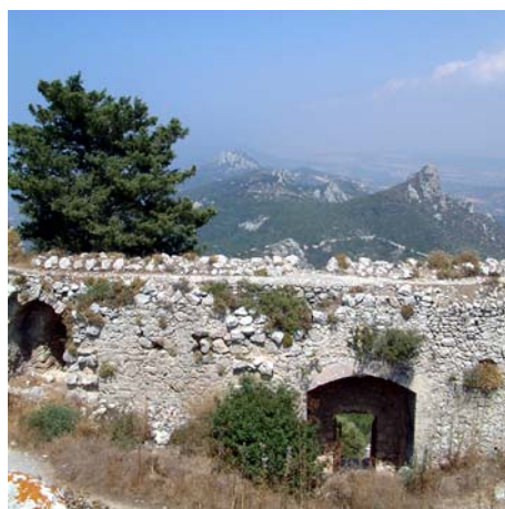
Fig. 186: The Second Gate From Inside.
