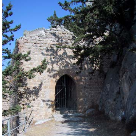
Fig. 137: The Gate Structure From Outside.
