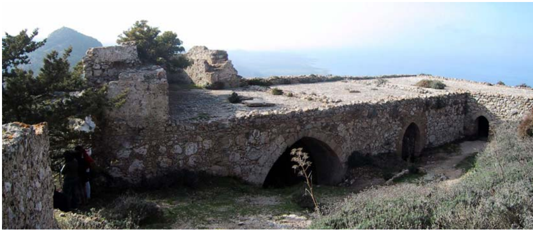
Figure 197: The Chambers In The East With A Horse Shoe Shaped Tower.
