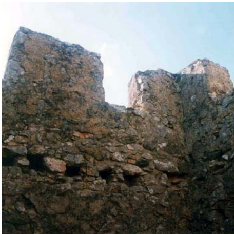
Fig. 128: The Crenellated Roof And The Traces Of Wooden Fighting Platform.
