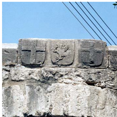
Fig. 52: The Relief On The Aqueduct.
