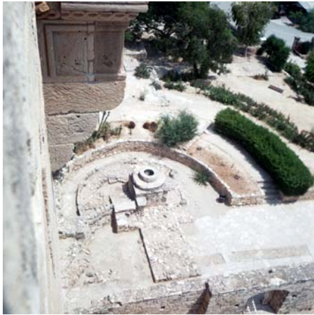
Fig.48: The Well Is Seen From The Roof. The Brackets Of Machicolations Are On The Top Left.
