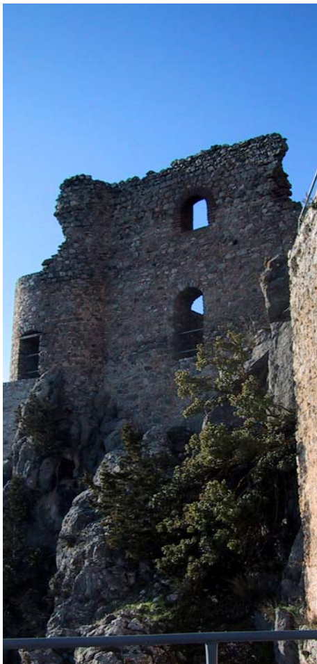
Fig. 144: The Main Building From The Terrace In Front Of It.
