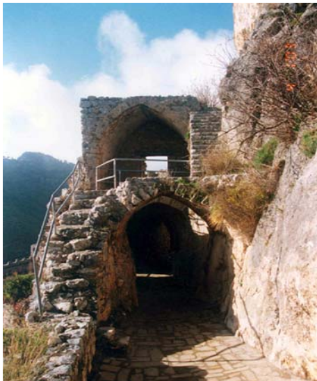
Fig. 109: Gate From Inside.
