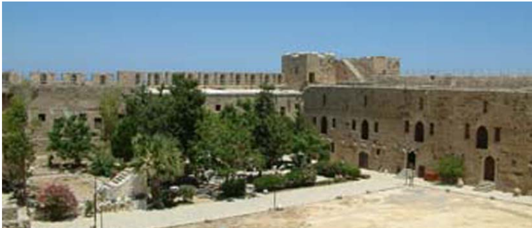
Figure 64: View Of The Buildings Around Courtyard.
