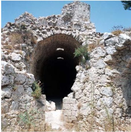
Fig. 189: The Vaulted Entrance To The Tower.
