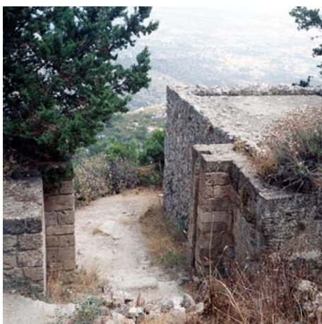
Fig. 177: The Gate Structure That Enters The Barbican.
