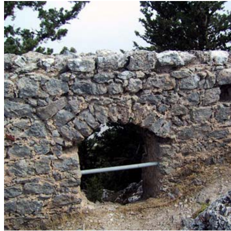
Fig. 159: Opening On The Enclosure Wall.
