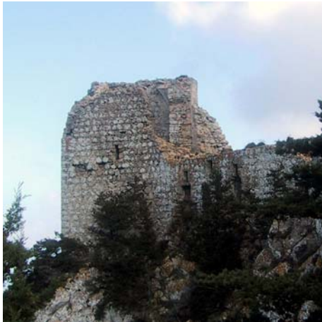
Fig. 191: The Square Tower Protecting The Barbican.
