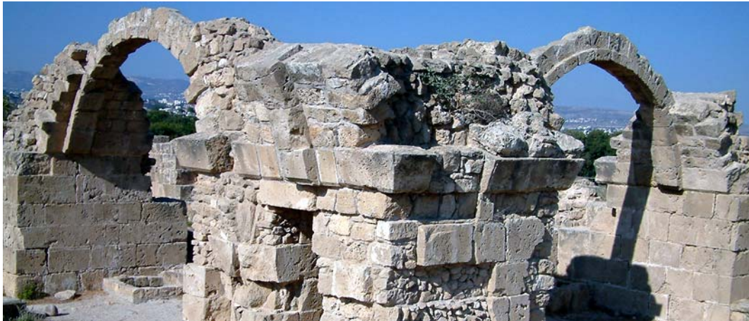
Figure 78: Remains Of The Vaults From Saranda Colones.
