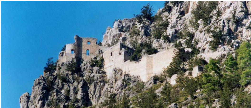
Figure 134: The Walls Of The Castle Emerges As A Part Of The Rocky Cliff. Due To The Natural Strength Of The Site, The Castle Does Not Have An Enclosure Wall.
