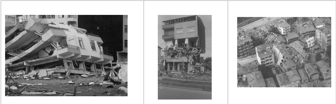
Figure 5.3. Physical Damages in Building Fabric
