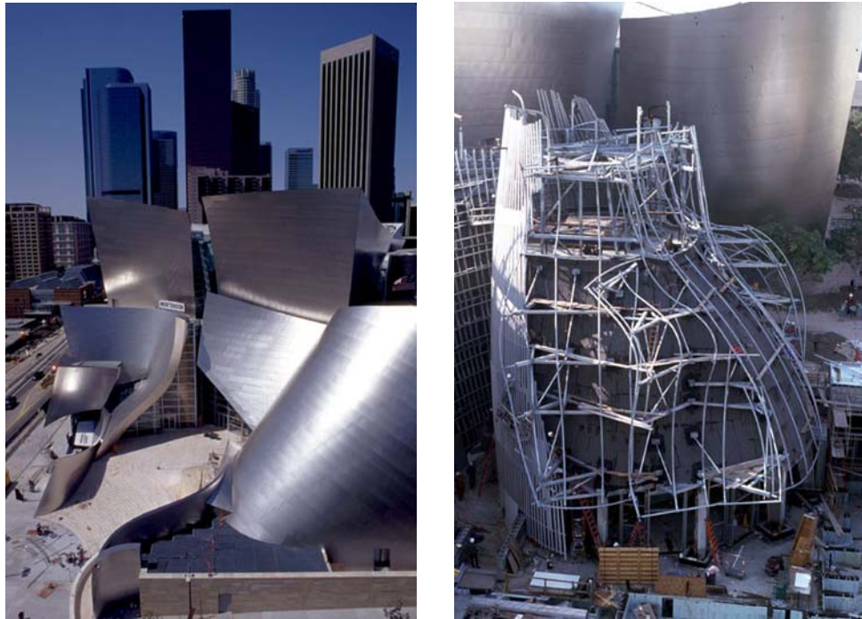
Figure 6.17. Walt Disney Concert Hall, above left entrance, right construction, west side, Los Angeles, California, 2003.
