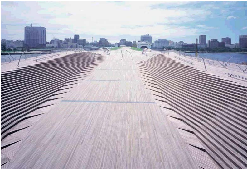
Figure 6.11. Yokohama International Port Terminal, above top and bottom roof terrace park setting, 1995-2002.
