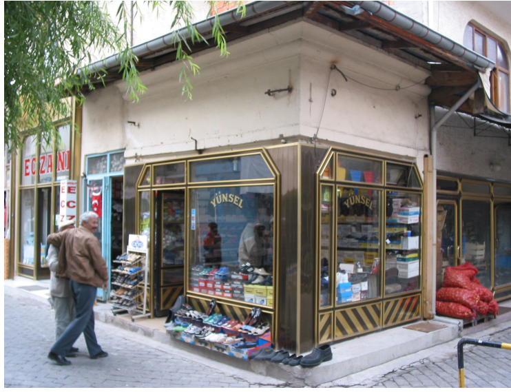
Figure 29 Inappropriate fenestrations covering façades of shops
