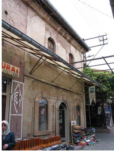
Figure 27 Additional eaves permanently fixed on façades
