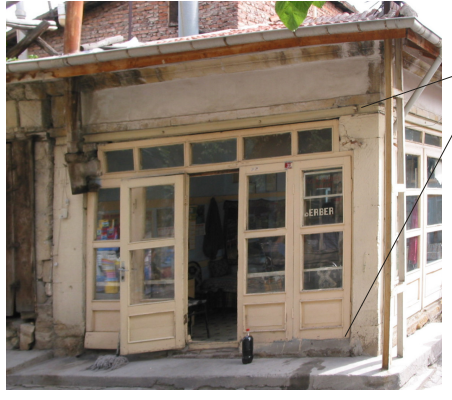
PHT 3.1: Shop with shutters removed
