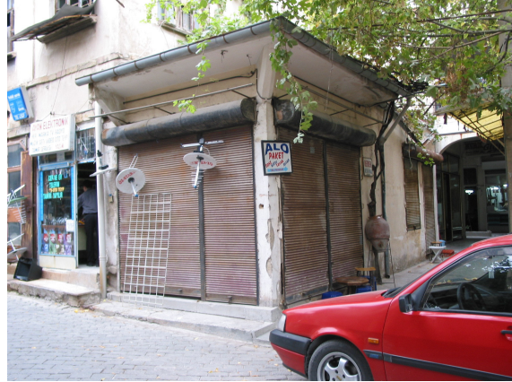
Figure 26 Additional metal rolling shutters
