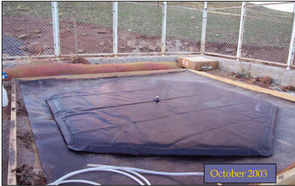
Figure 3.5 Snow pillow installation (Cat)
