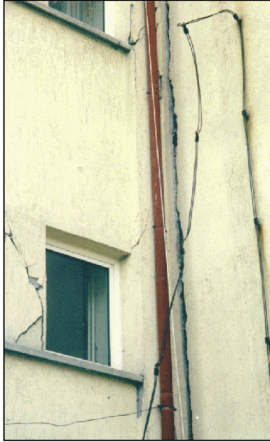
Figure 6.30 D9 columns at the first and second stories
