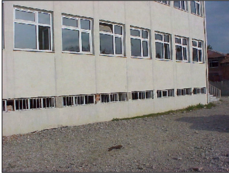
Figure 6.53 Rear elevation of the building after Düzce earthquake of 12 November 1999
