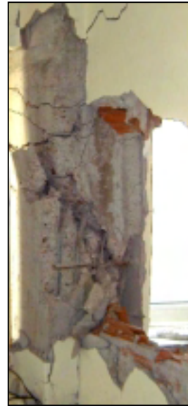
Figure 6.27 Severely damaged column D10 at the first story
