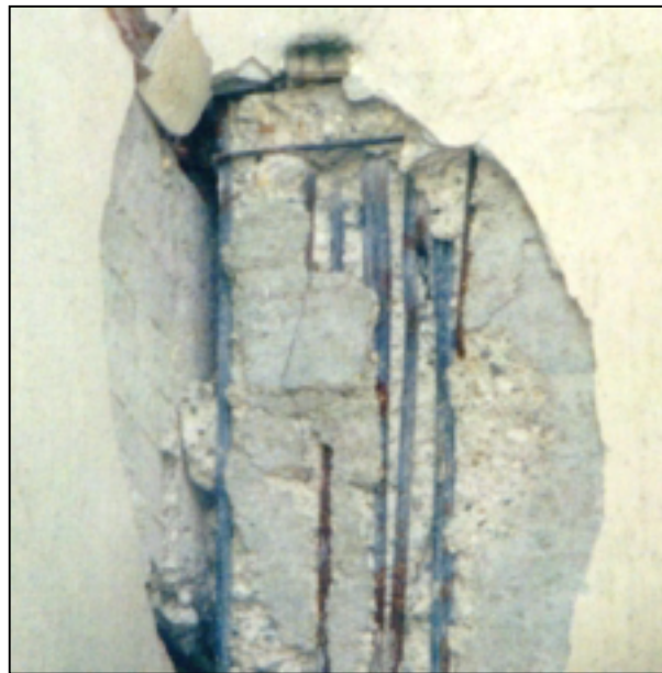
Figure 6.13 Column D12 at the ground story
