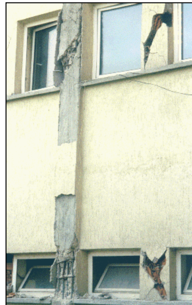
Figure 6.11 Failed D10 columns at the ground and first stories
