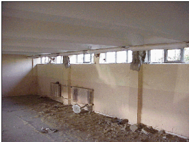
Figure 6.54 Columns F3 and F5 at the ground story
