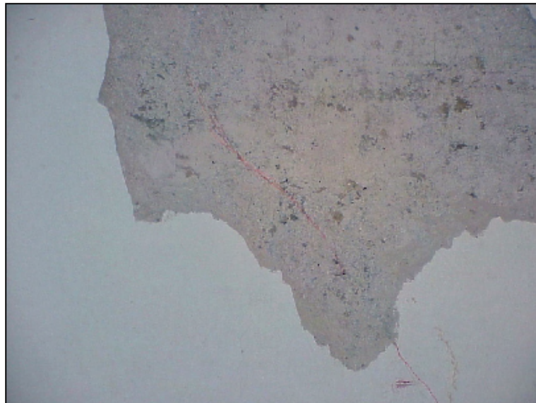
Figure 6.58 Diagonal cracks on the web portion of the shear wall P1 at the ground story
