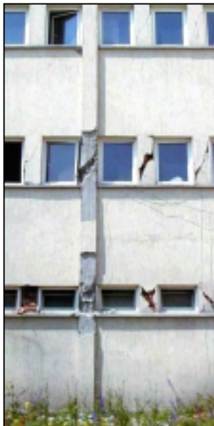
Figure 6.11 Failed D10 columns at the ground and first stories
