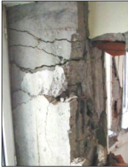
Figure 6.27 Severely damaged column D10 at the first story
