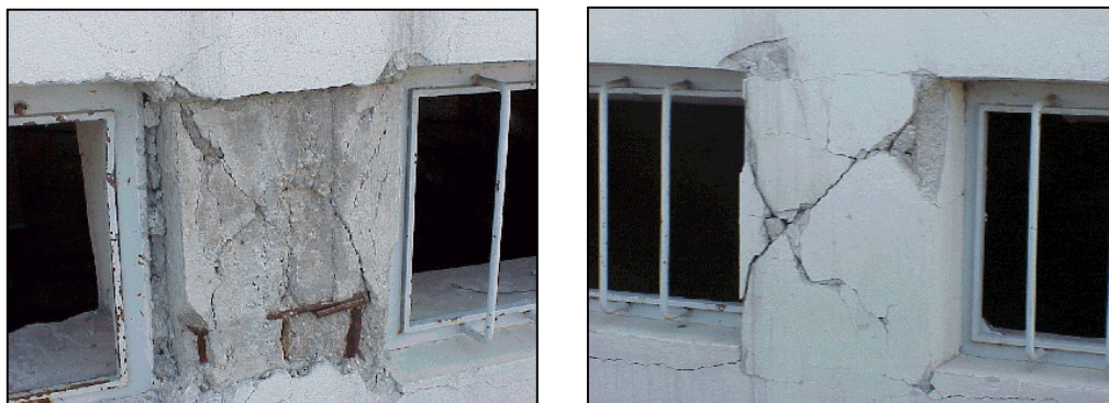
Figure 6.55 Columns F8 and F10 at the ground story
