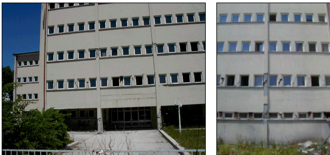
Figure 6.8 Front and rear elevations of the building after Düzce earthquake
