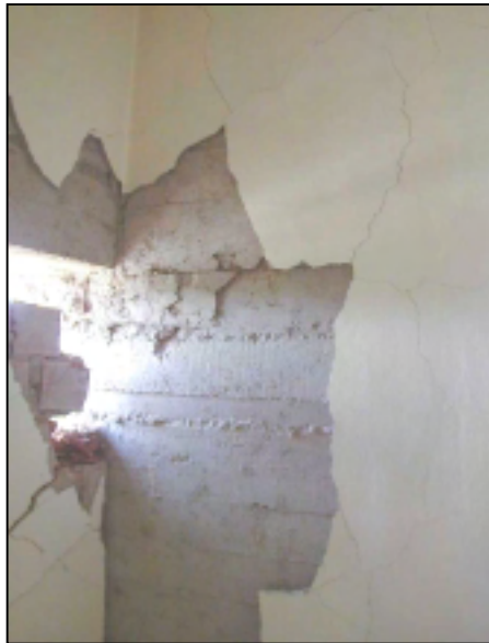
Figure 6.28 Column G12 at the first story
