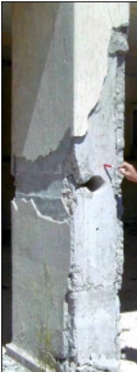
Figure 6.25 Column G10 at the ground story
