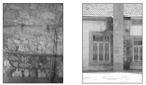
Figure 2.28 Weatherings on masonry elements Figure 2.29 Weatherings on east façade
