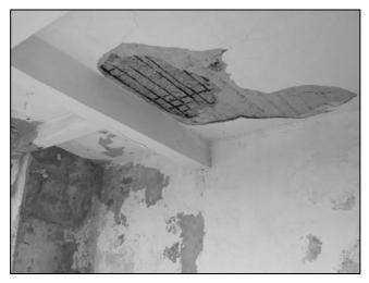
Figure 2.31 Weatherings in reinforced concrete slab
