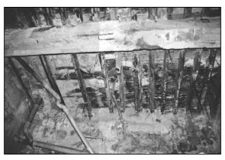
Figure 2.30 Weatherings in timber flooring
