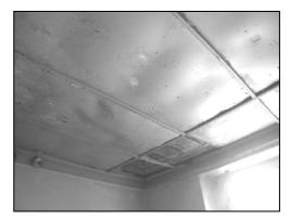
Figure 2.37 Plywood ceilings in space 101
