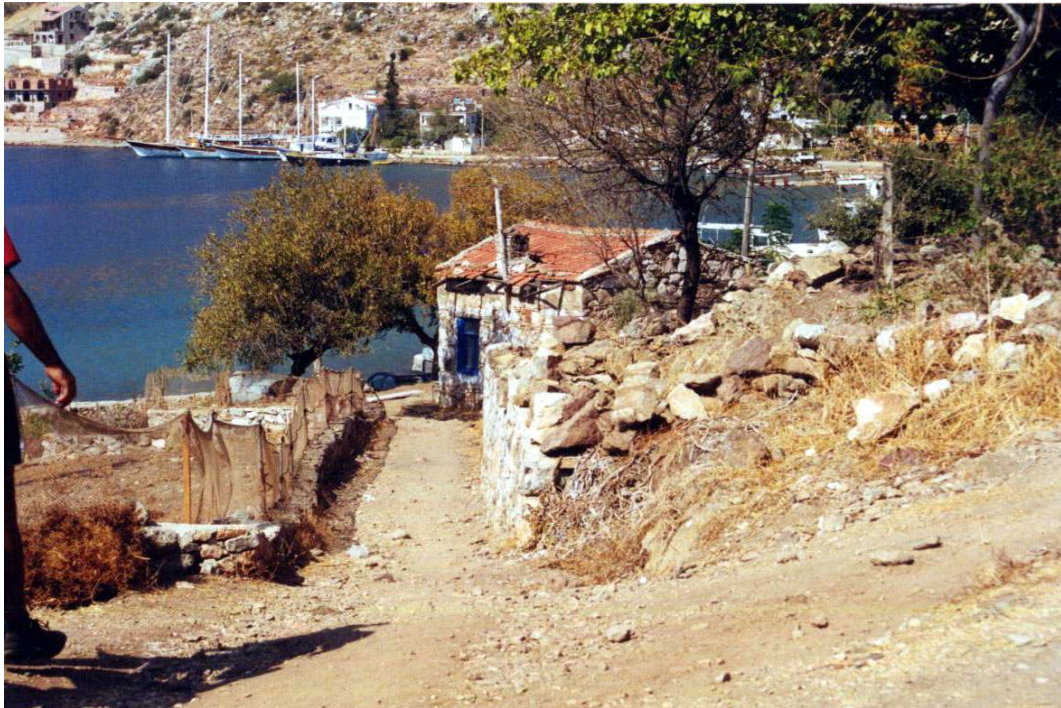
Figure 40. An example of wall and street pattern, which are the local values of Bozburun and have to be knocked down when the Coastal law is enforced. Establishment of wall, fence and railing within the shore strip is prohibited (UD Studio Archive).
