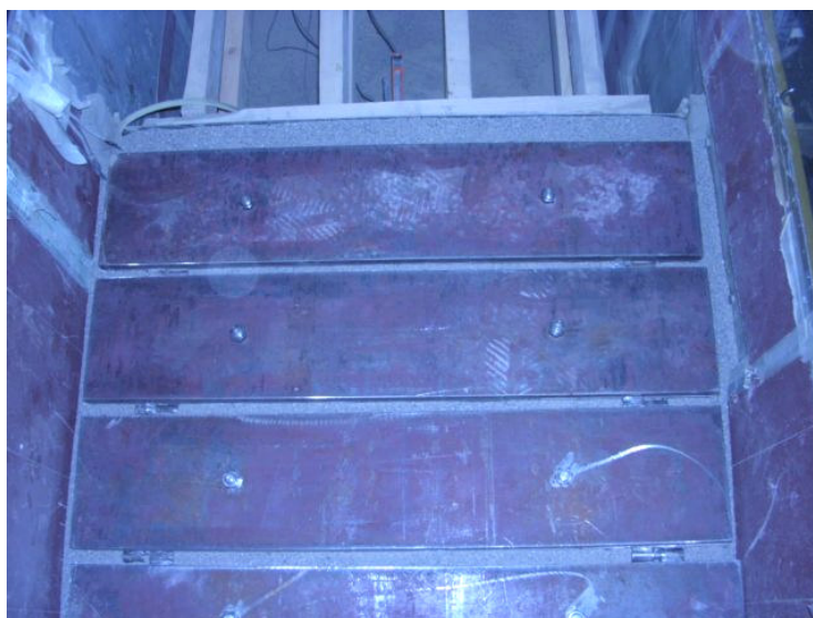
Figure 3.8 Surcharge blocks on top of the backfill
