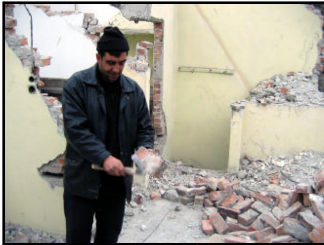
Figure 4.28 Cleaning of bricks with an adze
