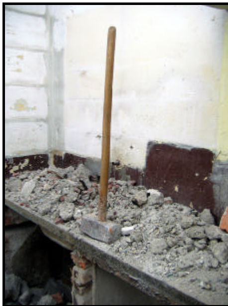
Figure 4.6 Sledgehammer used for breaking masonry and reinforced concrete components
