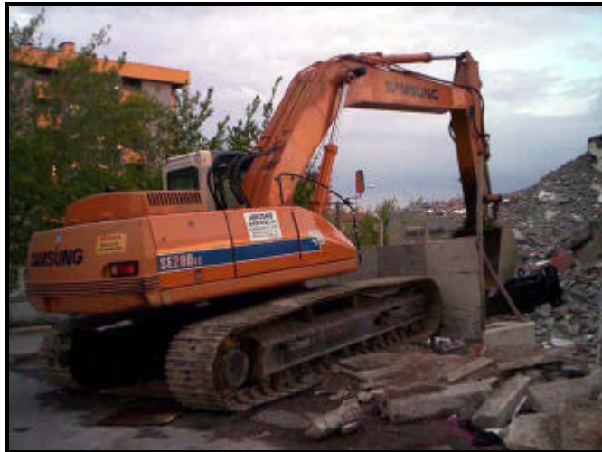
Figure 4.2 Excavator used for digging
