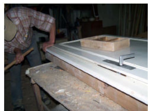
Figures 5.21-22-23-24 A door recovered from a demolished building being repaired in a warehouse on Bentderesi Avenue
