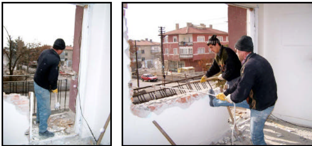
Figures 4.18-19 Dismantling the wrought iron balcony balustrade (building C)
