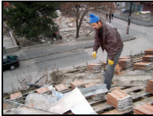
Figures 4.21-22 Recovery of the roofing tiles (building C)
