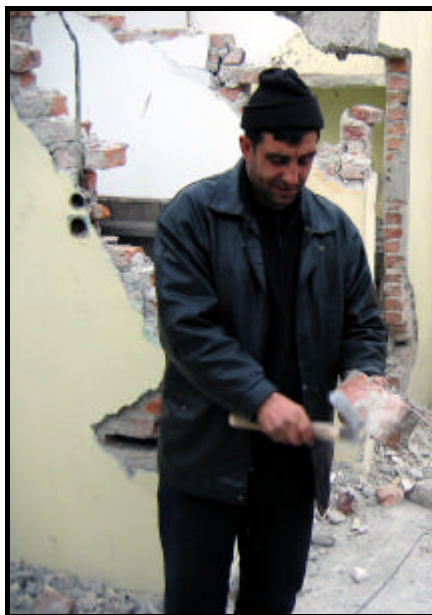
Figure 4.1 Adze used for cleaning bricks
