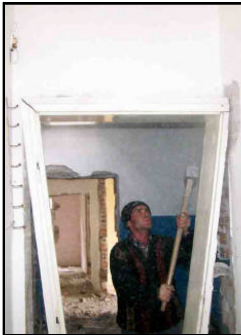
Figures 4.12-13 Removal of the door frame from building C
