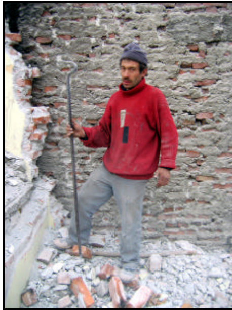
Figure 4.5 Manila , a long handed wrench, used in recovery of bricks
