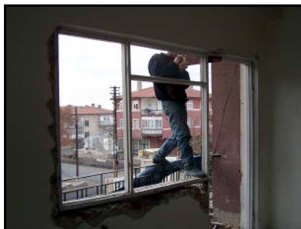
Figure 5.30 The windows and door produced as a unit (building C)
