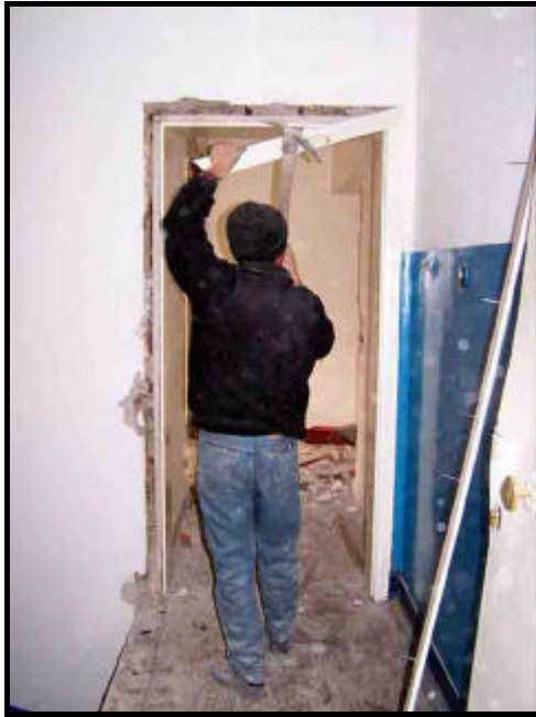
Figures 4.10-11 Taking out the door frame from building C
