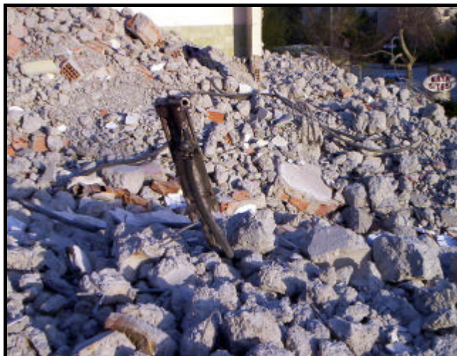
Figure 4.4 Pneumatic drill used for breaking reinforced concrete components
