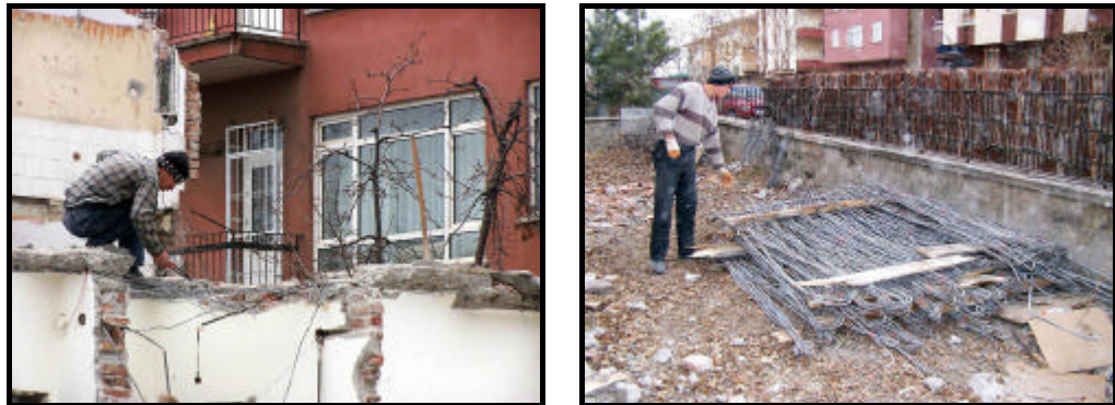
Figures 4.31-32 Recovery of rebar (building C)
