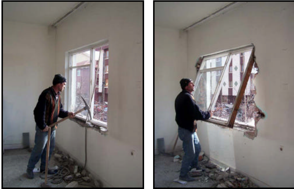
Figures 4.8-9 Disassembling the window (building C)
