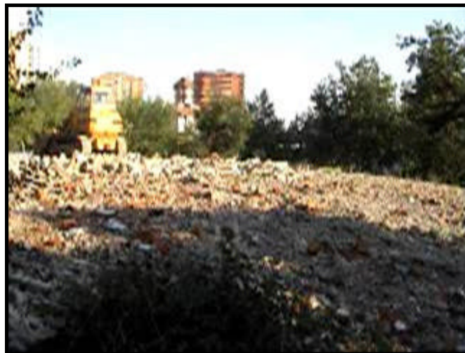
Figure 3.3 After demolition of building A in Oran
