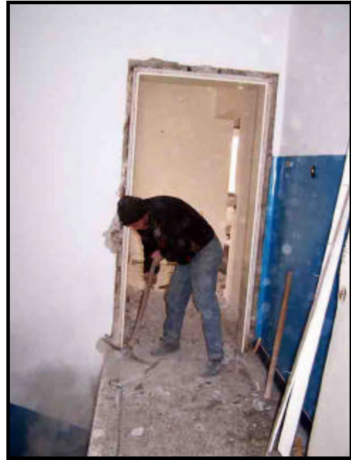
Figures 4.10-11 Taking out the door frame from building C
