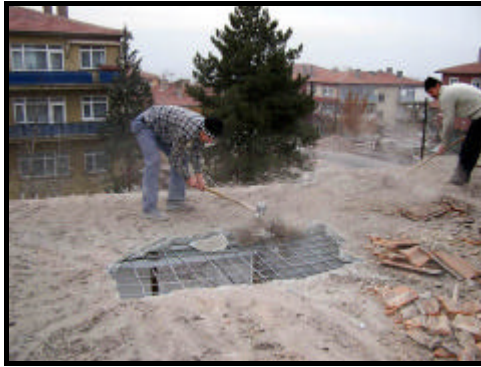
Figures 4.23-24 Demolition of the roof slab (building C)
