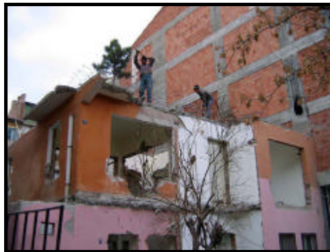
Figures 4.25-26 Demolition of the roof slab of a masonry building in Yenimahalle
