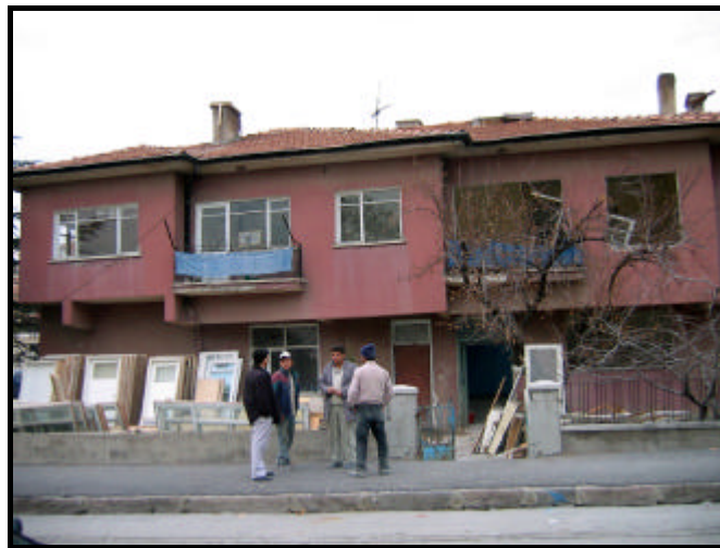
Figure 3.5 Before demolition of building C in Yenimahalle
