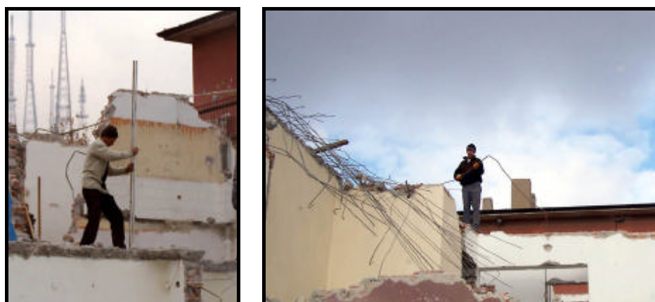
Figures 4.33-34 Recovery of pipes and electric cables (building C)
