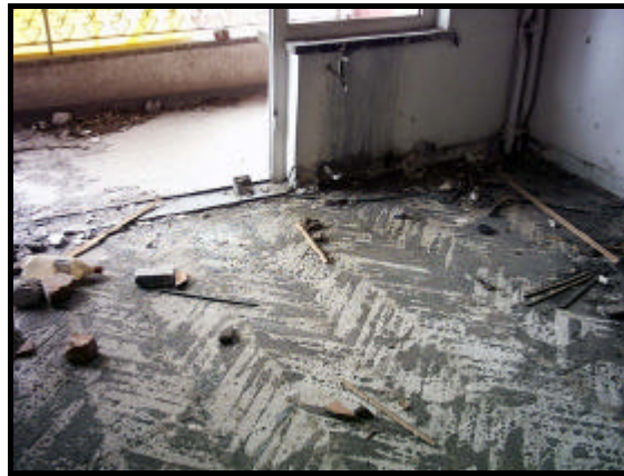
Figure 4.35 Glued parquet coverings were removed from building B
