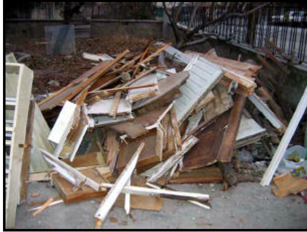
Figure 5.20 Timber components damaged during dismantling can be used as fuel to burn (building C)
