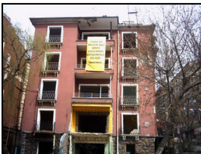
Figure 3.4 During the deconstruction of building B in Kavaklıdere
