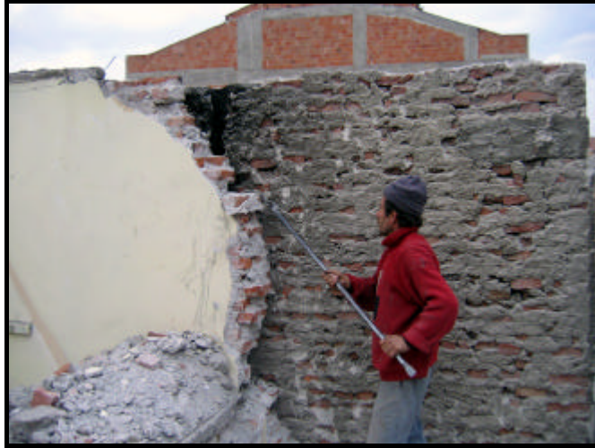
Figure 4.27 Removal of bricks from the structure with a manila
