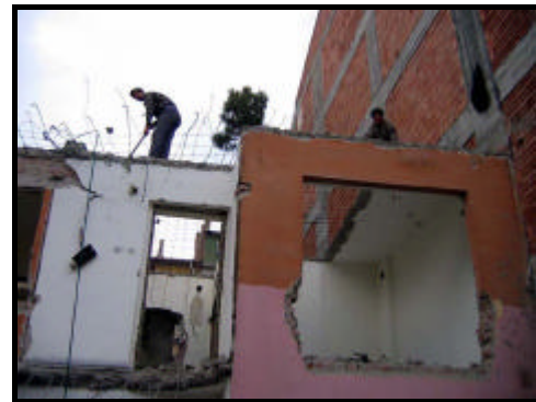
Figures 4.25-26 Demolition of the roof slab of a masonry building in Yenimahalle
