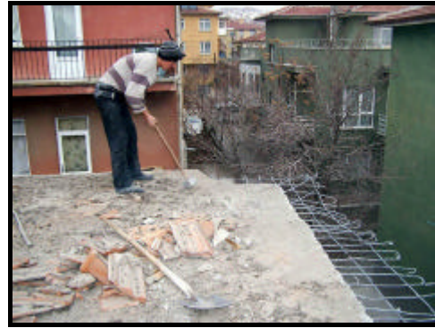
Figures 4.23-24 Demolition of the roof slab (building C)
