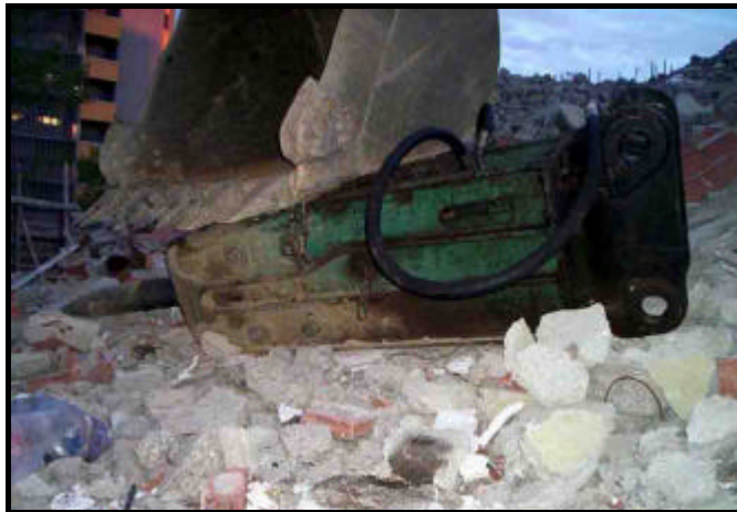
Figure 4.3 Breaker attachments used for breaking reinforced concrete components
