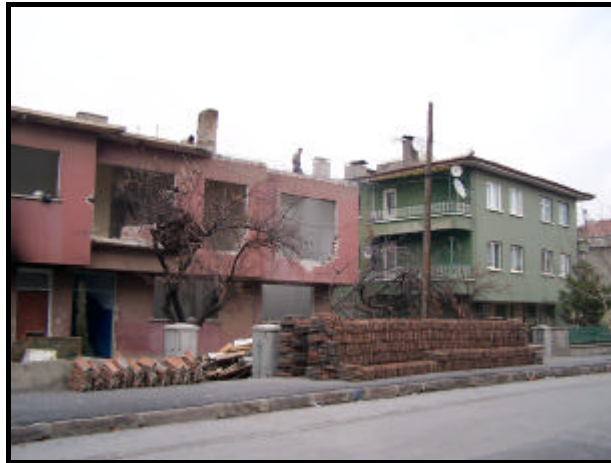
Figure 5.14 Roofing tiles of building C
