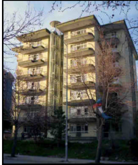
Figure 3.2 Before demolition of building A in Oran
