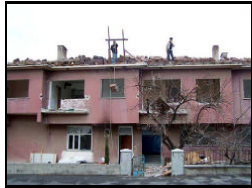
Figures 4.21-22 Recovery of the roofing tiles (building C)
