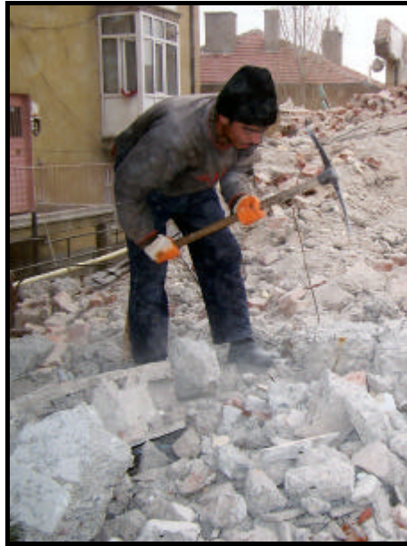
Figure 4.7 Pickaxe used for breaking masonry and reinforced concrete components as well as in recovery works
