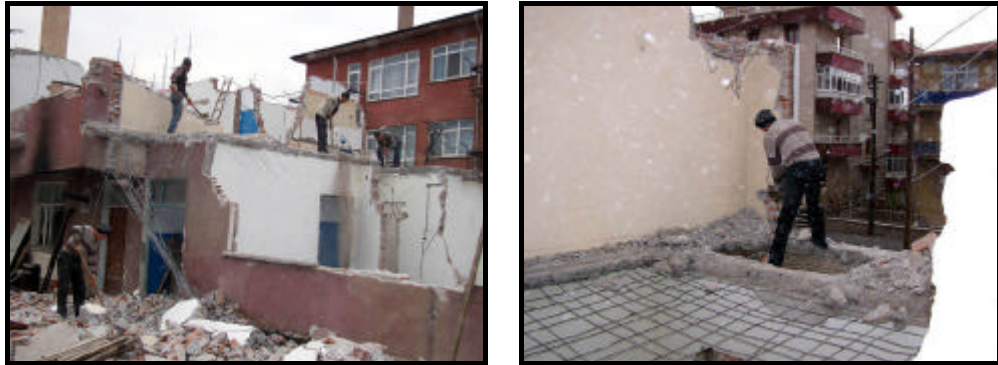
Figures 4.29-30 Demolition of floor slab (building C)
